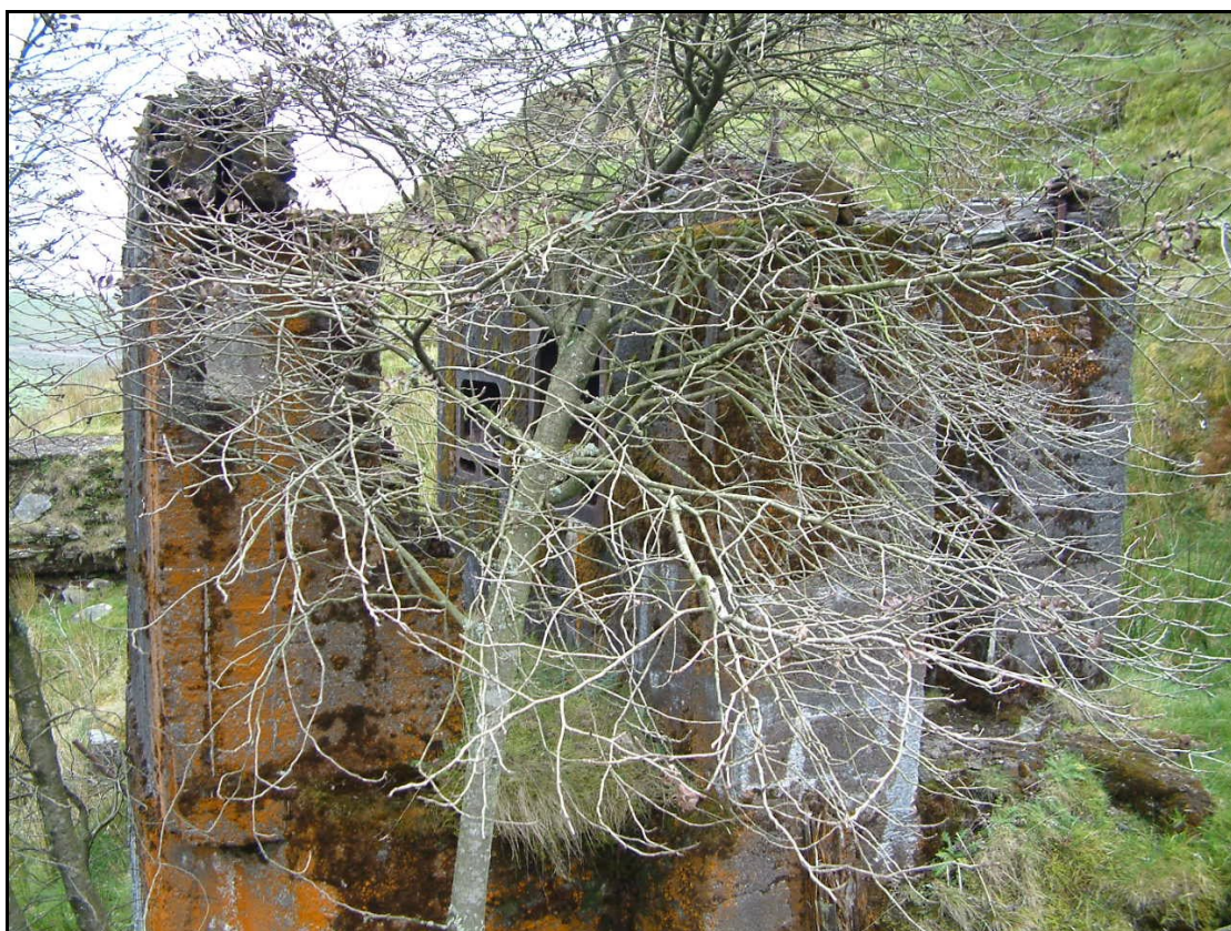
Nantiago Mine, winding house (NGR SN82488639) © CPAT Image 1519-0051
