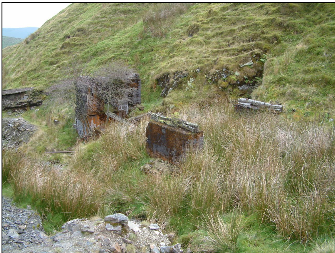
Nantiago Mine, winding house (NGR SN82488639) © CPAT Image 1519-0046
