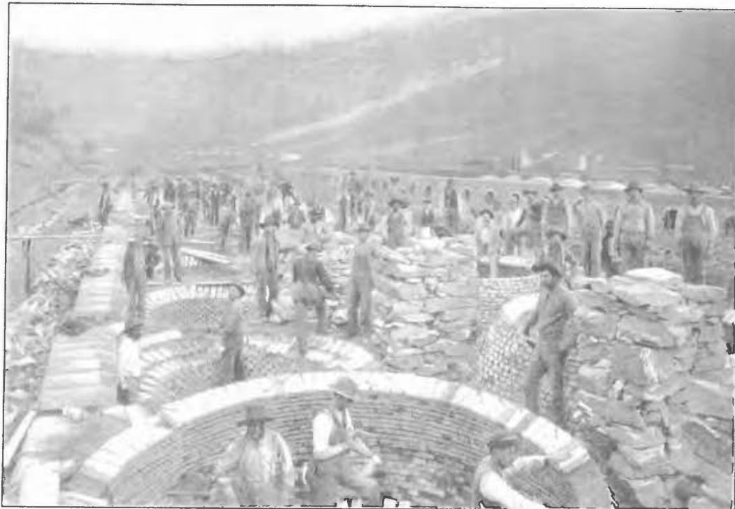
FIG. 9. CONSTRUCTION OF BEEHIVE OVENS
