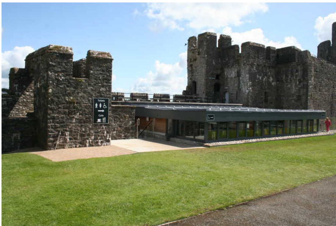
Photo 15: A view of the new café after completion, looking southeast.
