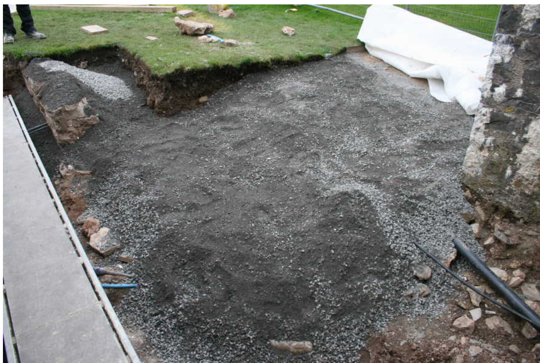
Photo 14: The graded limestone (8mm to dust) laid over the revealed archaeological features prior to being covered by a geotextile membrane (top right).
