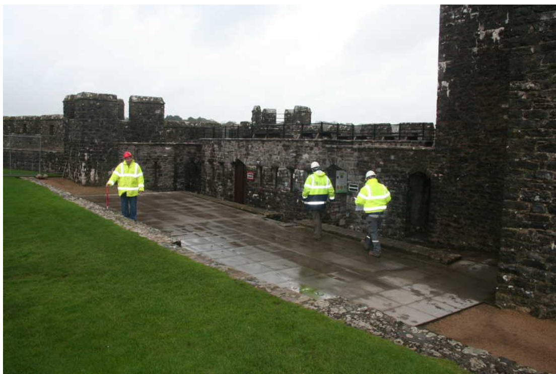
Photo 2: Oblique view of the two retaining walls and flagstone area in front of St. Anne's Bastion prior to groundworks. View north.
