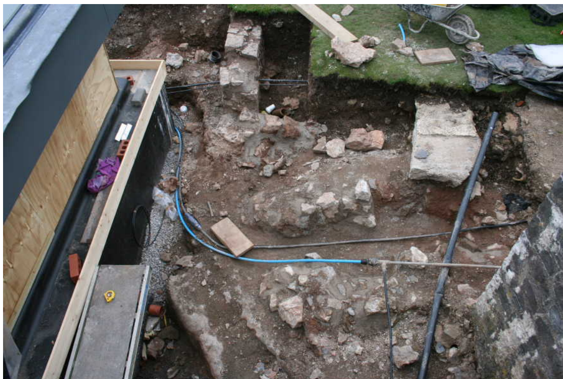
Photo 13: Revealed structures as they looked after consolidation, immediately prior to their reburial in February 2009.
