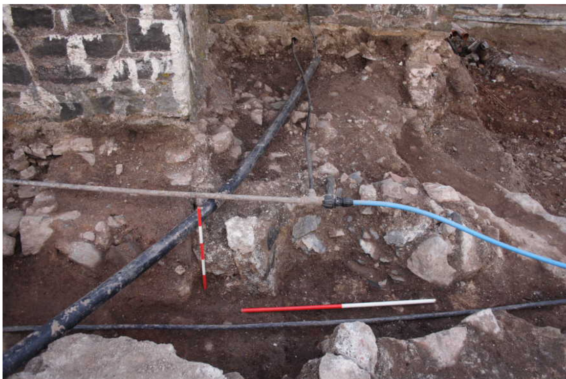
Photo 10: View northeast across structure 132, with wall 131 to the left, layer 133 in the upper part of the photo and truncation from modern services, scales 1m and 0.5m. Wall 104 lies in the upper right part of the photograph.
