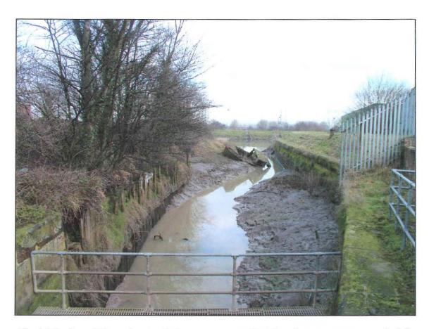
Fig. 16 Sandycroft Quay showing timber revetment on the left and stone revetment on the left.
