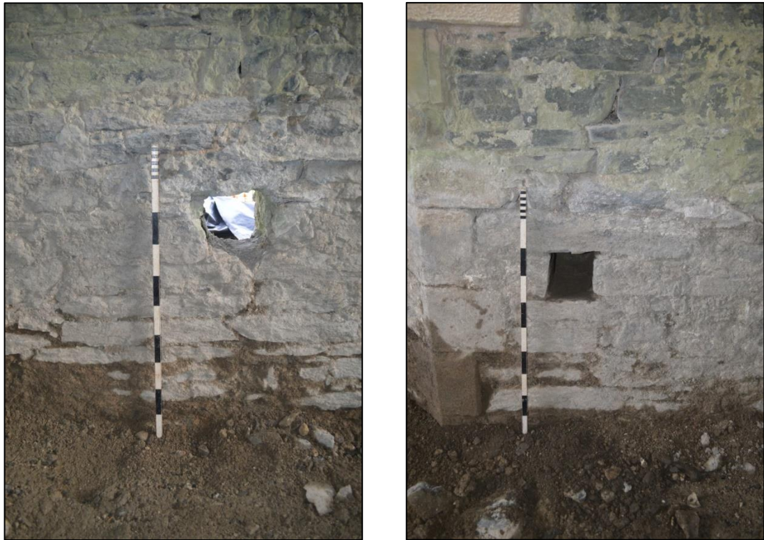
Fig. 21 Draw-bar holes for bracing the gatehouse door, north wall and south wall, south turret. Photo CPAT 4946-0199, 4946-0188
