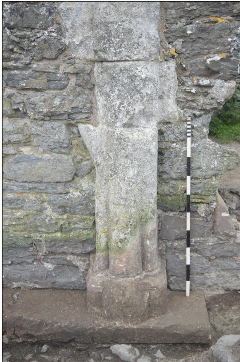
Fig. 13 South turret wall. Base of dressed colonette/pillar (017), viewed from the north. Photo CPAT 4946-0100
