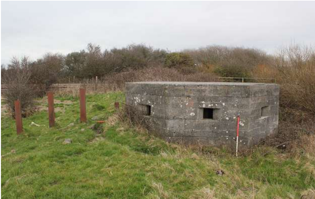
Figure 67: Pillbox with anti tank rails to the side
