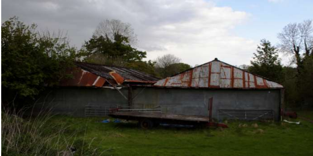
Figure 143: Only the concrete plinth from the beacon survives with a shed built over it
