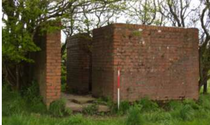
Figure 140: Brick transformer plinth
