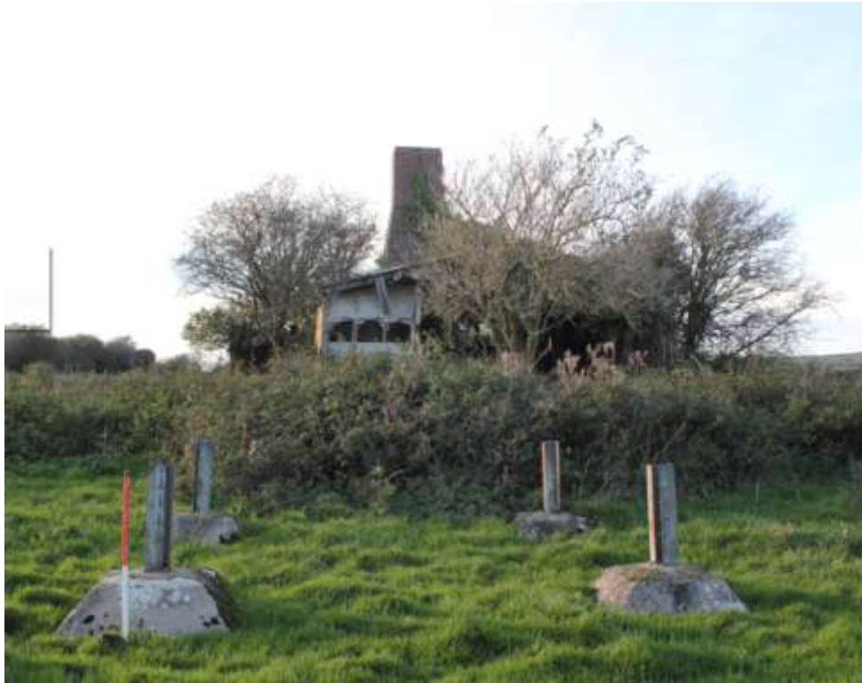
Figure 74: Radio station at RAF Pembrey, mast fixings in the foreground
