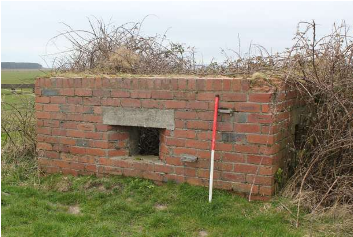
Figure 65: Pillbox on the sea wall at Pembrey, note metal access treads in brickwork
