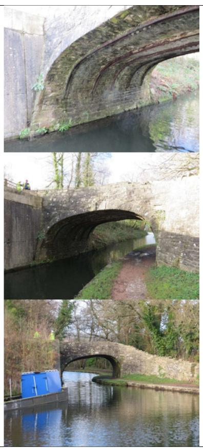
Condition: Repair required to parapets. There has been a substantial collapse on the south side.
