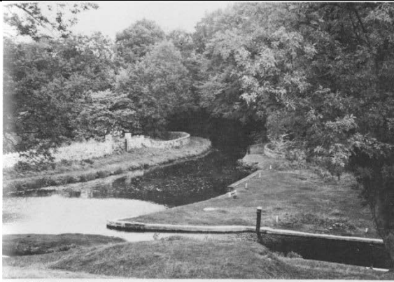
Plate 25 The dry dock at Govilon with the river aqueduct in the background. There are stop plank grooves in the left foreground and a drain paddle for the dock in the right foreground. The water drains through a culvert to the river near the aqueduct. Note the windlass to the left of the paddle for lifting a drain plug from the bed of the canal.
