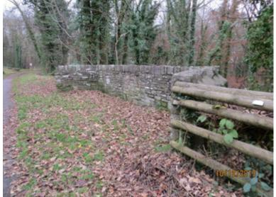
Condition: Towpath parapet cracked vertically at centre with coping missing.
