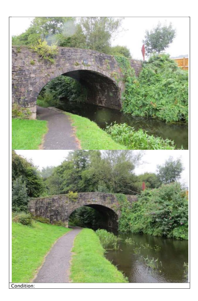
Good but detailed survey of masonry desirable. Poor ribbon pointing.
