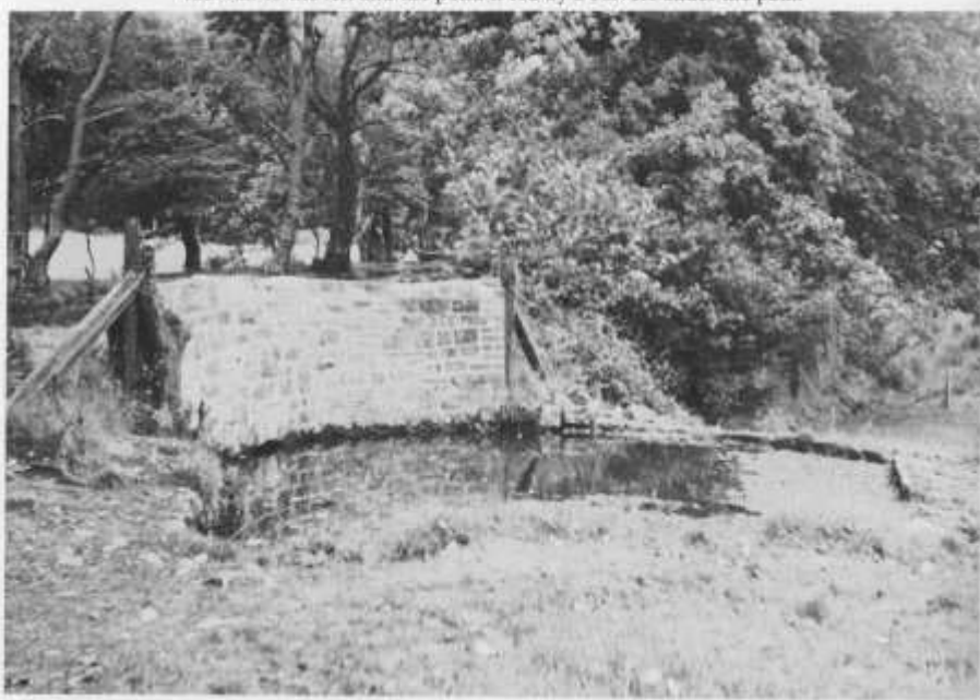
Plate 32 Overflow weir forming a cattle pond north of bridge 77. The canal and towing path are over the wall to the left and the pond is fed by a culvert under the path.
