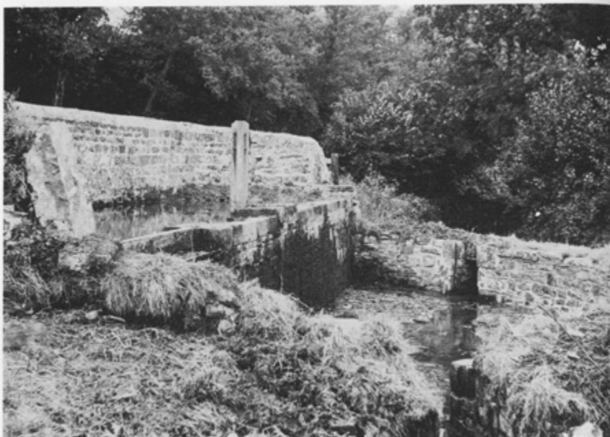
Plate 31 Overflow weir and drain sluice north of bridge 82. The towing path is beyond the wall and the water in the upper pond is at canal level. It is connected to the canal by a culvert under the path. Water passing over the weir or through the drain sluice leaves the lower pond via culverts in the background and foreground.
