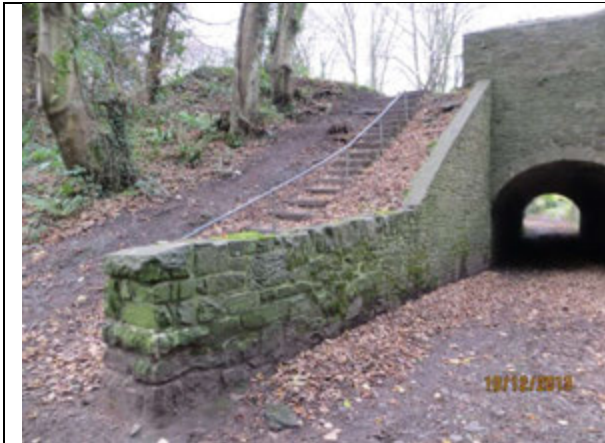
Wing wall and stair towpath side
