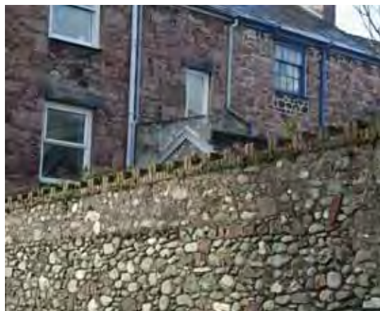
Random rubble to the rear of Segontium Terrace, and river stones in the boundary wall.
