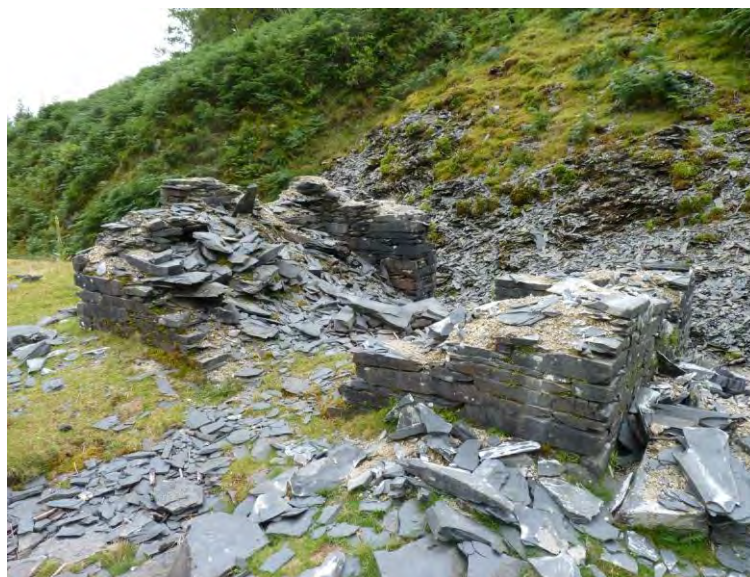
Fig 20 Weighhouse. The machine pit is under slate waste in the bottom left of the picture
