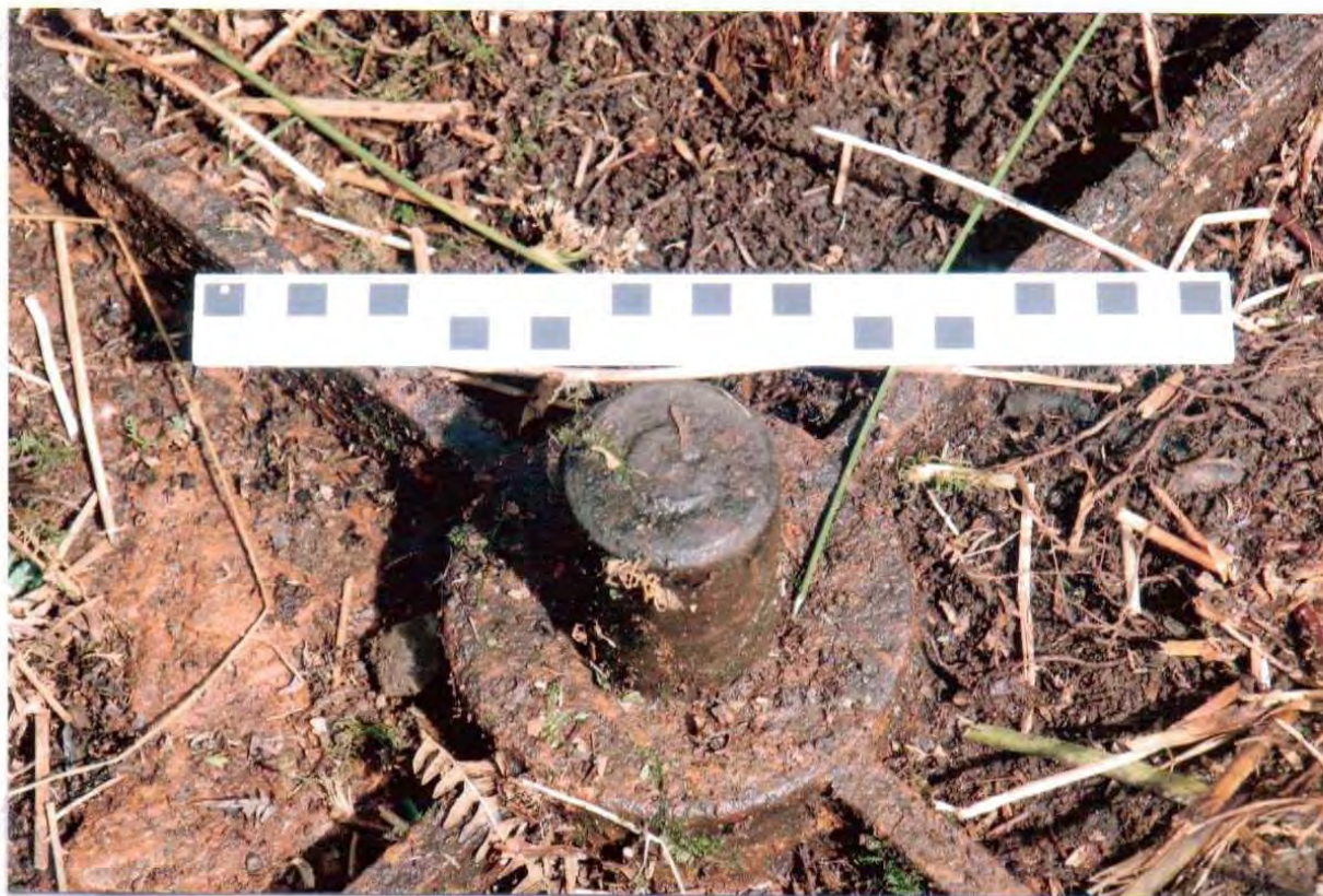
Photo 14. The centre pivot of the turntable base.
