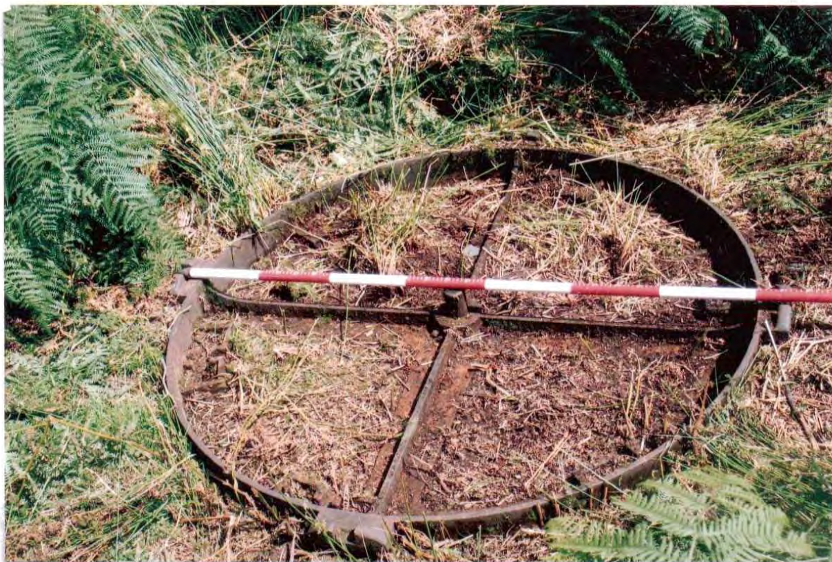
Photo 13. The turntable base, in the upper level of Cae Abatty Quarry. It is to the North of the drumhouse, in line with a cutting leading into the Twll.
