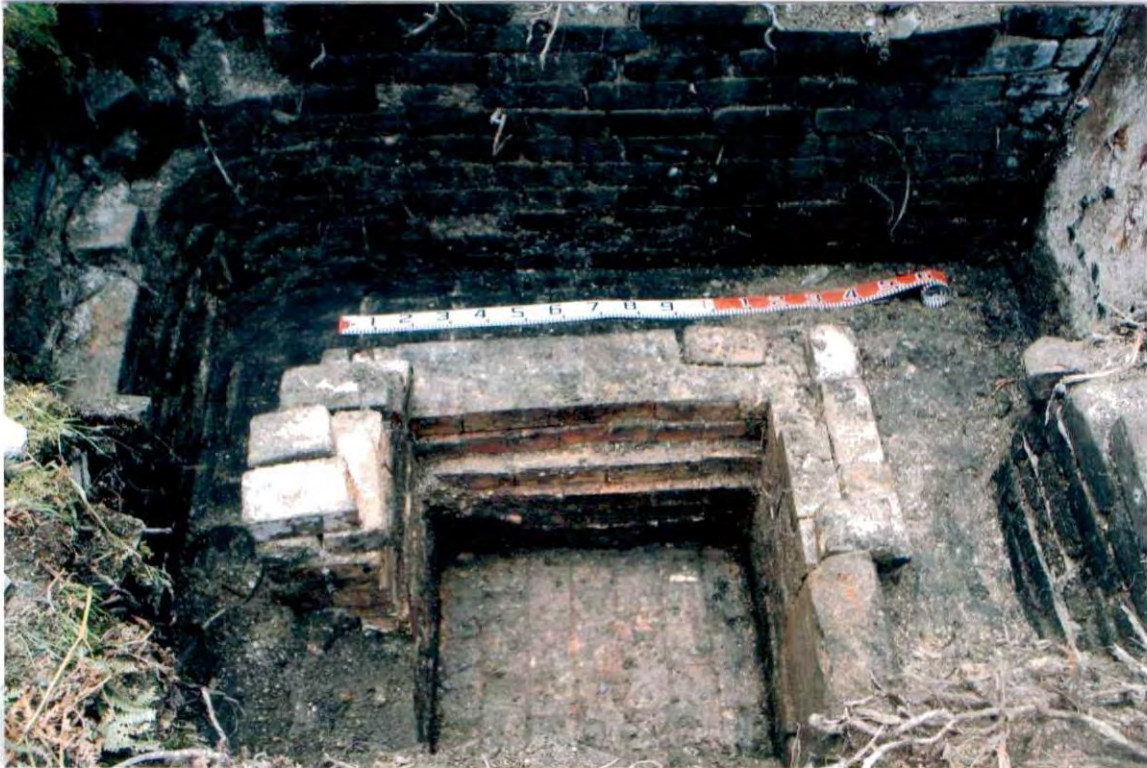
Photo 1. The excavated West end of the boiler flues. The damper to the chimney flue is on the right.
