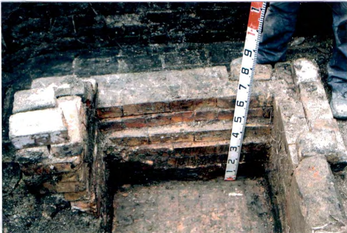
Photo 2. The West end of inner flue, at a lower level than the outer flue. Combustion gases from the boiler would have entered the flues at this point. An angled boiler support brick can be seen on the right.
