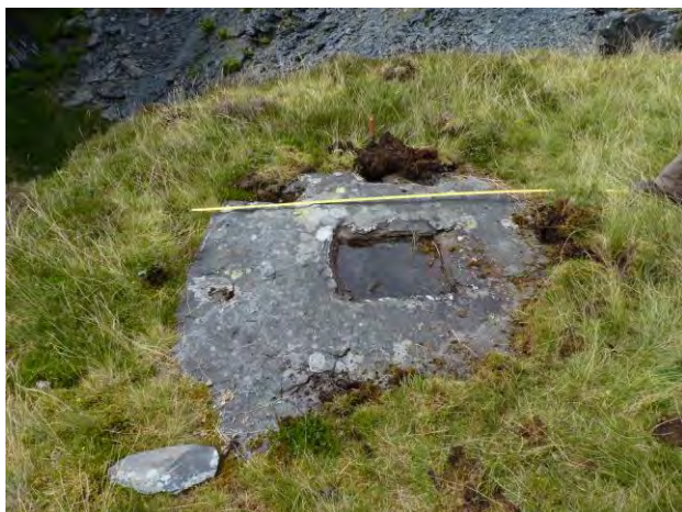
Concrete crane base
