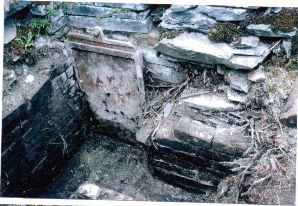
Photo 5. The North West corner of the outer flue, showing the chimney damper and the curved brickwork leading to it.
