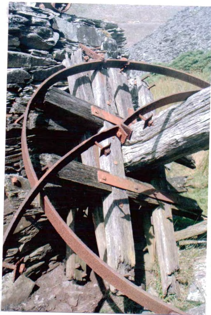
Photo 9. East spider of the Cae Abatty Incline Drum. The two cross members are half jointed and strapped across the open sides of the joint. The brake band and the braking surface rim encircle the spider.
