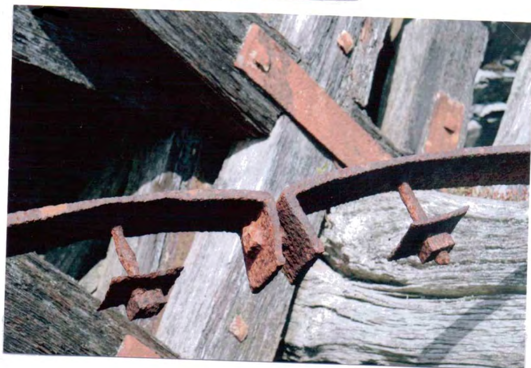
Photo 10. Detail of the braking surface rim of the drum, showing one of the four joints and two of the bolts which fixed it to the surface timbers of the drum.
