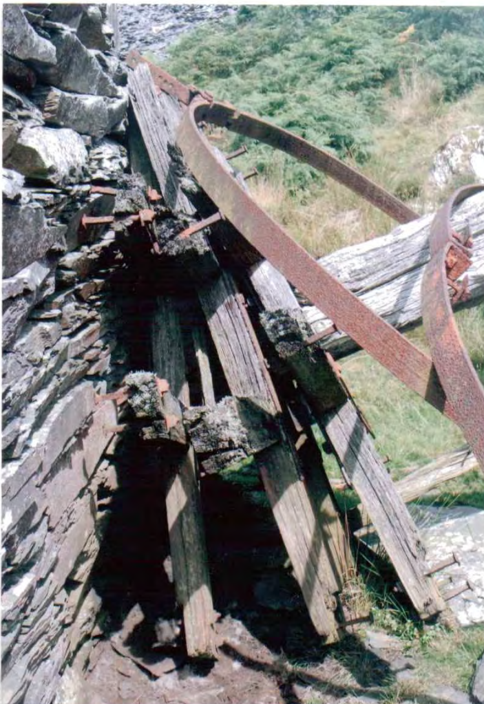
Photo 8. The cross members of the three spiders of the Cae Abatty Quarry Incline Drum. The rim timbers have totally disappeared, but their size can be derived from the bolts in the ends of the cross members.
