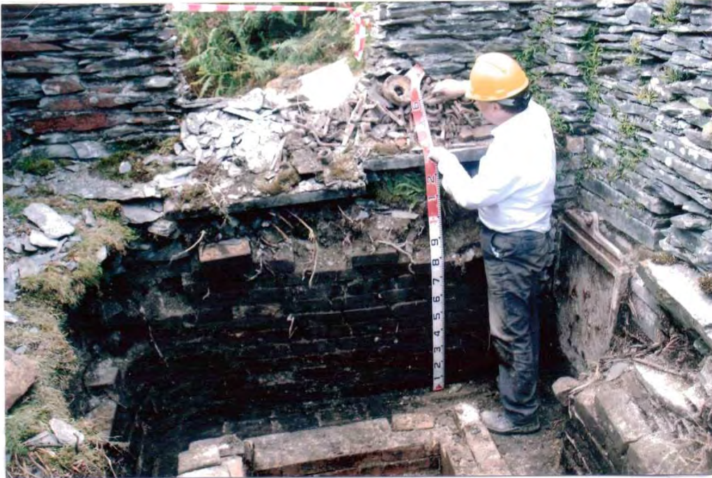
Photo 3. David Gwyn measuring the depth of the outer flue.
