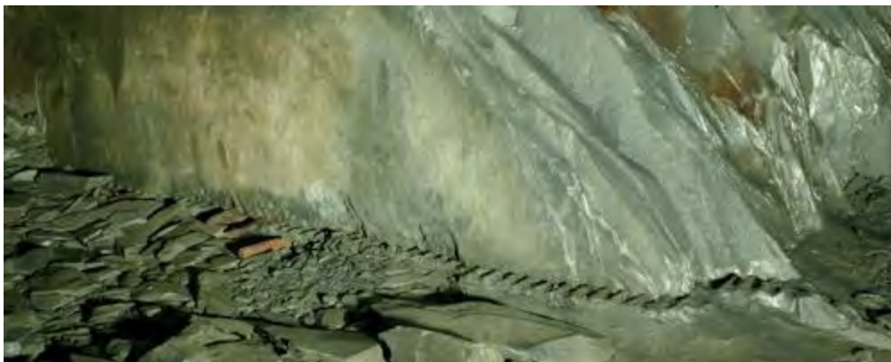
Channelling Holes at the base of the working face in Chamber 1
