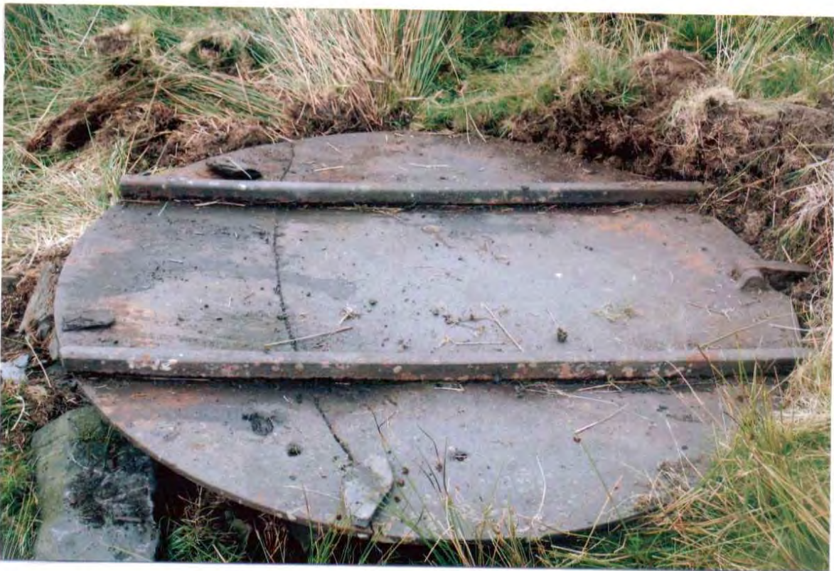
Photo 16. The top of the turntable was found at the summit level of the Cae Abatty tramway. It apparently got broken during removal, and was abandoned. The rails indicate that the gauge used in the quarry was 2' 2".
