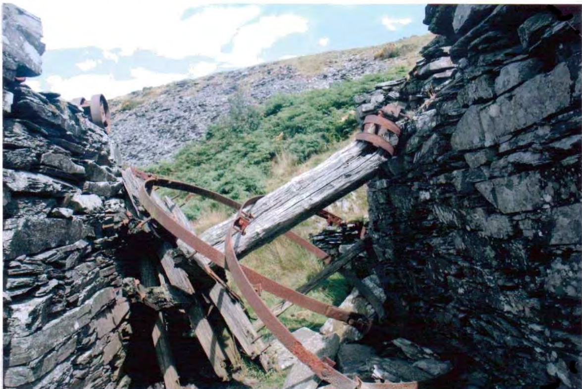
Photo 4. Looking North between the walls of the Cae Abatty Quarry Drumhouse. The drum axle has broken where it enters the West end cap, which is still on the drumhouse wall. The remains of the three drum spiders, the braking surface ring and brake band have fallen towards the West end of the axle.
