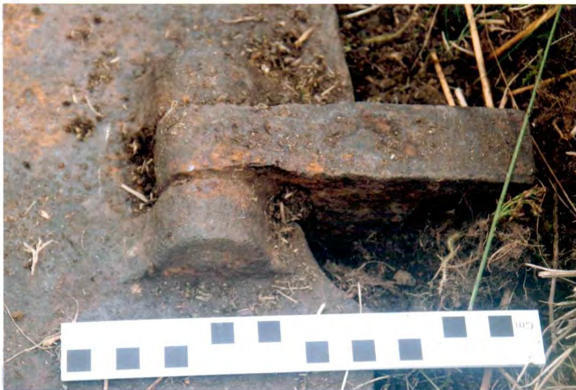
Photo 17. Latch mechanism on the turntable top.
