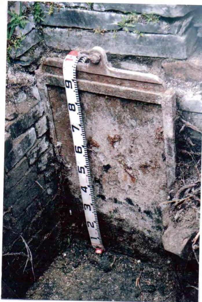
Photo 6. The damper to the chimney flue. The top 30 cm of the damper was visible above the rubble, before excavation was started.
