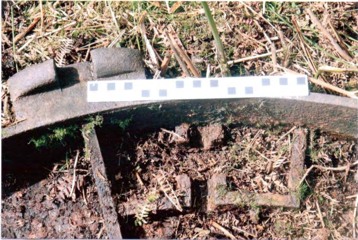
Photo 15. One of the six roller boxes on the turntable base, and one of four latching points, adjacent to the spokes.
