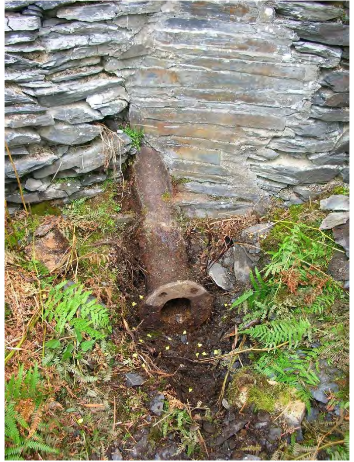
.MIN 112 cast iron pipe entering turbine building
