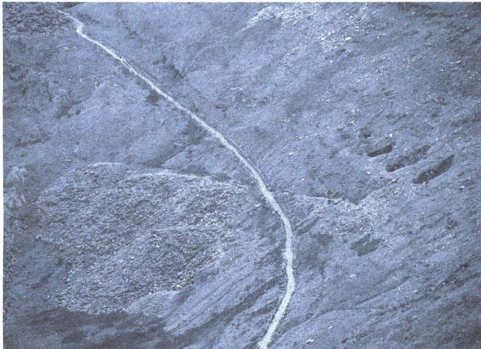
Photograph 1. A General View of the Site in August 2005. The track rising Cwmorthin to Rhosydd cuts through the tip from floor C whilst the tips from floors B and A can be seen below. On the hillside above are the open chambers C1, C2, C3 and C5.
