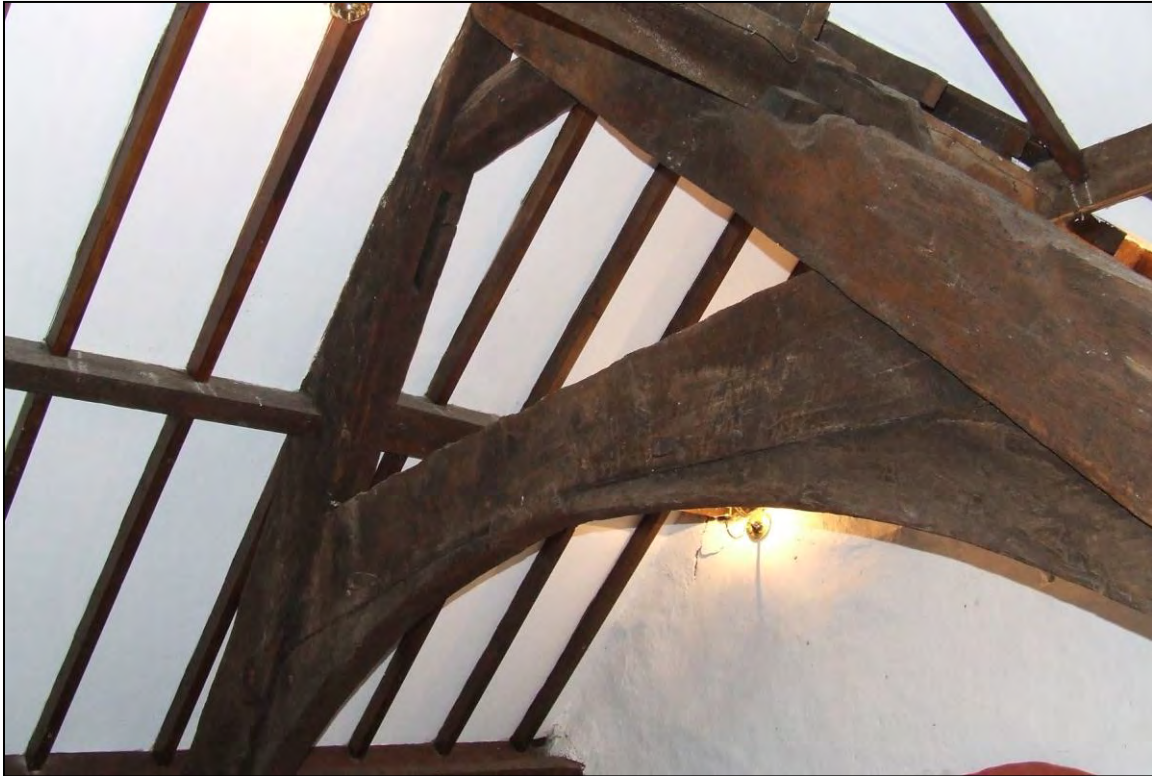
Figure 1: Cruck-truss at Cynfal Fawr.
