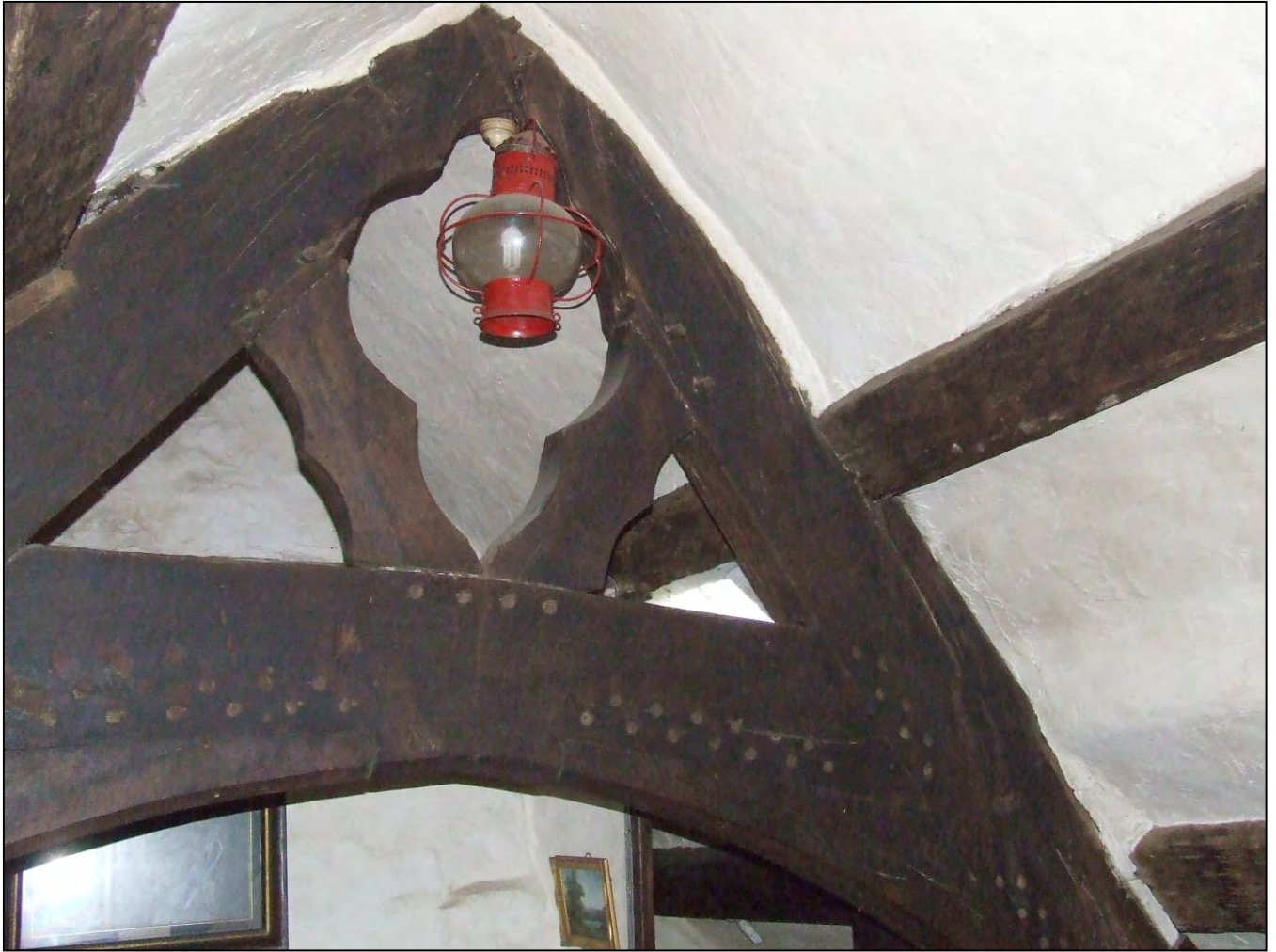
Figure 2: Photograph of the elaborate central truss
