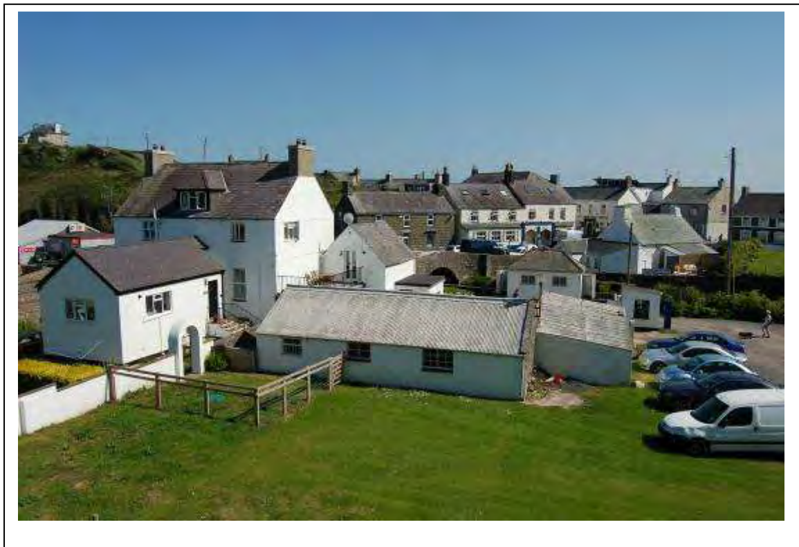
Plate 10: Outbuildings from the north
