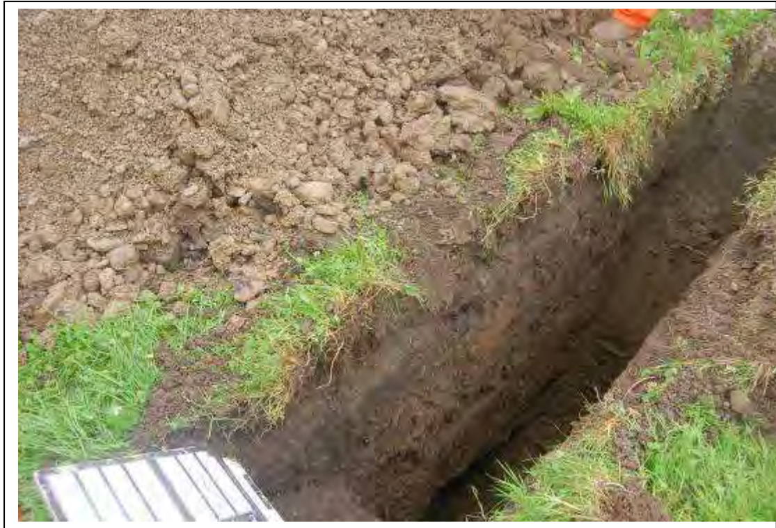
Plate 13: Test pit 2, looking west
