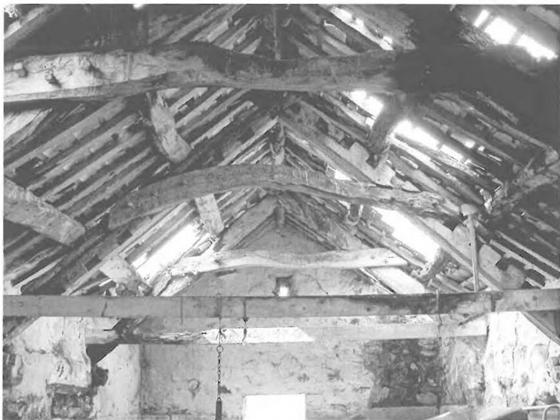
Figure 24 i. Mortised chamfered beams reused in Hafod Rhisgl cowhouse
