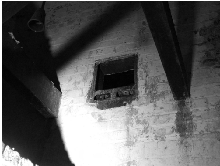
Plate 42 - Bearing box on south wall of E8
