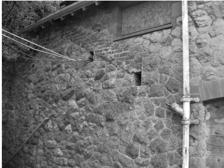
Plate 15 - Roof scar on stable block, looking southeast
