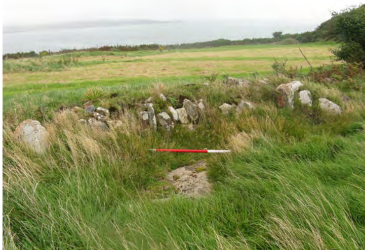
Plate 25 - Random built clawdd wall
