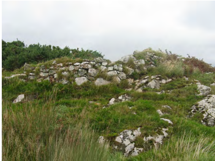
Plate 19 - Random built clawdd wall
