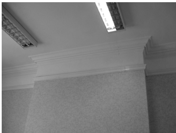
Plate 48 - Cornicing in Room 1 on chimney breast
