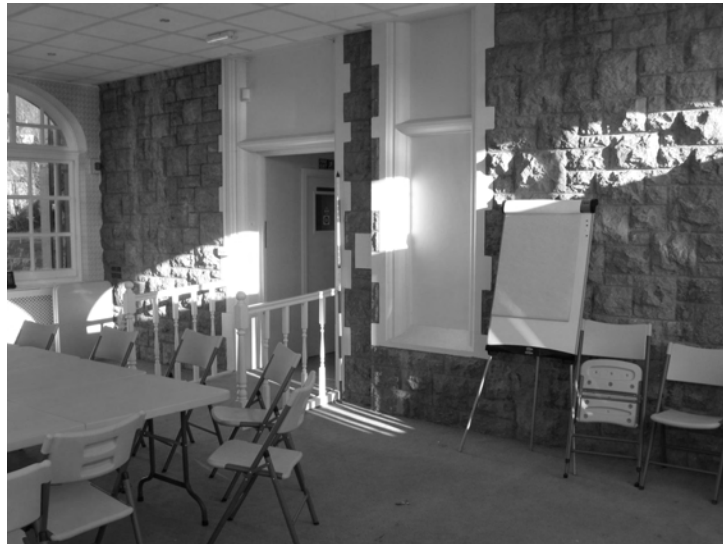
Plate 57 - South wall of room 92 showing blocked up window and entrance
