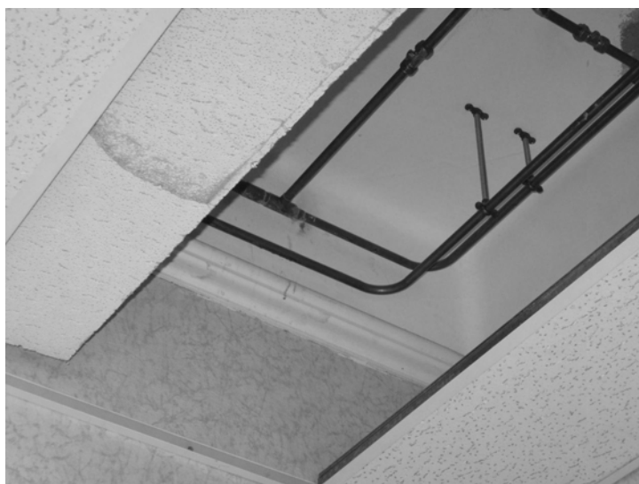
Plate 59 - Architrave hidden by lowered ceiling
