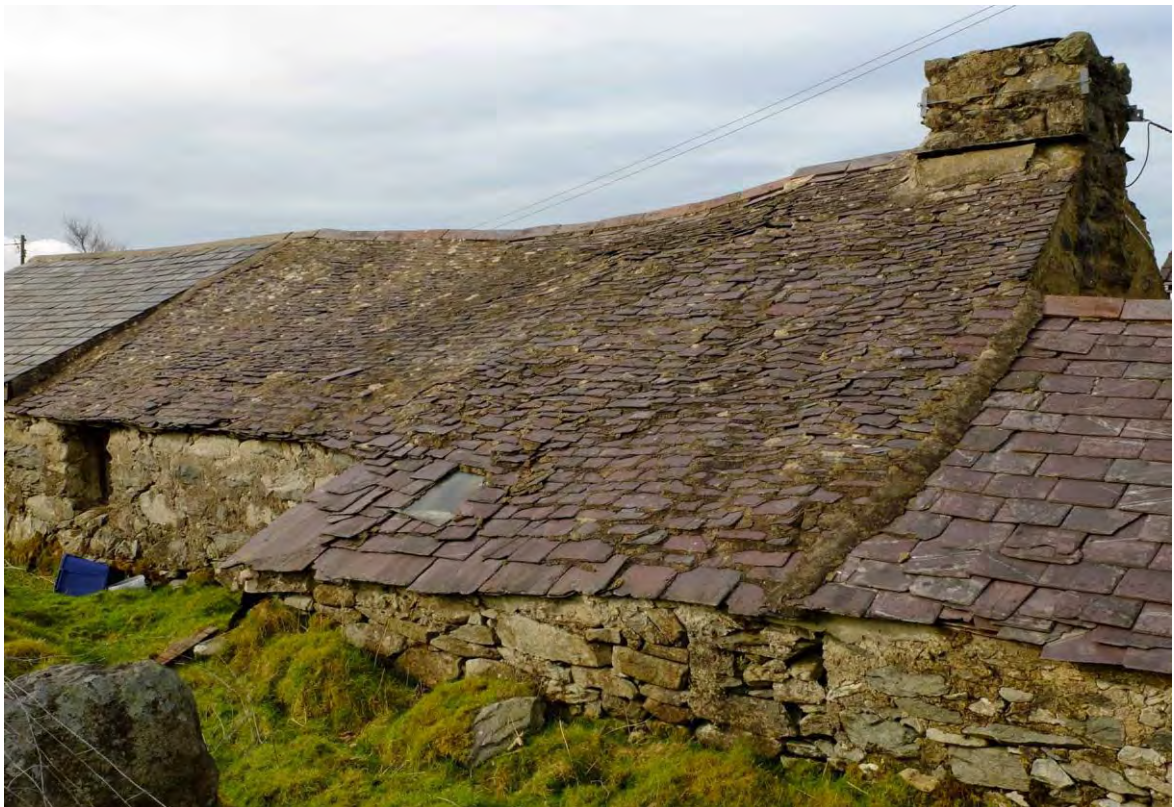
Fig 17 The old cottage at Bryn Tirion in Cilgwyn has a roof of generally poor-quality small slates, maintained by grouting.
