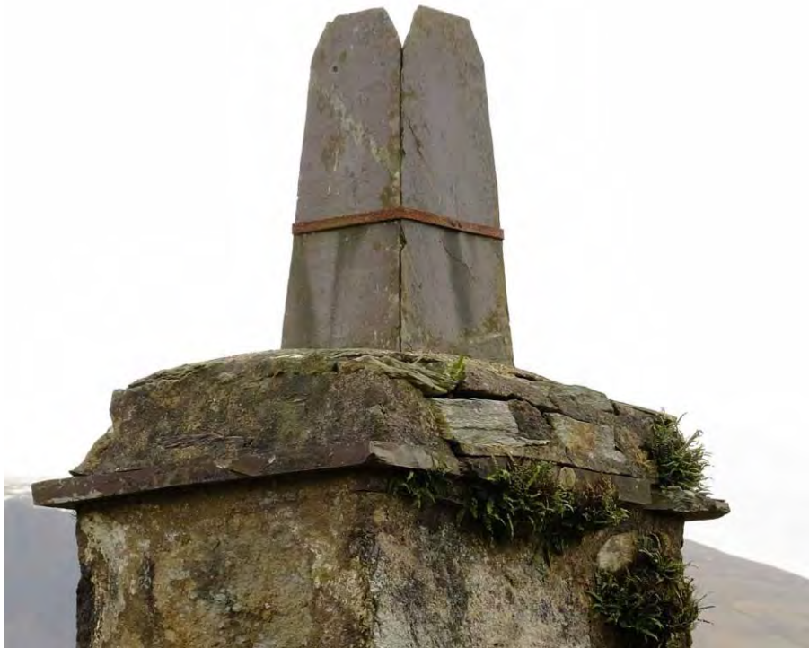
Fig 20 Slate chimney pot, Cilgwyn
