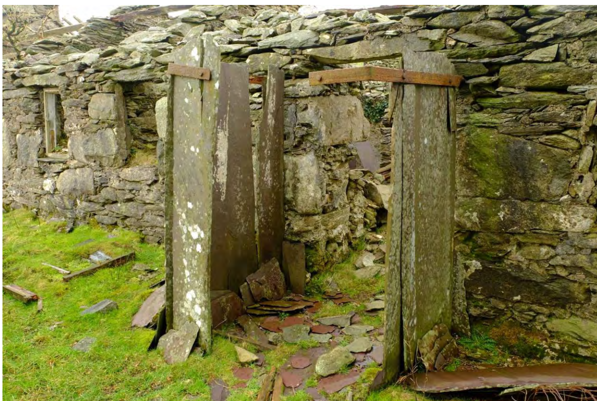
Fig 19 Storm porch of slate slabs at Pen-ffynnon-wen, Cilgwyn
