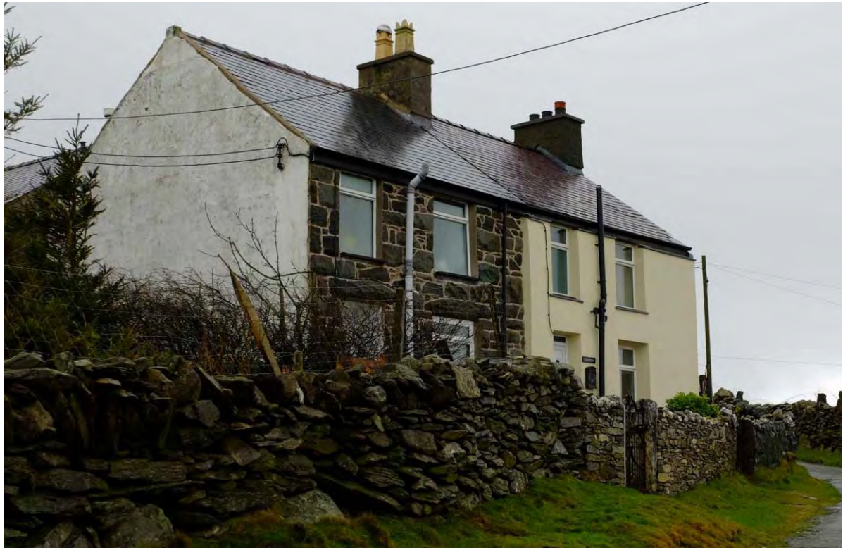
Fig 12 Two-storey houses in Cilgwyn
