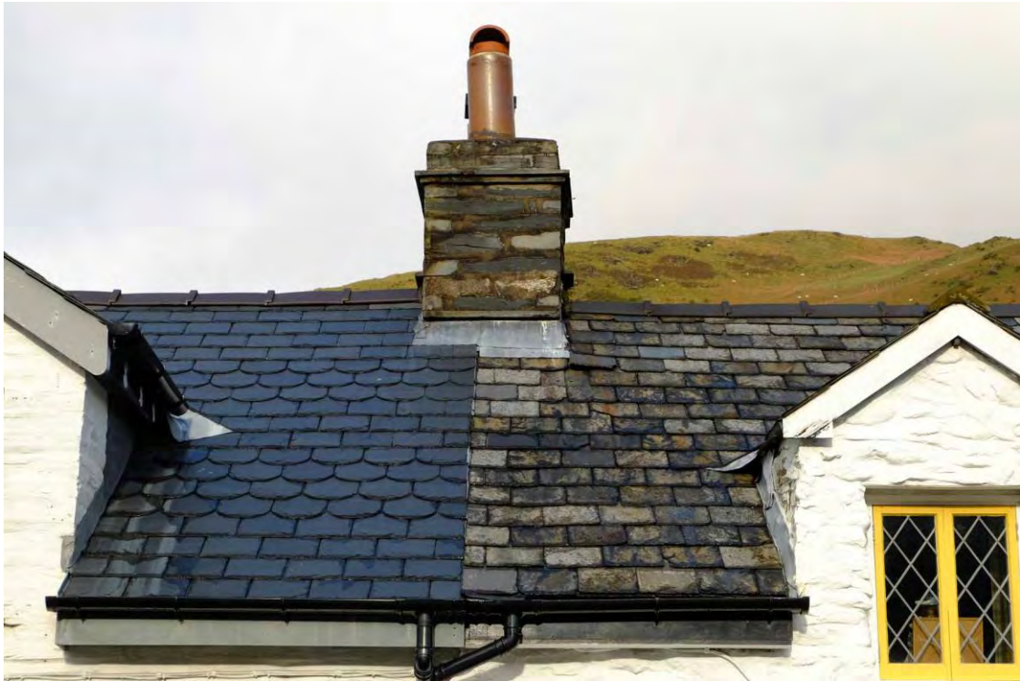
Fig 24 Roof slates have been replaced on many buildings, including these cottages in the village centre. The modern roof on the left has bands of fish-scale slates, historically absent from the village.
