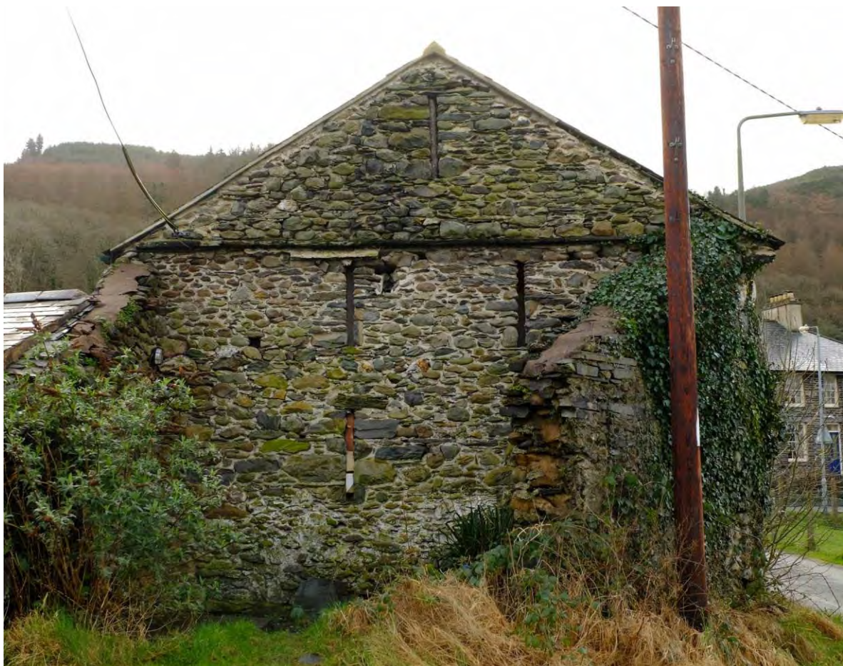
Fig 10 Outbuilding behind the Railway Inn, showing its ventilation strips and field-stone construction.
