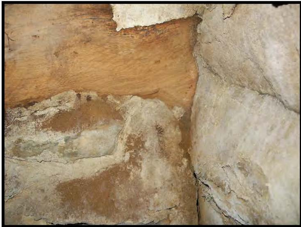
Plate 21 Basement -south end of main beam. Chamfer & stop just visible and fully located in wall with later supporting pillar underneath to the left.
