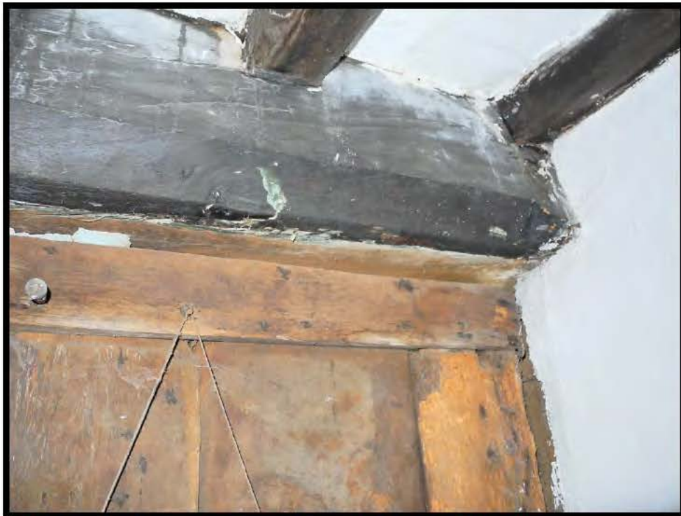
Plate 16 - Main beam over screen, chamfer & stop. No Mortise.
