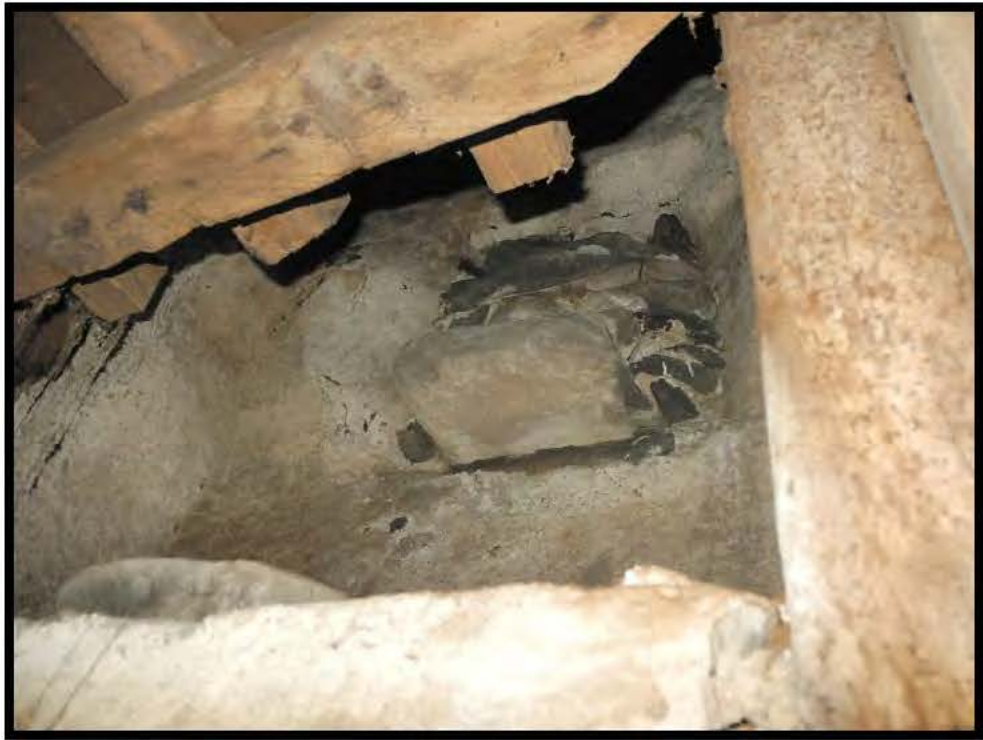
Plate 22 - Blocked cross passage door. This doorway appears to have been reduced in size leaving a small window, which can be seen has been filled in roughly with stones.
