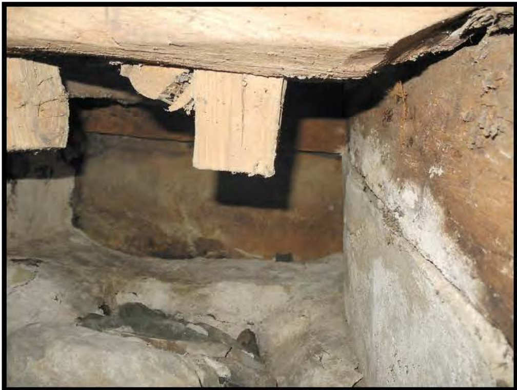
Plate 23 - In this image an oak frame is clearly seen, including head and the plaster can be seen applied to the reduced doorway.
