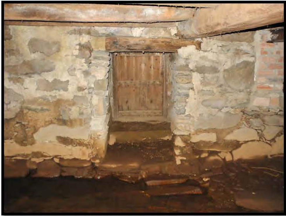
Plate 20 - Basement - external door, remodelled doorway south gable
