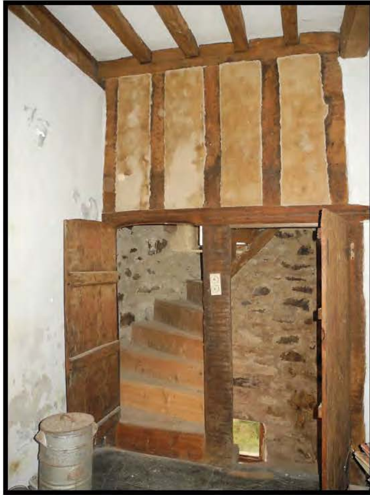
Plate 26 - Timber framed partition with doors to stairs.
