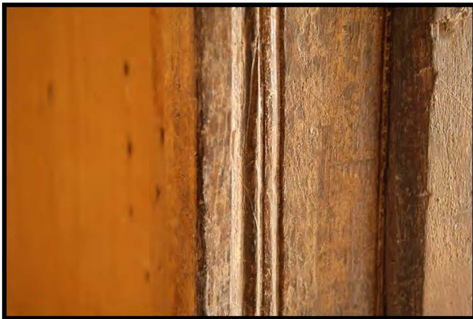
Plate 13 - door post south screen remnant. Moulding typical of 16th C
