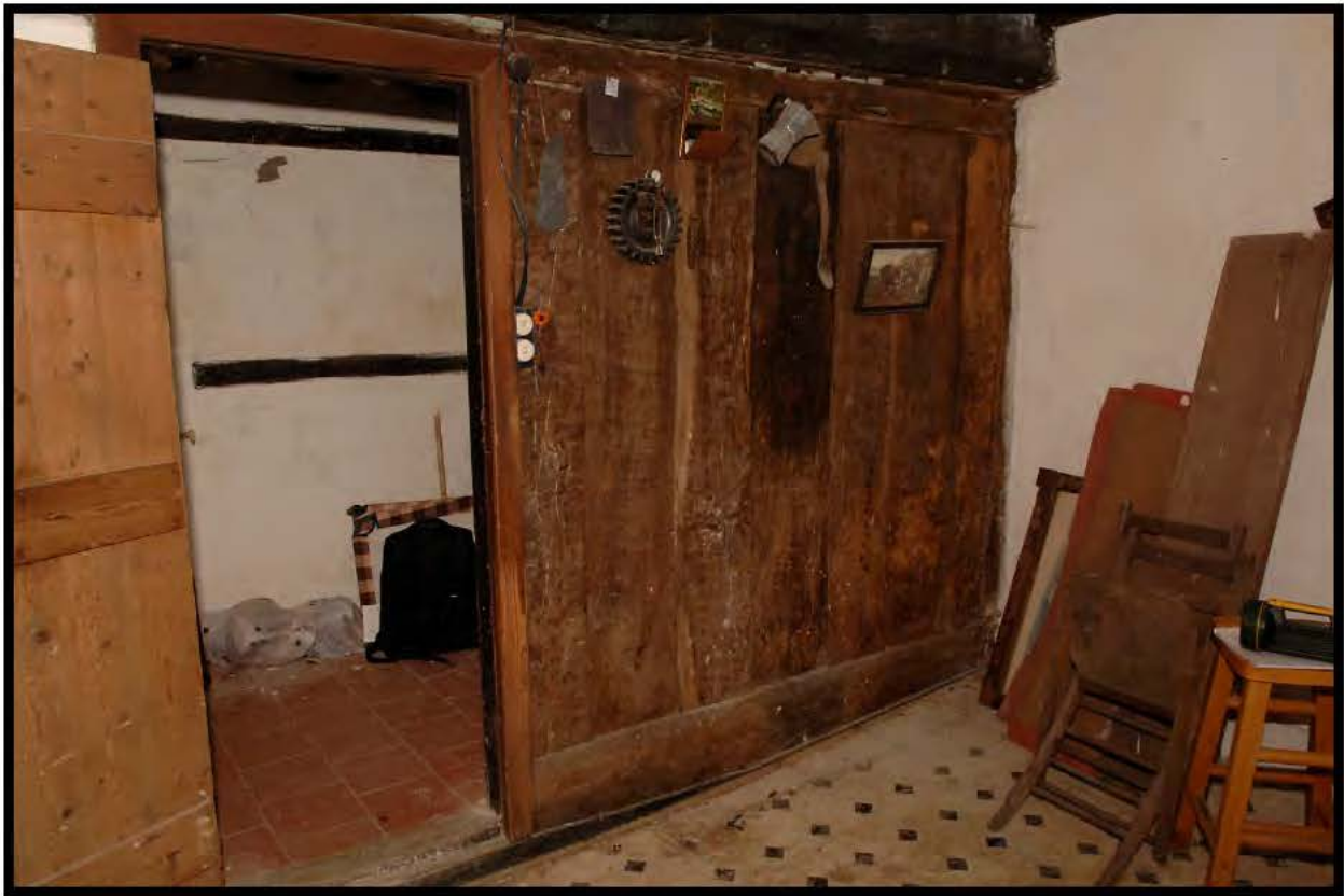
Plate 15 - Part of passage screen. Service room.
