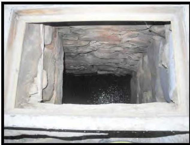
Plate 19 - Latrine chute directly over stream.
