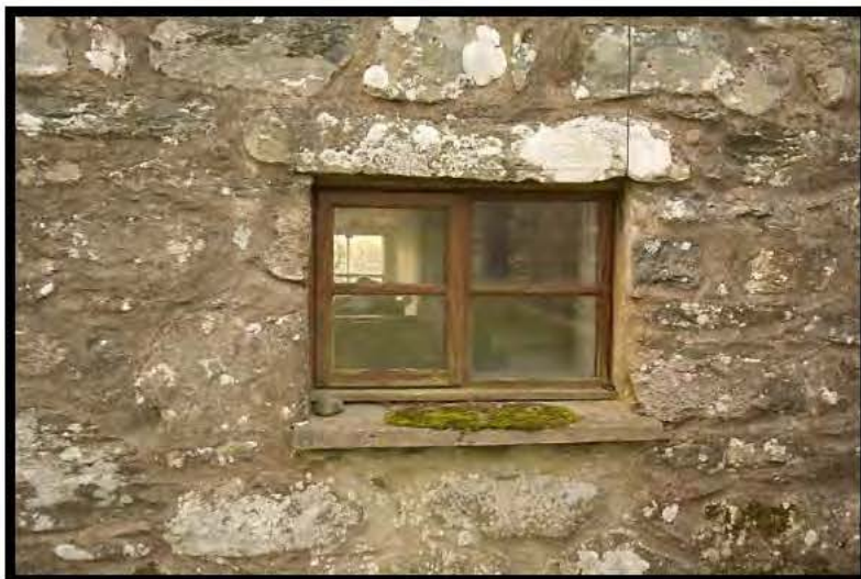
Plate 11 - Hall window with modern casement.
