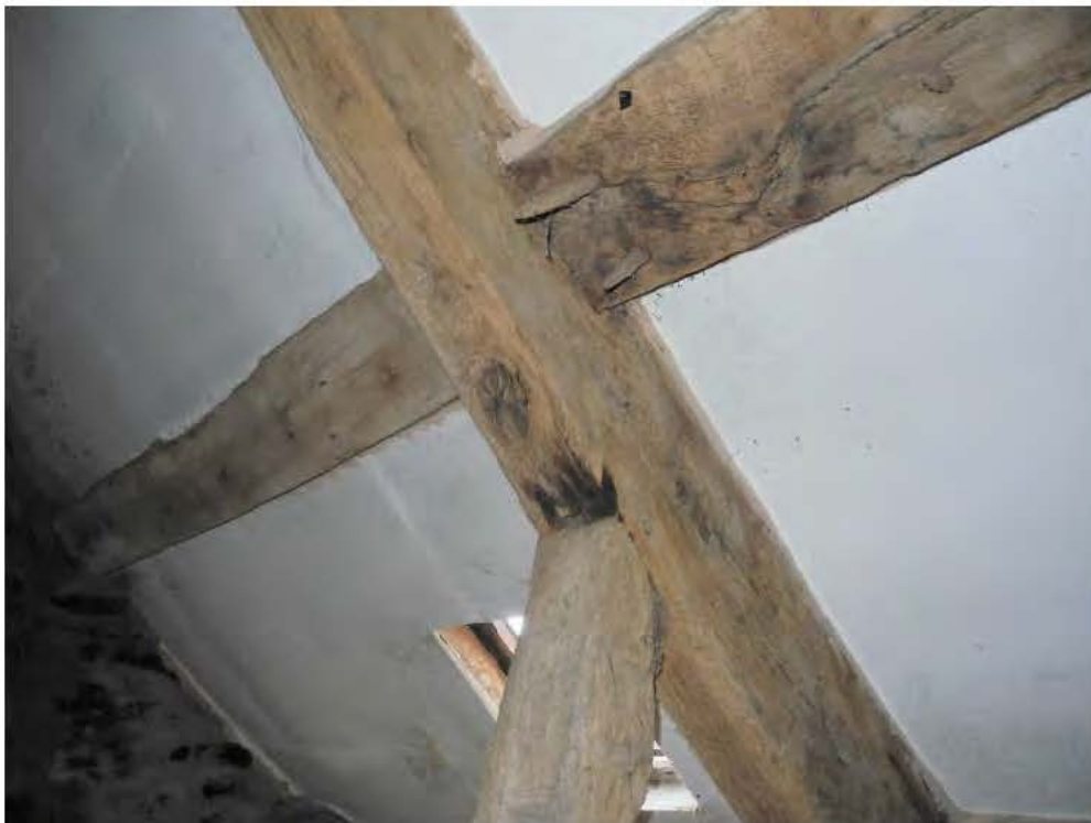
Plate 31 - Purlins scarf jointed with raking strut support below. Note scorch marks.
