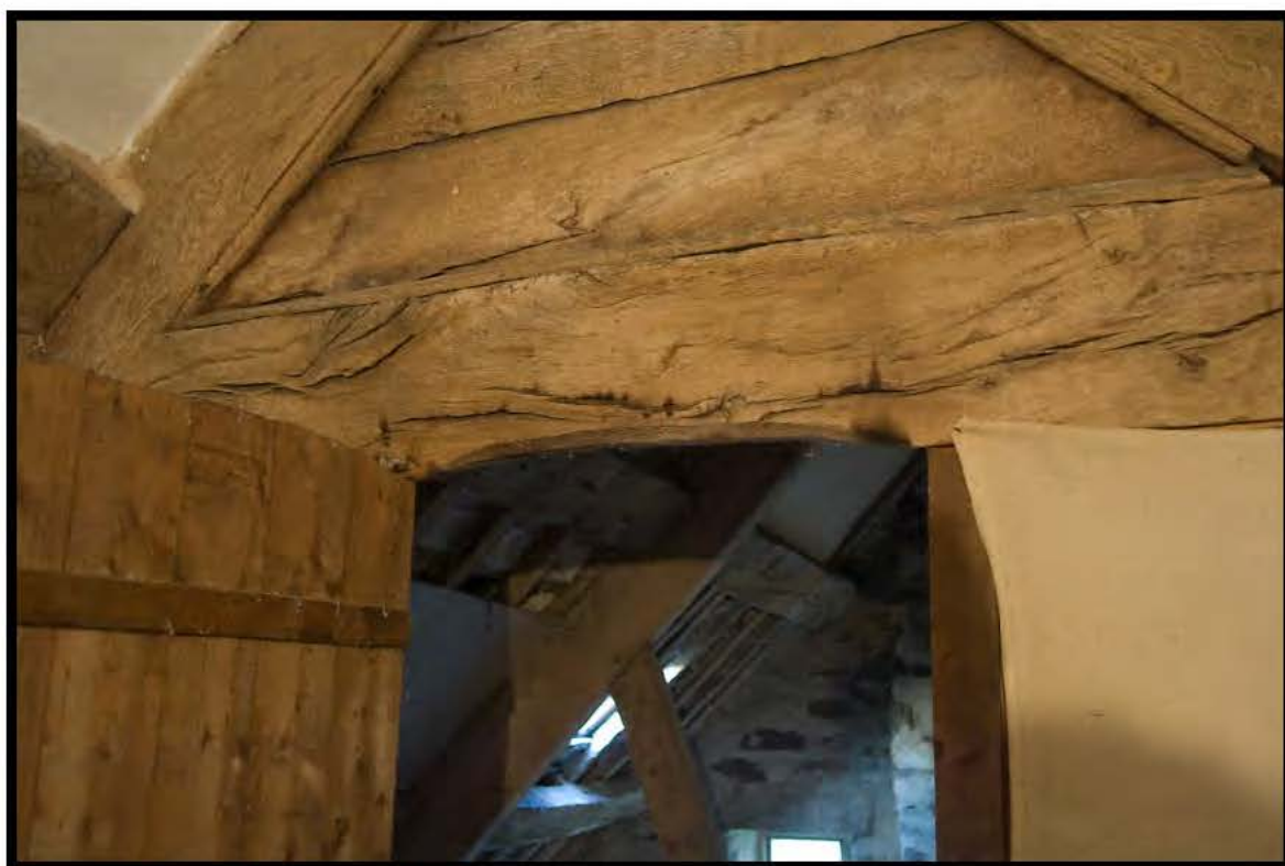
Plate 36 - Truss 2 collar door head
