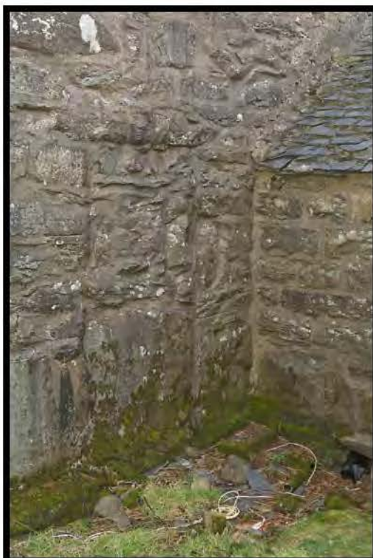
Plate 10 - Cross passage blocked doorway
