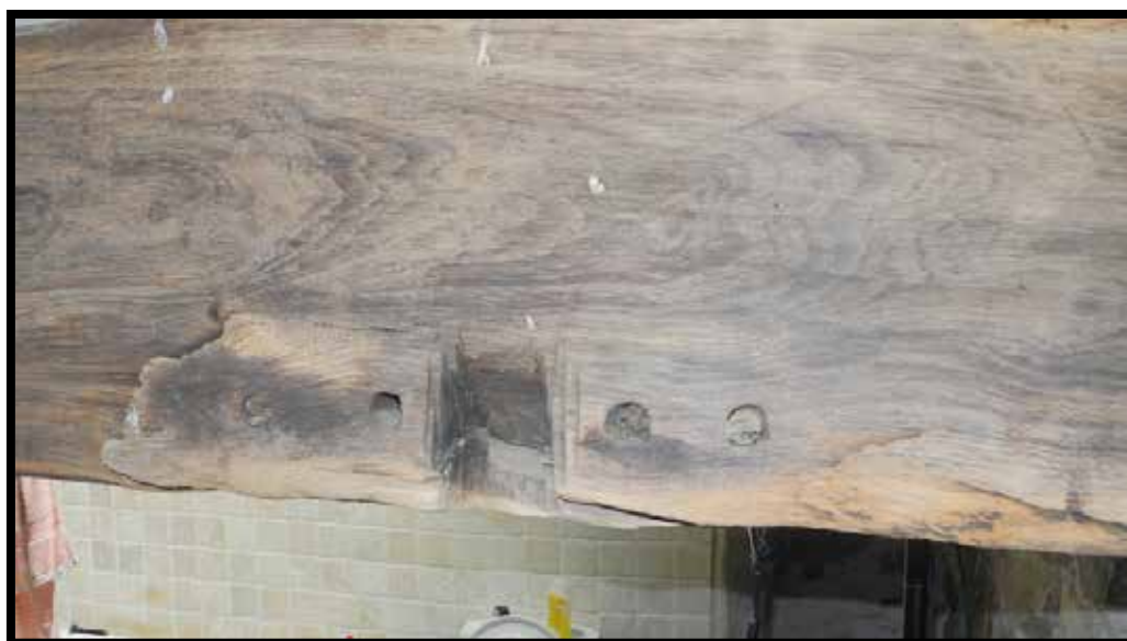
Plate 32: T3: base of principal and tie-beam; housing & peg holes –close-up
