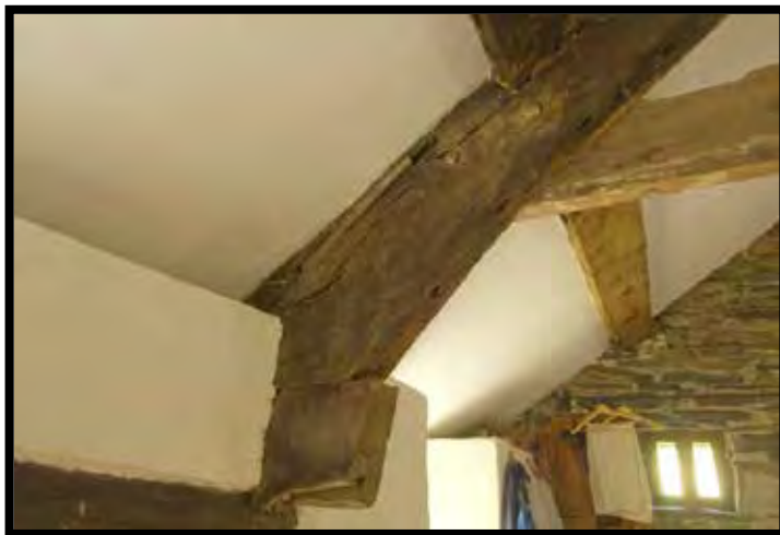
Plate 22: T1 – truncated tie beam
