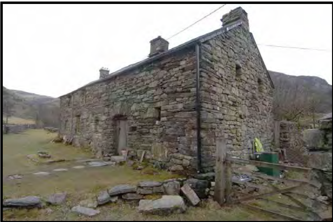
Plate 2: Front elevation & SW rebuilt gable
