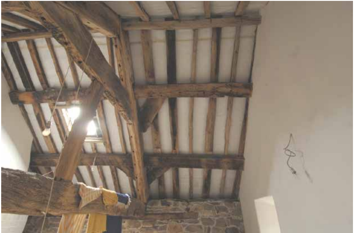
Plate 33: T3: rafters & wind braces
