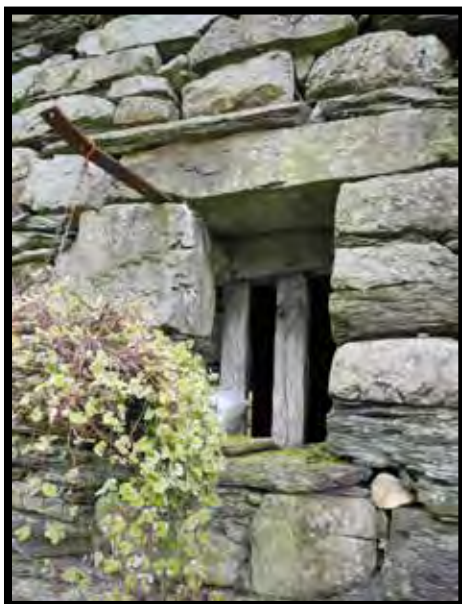
Plate 4: Front elevation mullion window
