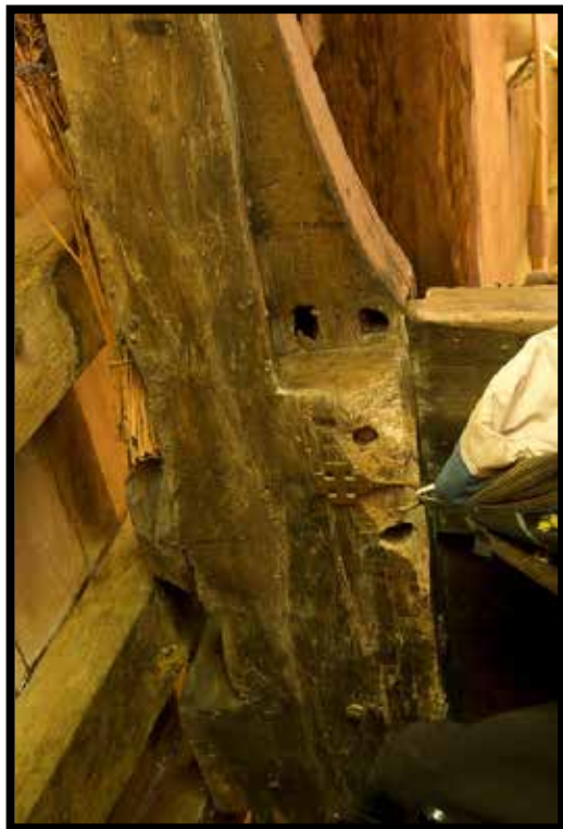
Plate 13: Rear side of dais partition; door head L
