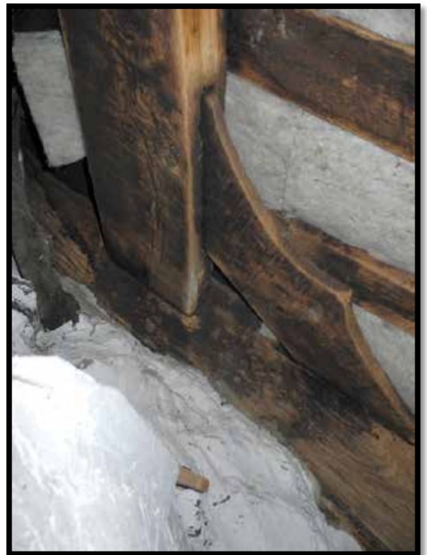
Plate 27: T2E: eastern principal -wind brace detail
