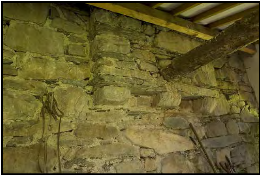
Plate 6: NE gable – corbelled external chimney breast
