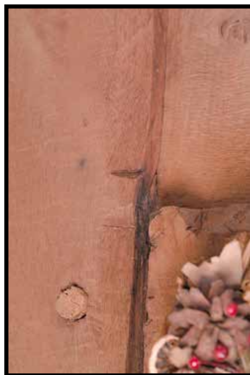
Plate 16: Screen detail – nailhead stop & chamfers
