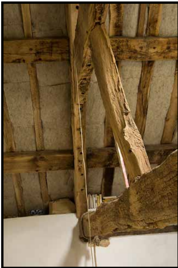
Plate 29: T3: truss showing erosion, stave holes
