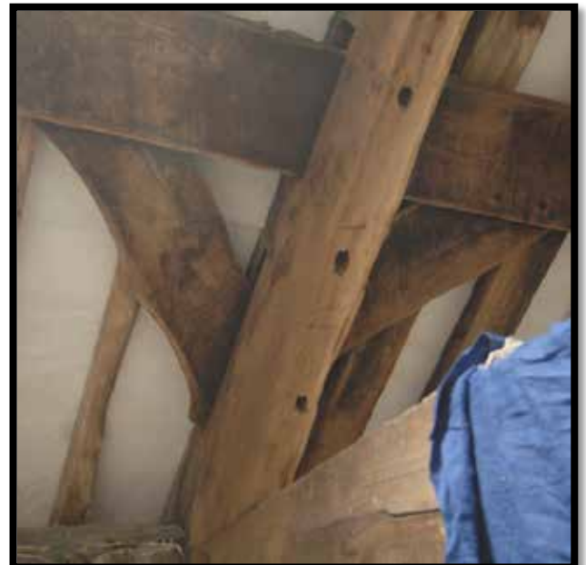
Plate 30: T3: wind braces and stave holes
