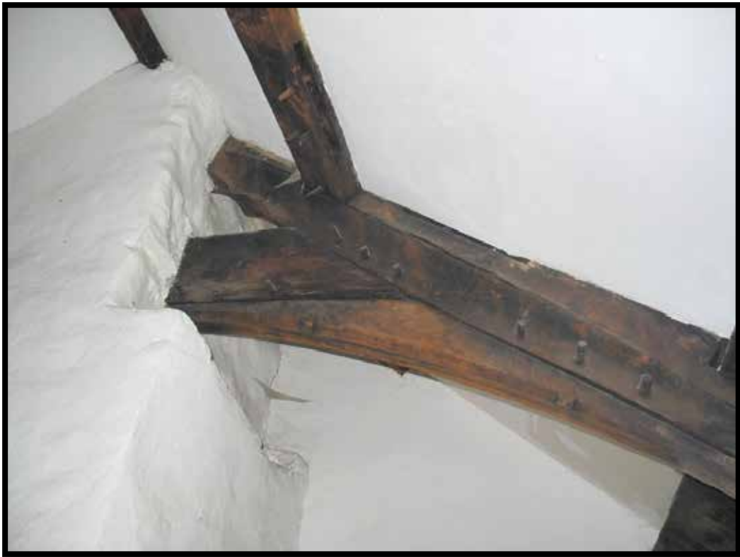
Plate 25: T2W: Pegs, wind brace mortise; smoke black
