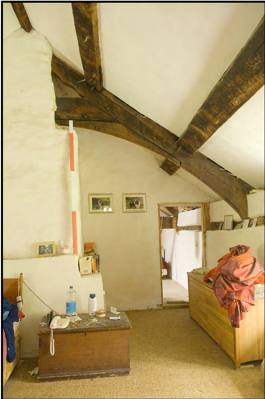
Plate 24: T2W: arch-braced truss from north east
