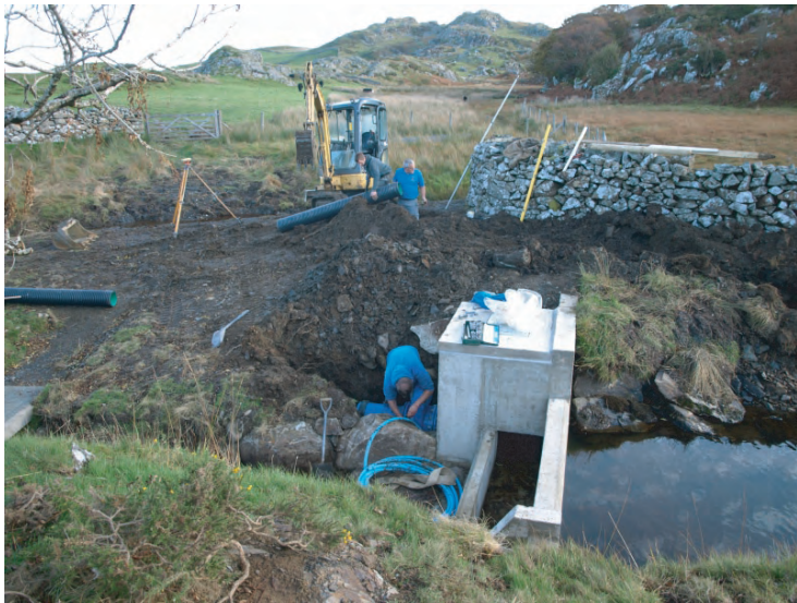
Plate 24. View of Intake 2 during working shot for trench work joining trench to Forebay tank.
