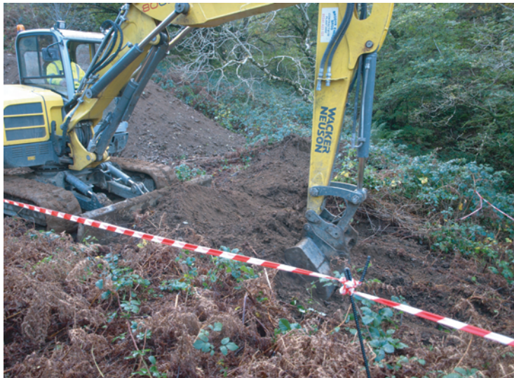
Plate 41. Working shot during trenching for penstock on downslope through bracken.
