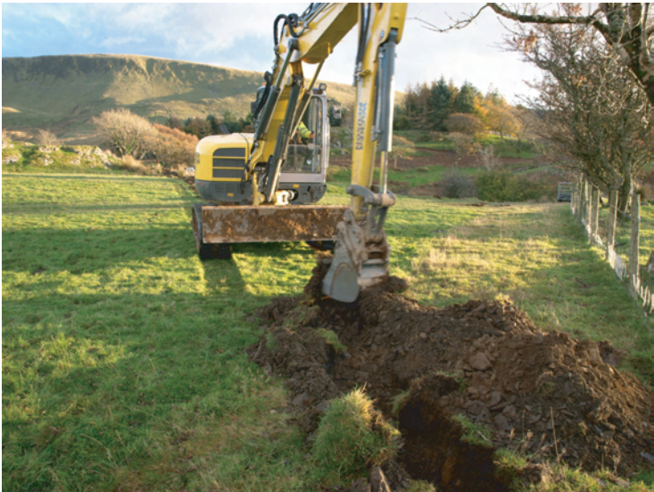
Plate 31. Working shot during trench cutting from Forebay tank to main Penstock. Looking southeast toward Forebay tank frp, trackway.
