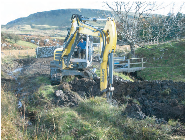
Plate 27. Working shot during trench cutting from Intake 2 to Forebay tank. Looking southeast.
