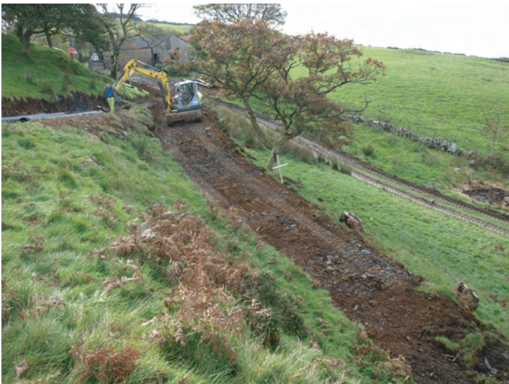
Plate 10. Working shot during groundwork for pipeline leading from Intake 1 to Forebay tank. Area of rock outcrop. Looking northwards.
