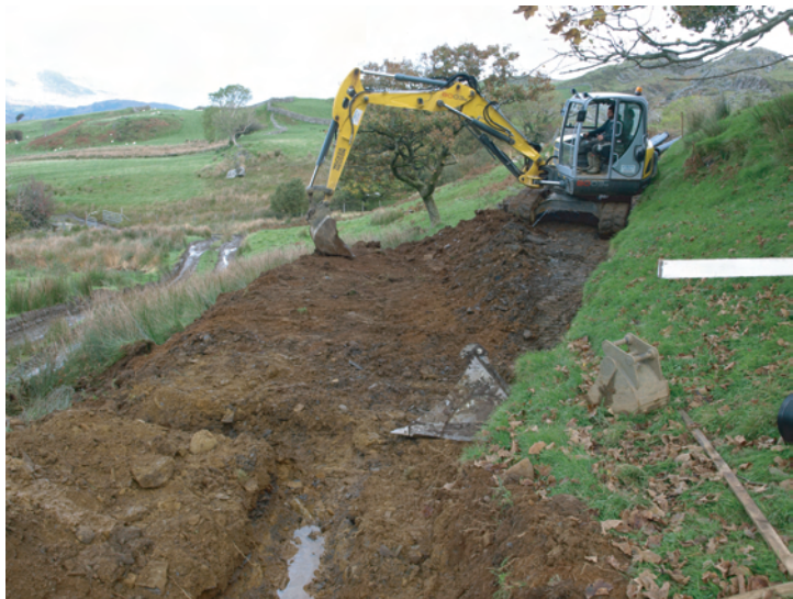
Plate 9. Working shot during groundwork for pipeline leading from Intake 1 to Forebay tank. Area of rock outcrop. Looking northwards.
