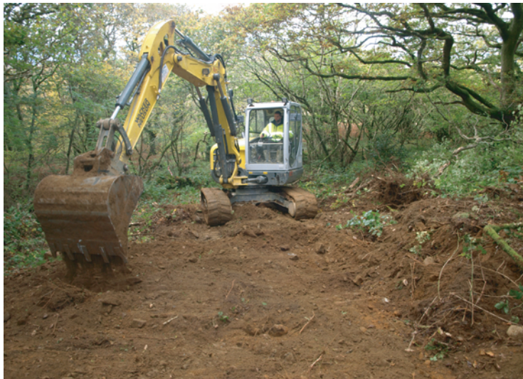
Plate 45. Working shot during groundwork for penstock through woodland. Looking northwest.
