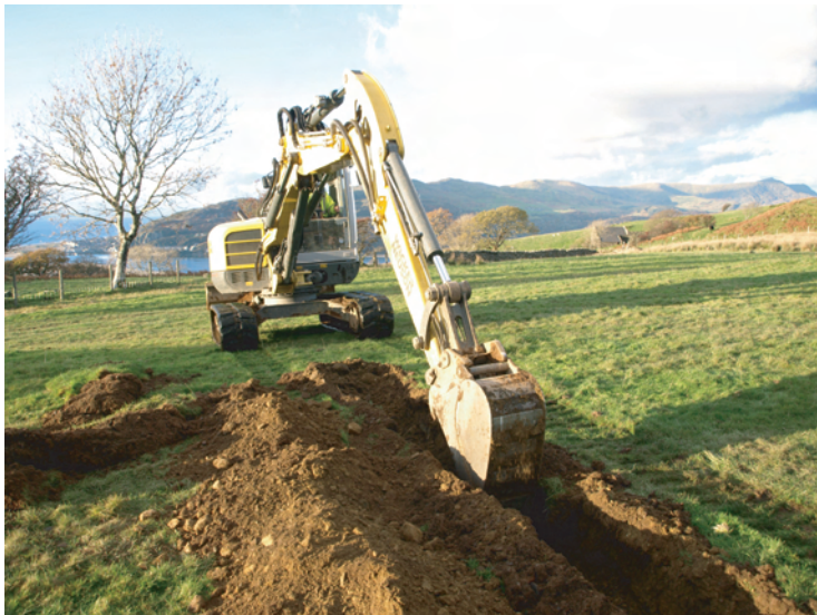
Plate 29. Working shot during trench cutting from Forebay tank to main Penstock. Looking northwest.
