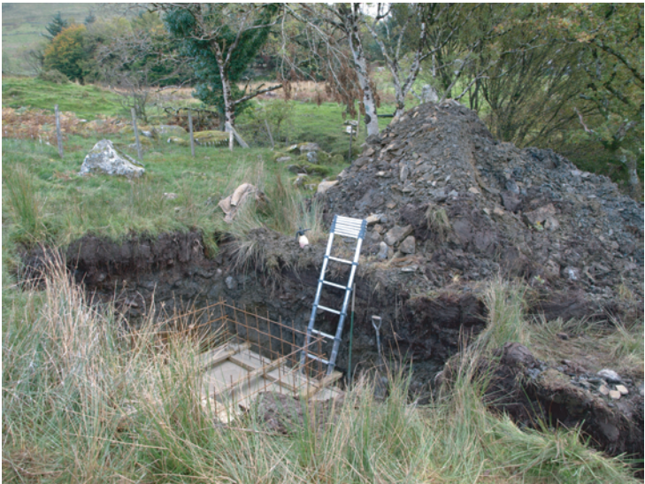
Plate 19. Forebay tank under construction. Looking southeast.
