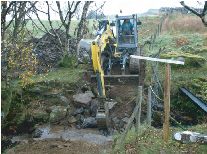
Plate 14. Working shot during groundwork for area crossing stream leading to Forebay tank.
