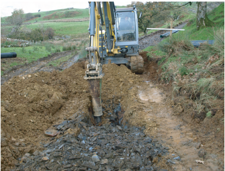
Plate 8. Working shot during groundwork for pipeline leading from Intake 1 to Forebay tank.
