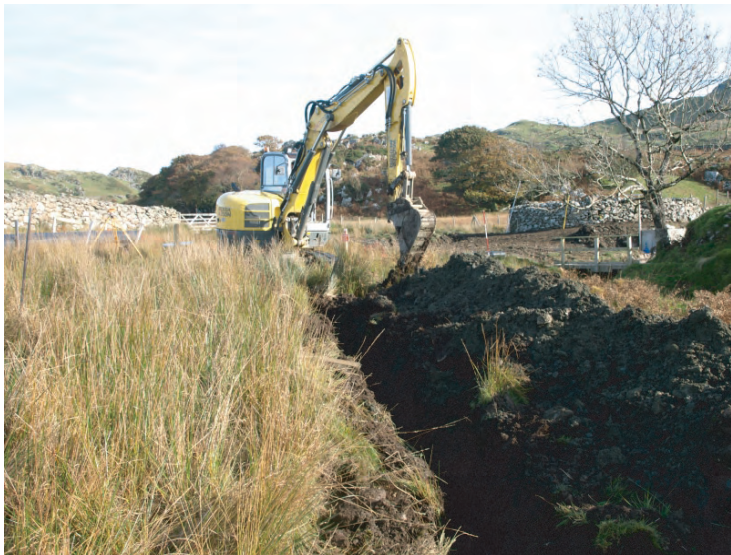
Plate 26. Working shot during trench cutting from Intake 2 to Forebay tank. Looking southeast.
