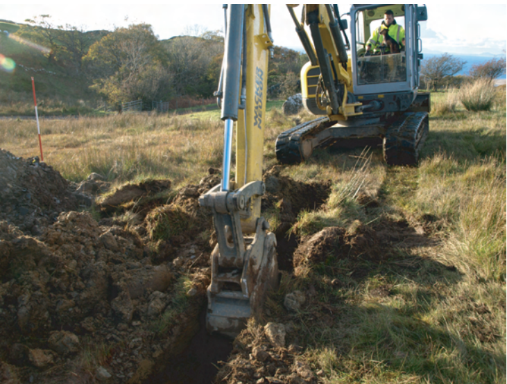
Plate 28. Working shot during trench cutting from Forebay tank to main Penstock. Looking northwest.
