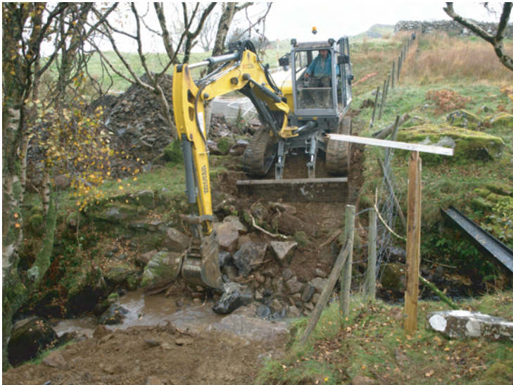
Plate 20. Working shot during trench cutting to Forebay tank from Intake 1. Looking northwards.
