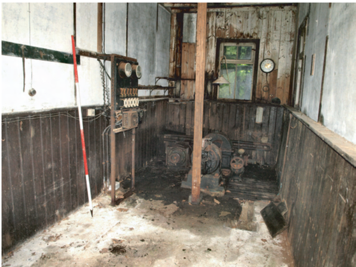
Plate 27. Interior of part of former coach house/garage showing former hydro-electric switch gear and turbine at Bron Meirion.
