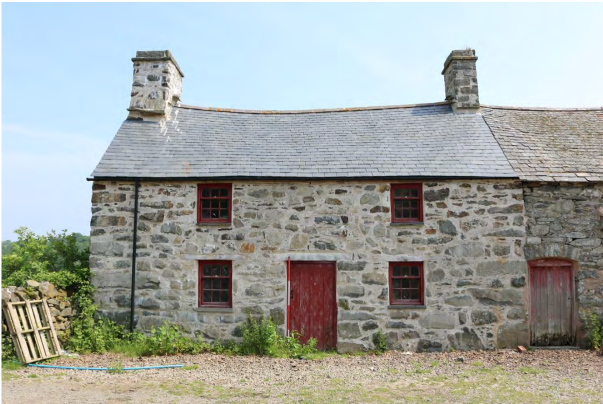
Maes yr Hendre cottage (building B) SH 7922 6747
