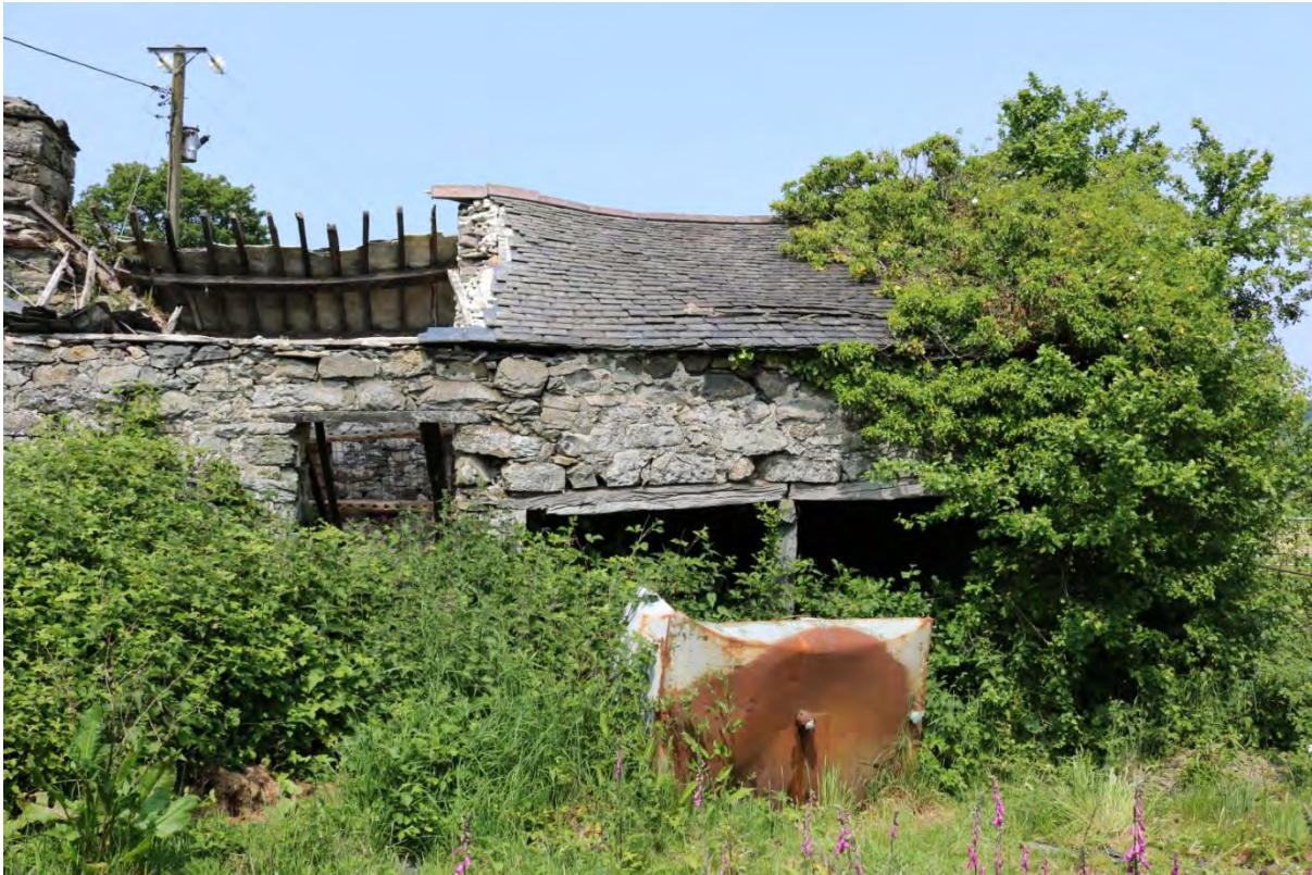
Cart shed (building G)SH 7920 6752
