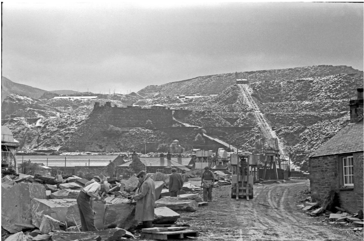
Figure 16: This view of Penrhyn quarry dated 1966 shows the transition period from railways to dumper trucks and fork-lifts, and shows how inclined planes were still the prominent features in the quarry landscape, as are roads now. © NMGW: 2018.6/38.
