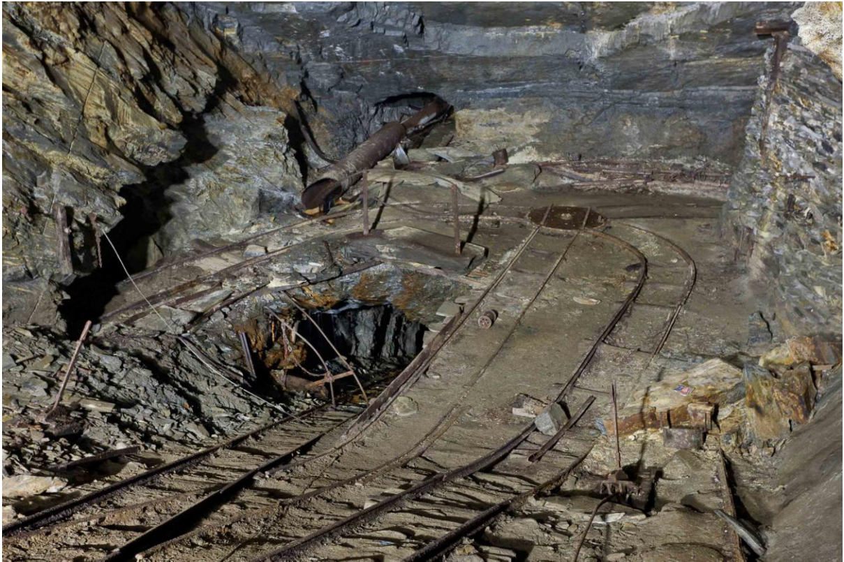
The intermediate landing which gave the New Ffridd incline access to floor A is a well-preserved example of how one inclined plane could be made to serve many floors in the underground slate workings of Ffestiniog. NPRN: 546428; PRN: 67455.
