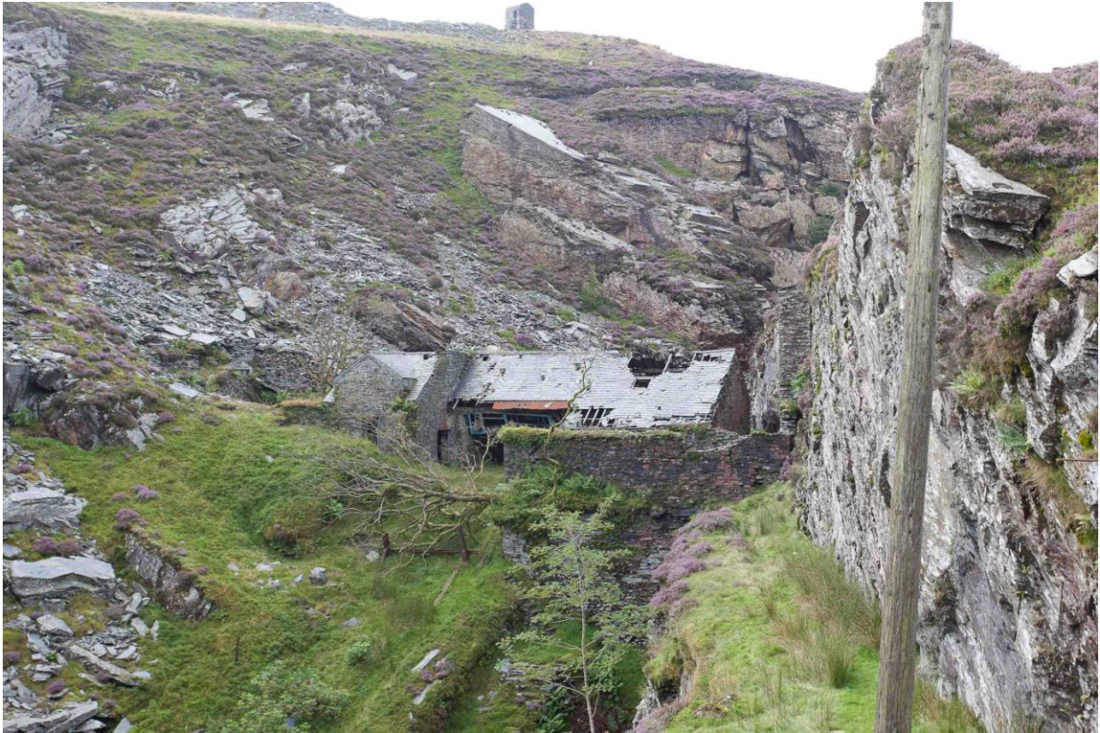
The Back Vein incline gave access to the underground workings at Maenofferen Slate Quarry and was known to the quarrymen as inclên Idris after one of its operators. It is the best surviving example of a once-common technology in the Ffestiniog slate industry, an up-haulage incline raising blocks and rubble to daylight. NPRN: 54615; PRN: 67462.
