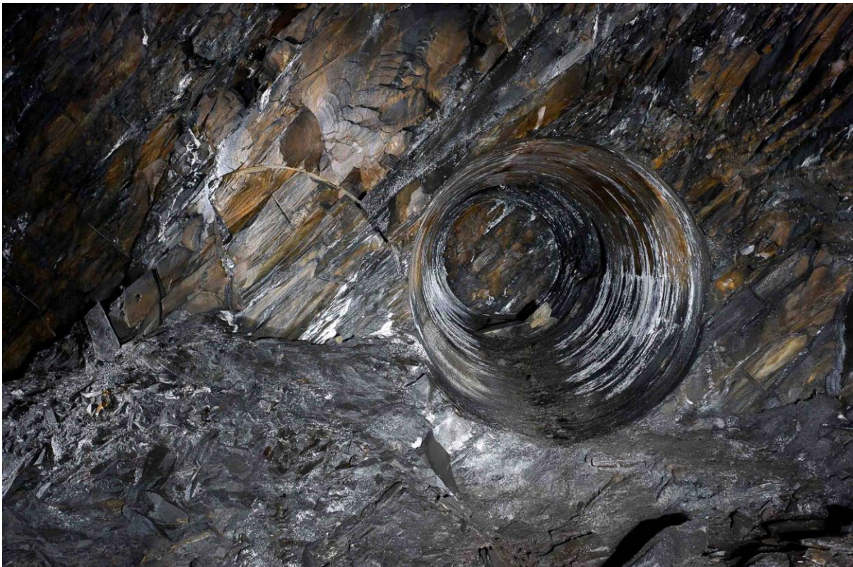
A circular section tunnel on floor 2 has been cut by a Hunter boring machine. NPRN: 546447; PRN: 67473.
