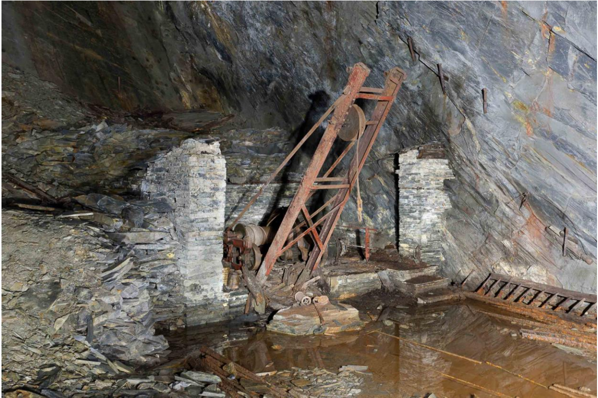
Chamber DE/1 (West) in the Back Vein demonstrates the wealth of artefactual survival underground, including the motor, winding drum, reduction gearing and unique crane-type pulley support for an up-haulage incline. NPRN: 546413; PRN: 67487.
