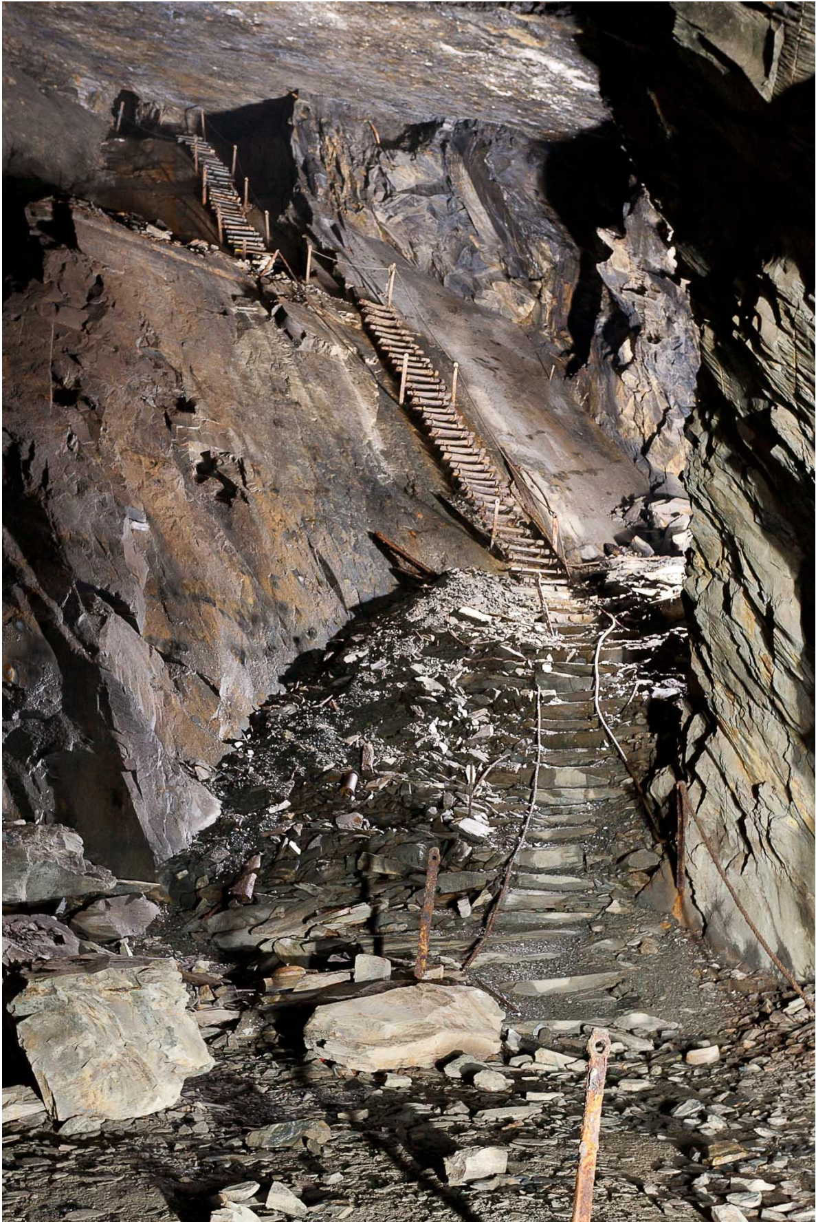
The slate-slab stairway connecting Floor C and Floor 1 in Cwmorthin Slate Quarry is a good example of a once-common feature. NPRN: 546414; PRN: 67488.
