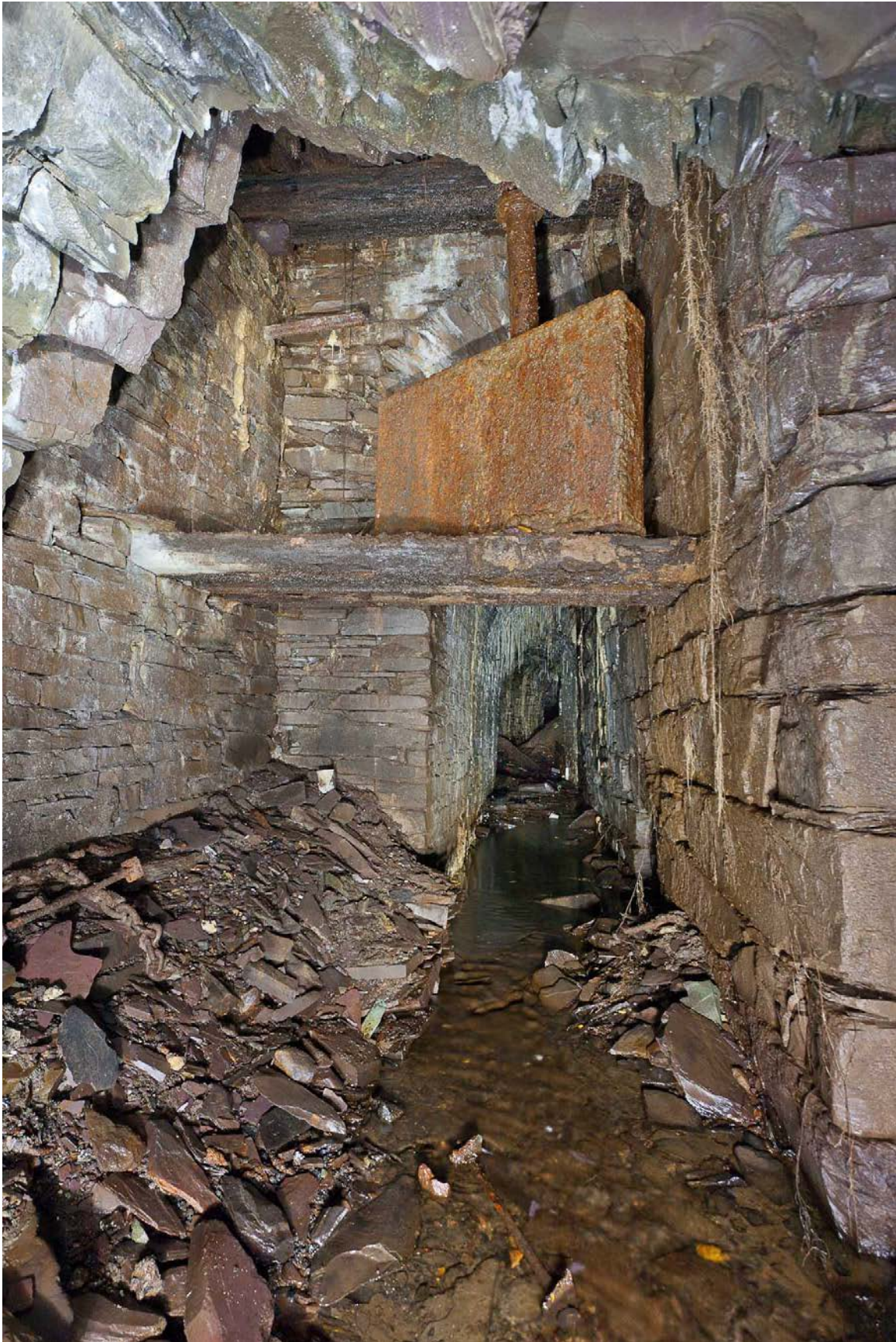
The water wheel formerly located in the pit (right) in the Tal y Sarn Slate Quarry drainage level powered a pump and may have powered a haulage system. NPRN: 546401; PRN: 67450.
