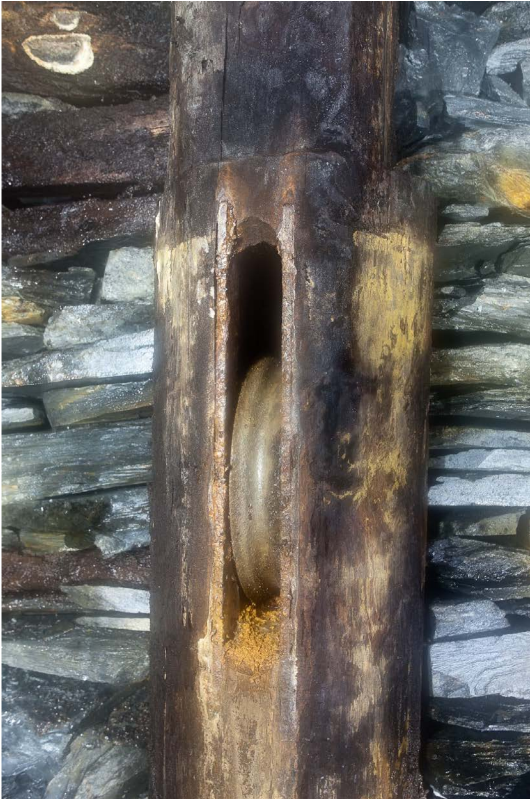
Ships' derricks have been re-used as supports in Floor 1 in the Back Vein. NPRN: 546408; PRN: 67482.
