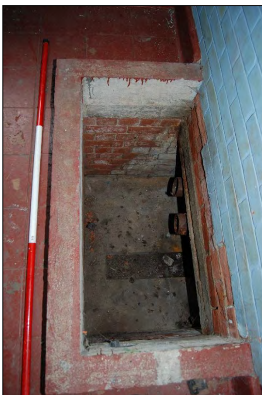
Plate 234: The pit in which the heating pipes leave the Boiler House
