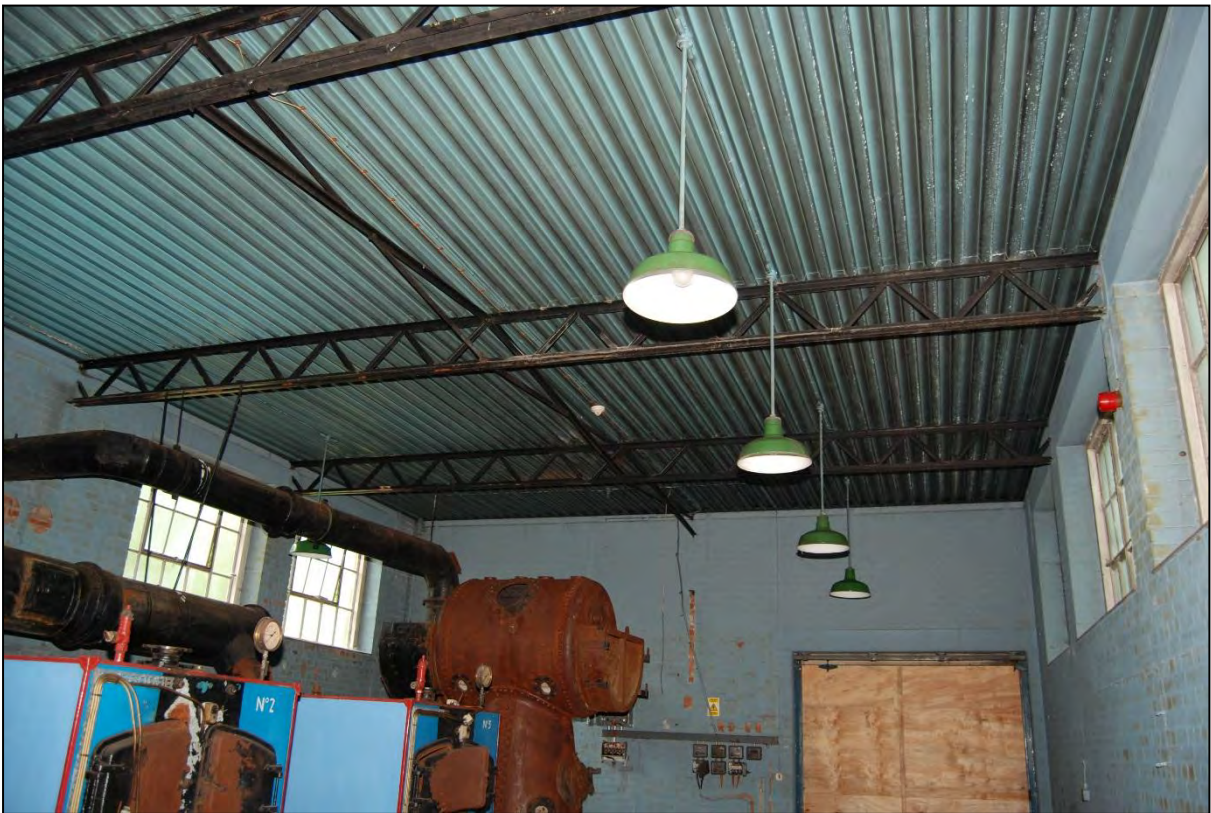
Plate 236: The roof structure of the Boiler House
