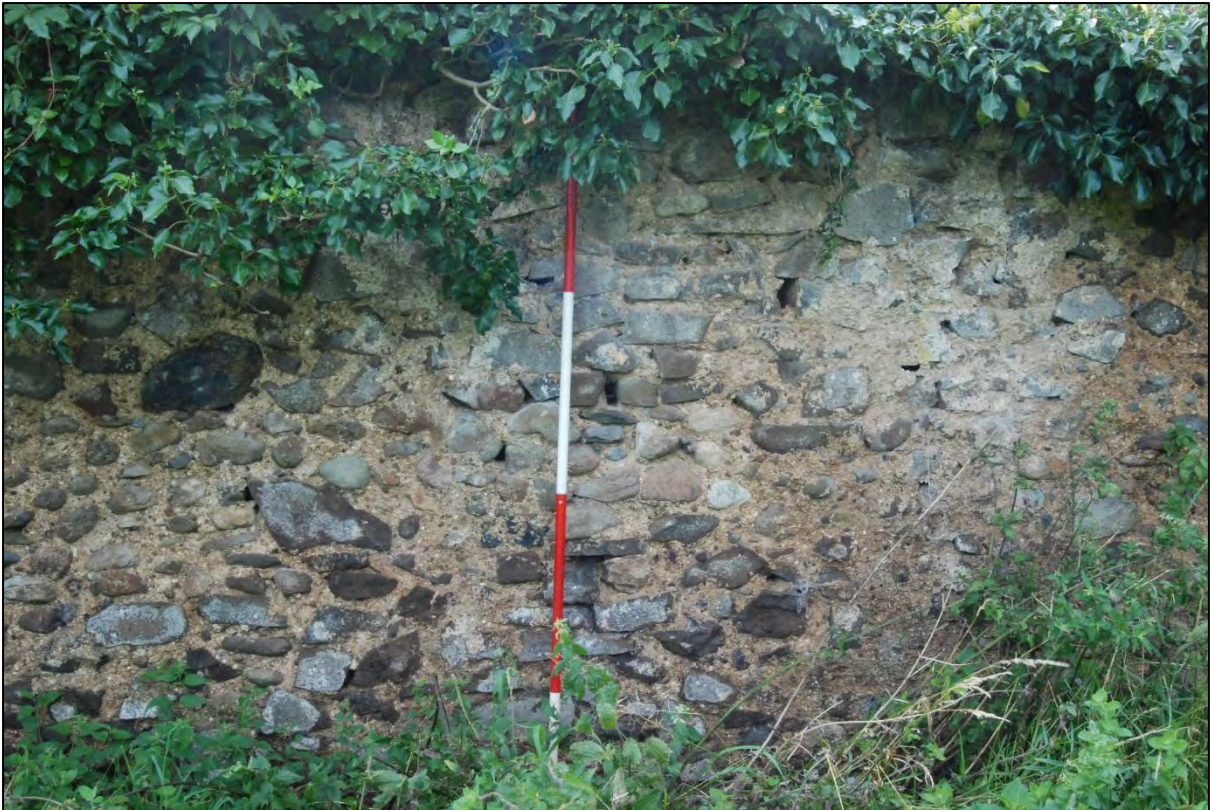
Plate 57: Patch with small stones and lime mortar between Buttresses 1 and 2 in the Walled Garden
