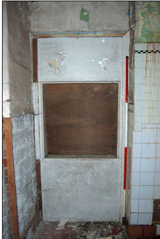
Plate 113: Blocked opening between the Kitchen and Room 10
