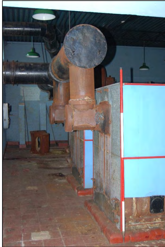
Plate 229: The exhaust system of the boilers
