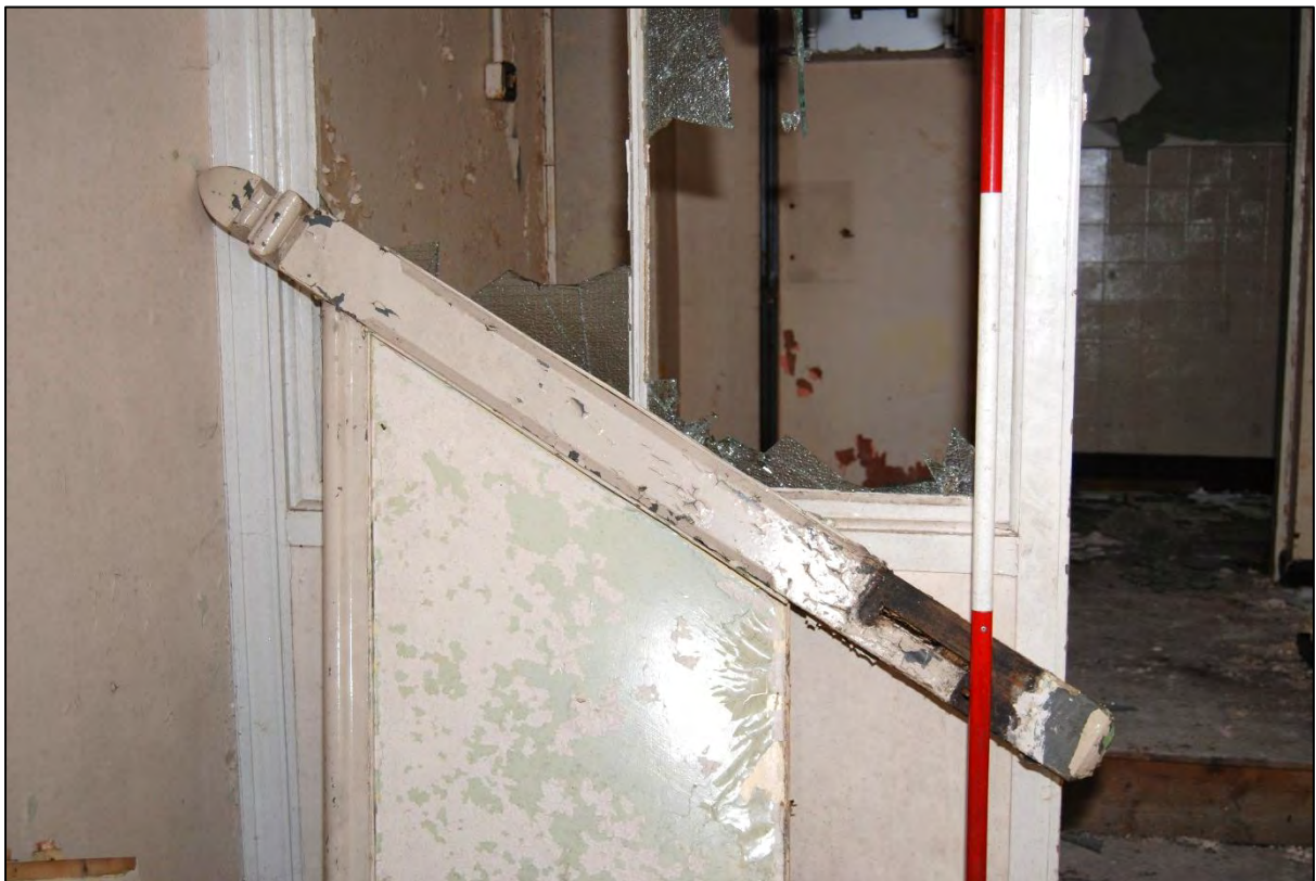
Plate 159: Newel post and handrail for the back staircase.
