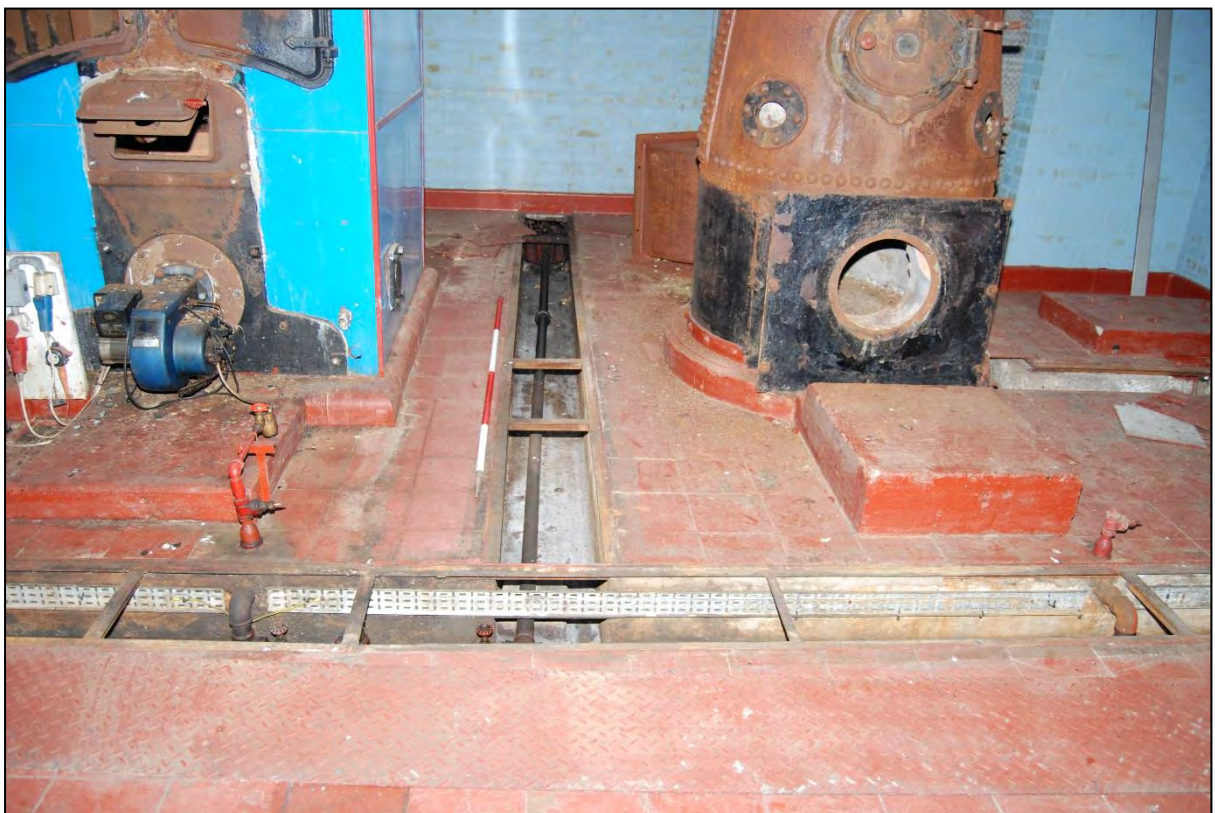
Plate 230: Trough in the floor of the Boiler house
