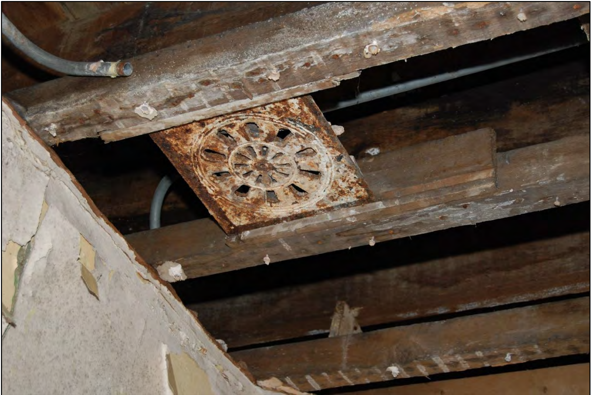
Plate 153: Perforated iron plate in the ceiling of Room F8
