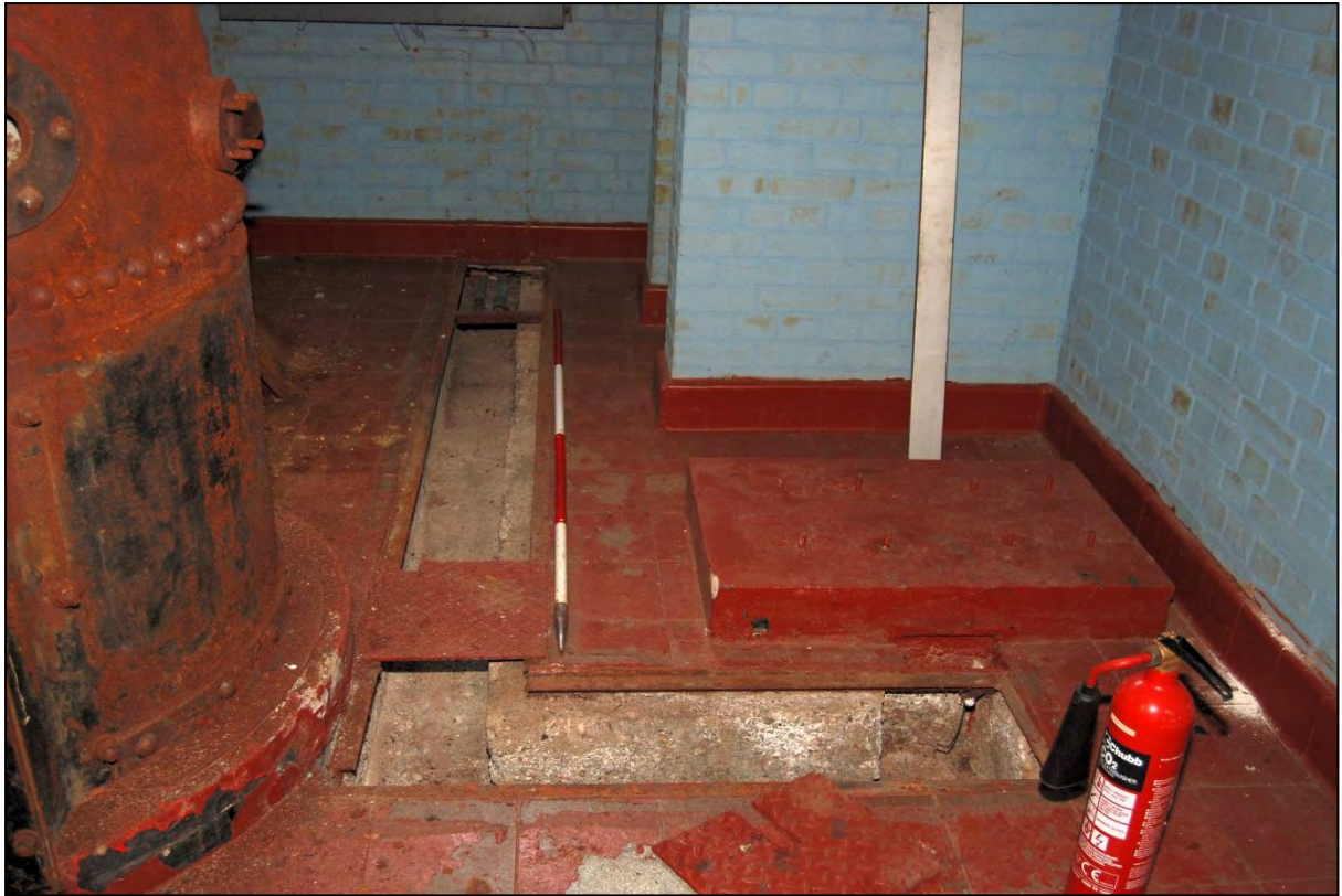
Plate 231: Trough in floor of the Boiler House
