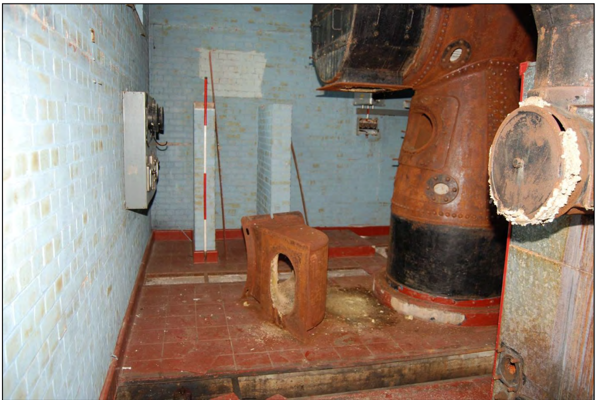
Plate 232: Stub walls, possible tank support in the Boiler House
