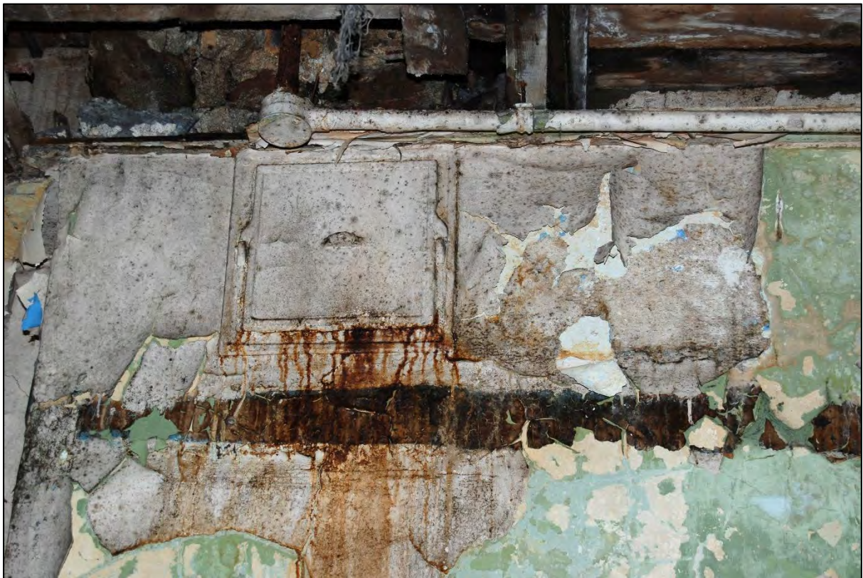
Plate 114: Hatch for cleaning the chimney in the Kitchen
