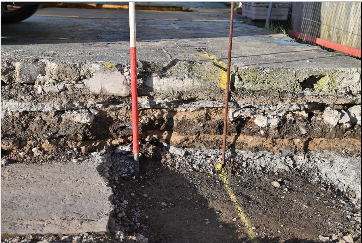
Plate 4: Section through the concrete layers covering part of the site
