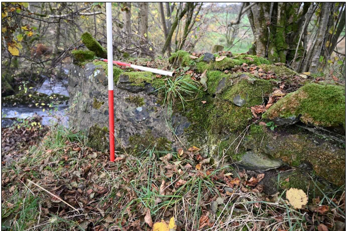
Plate 16: Junction between the stone bank and mortared stone wall on the northern bank
