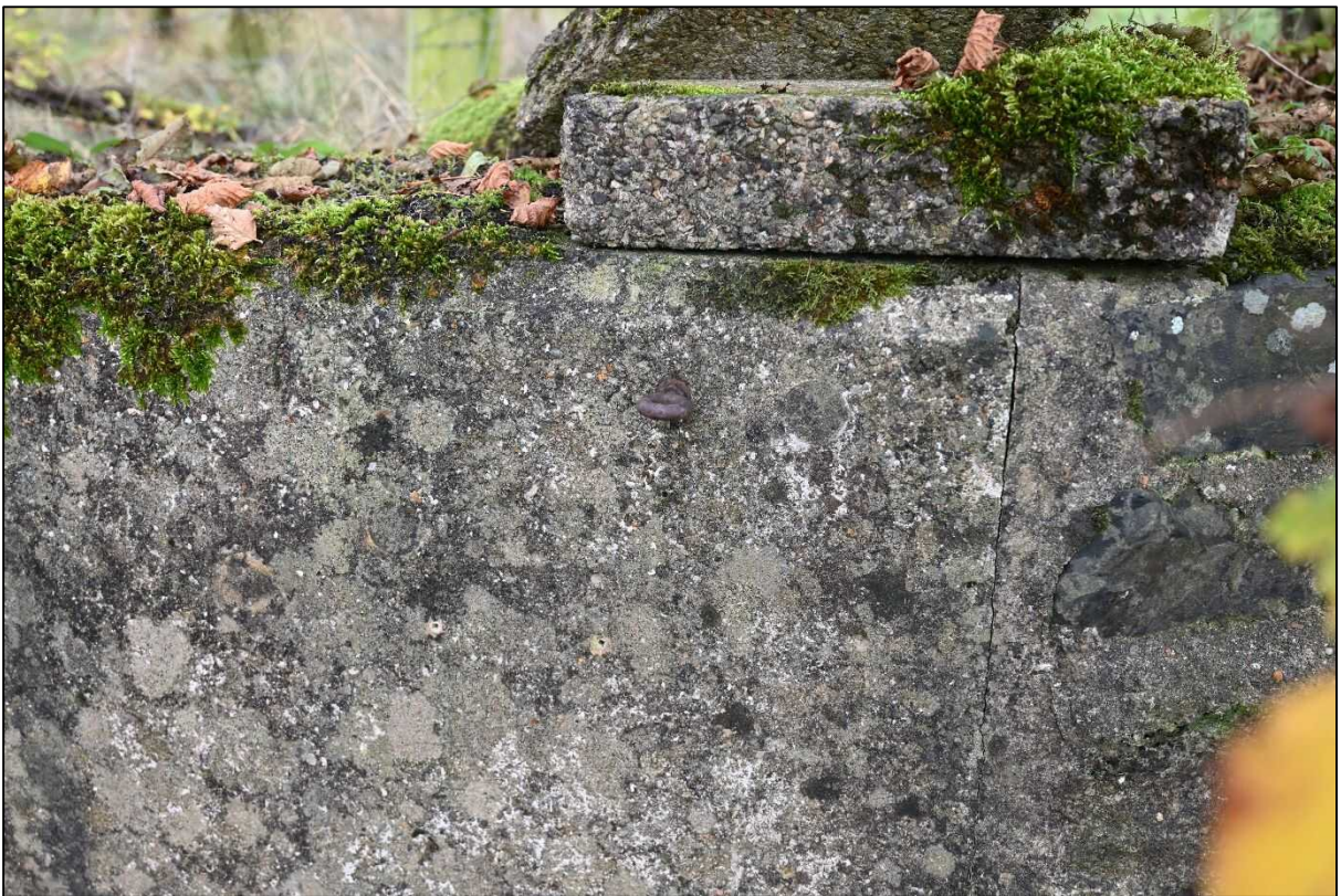
Plate 12: Eye bolt in the eastern end of the northern head wall
