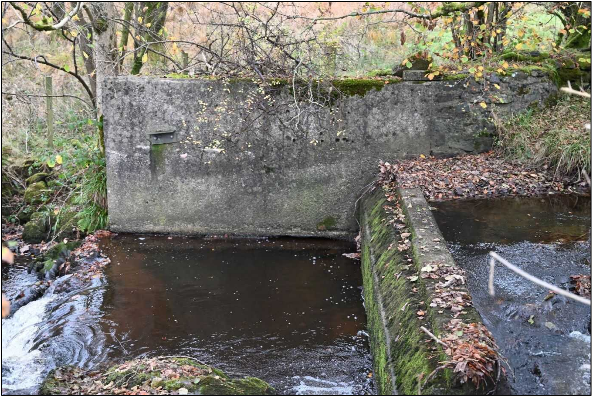
Plate 11: Northern concrete head wall
