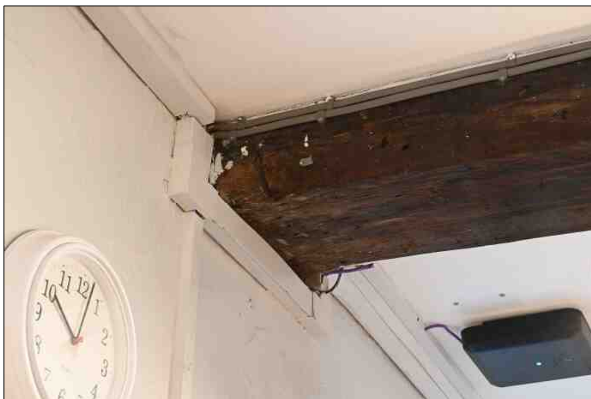
Plate 26: Chamfering and stop on the ceiling beam of the hall
