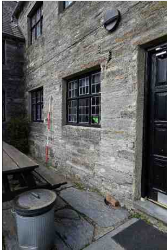
Plate 11: Partly blocked opening adjacent to the current front door
