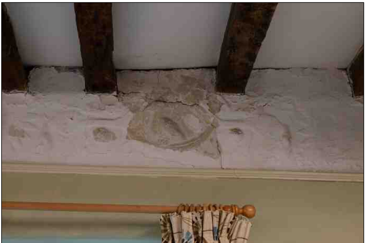
Plate 32: Area where the paint has flaked off showing the stonework of the frieze
