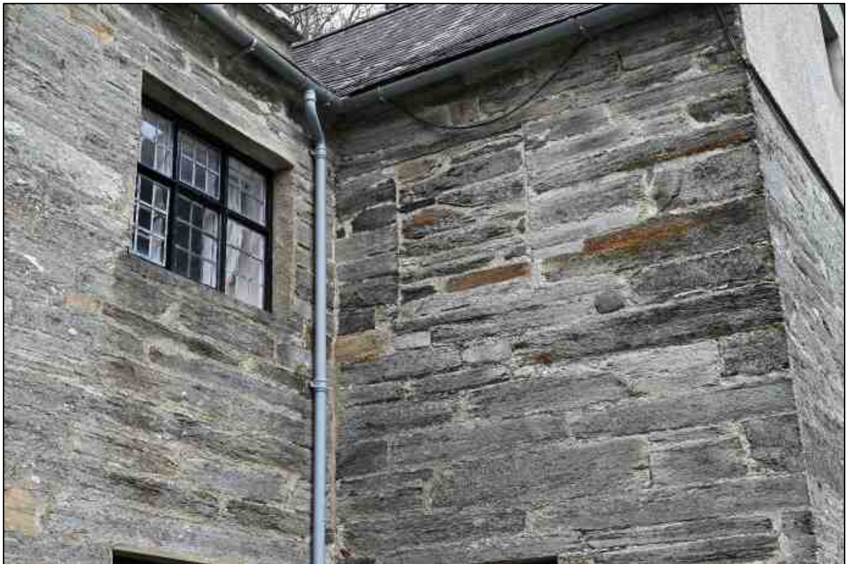
Plate 7: Blocked opening in the western face of the eastern range
