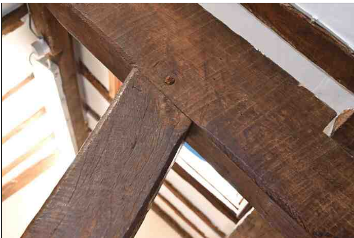
Plate 88: Carpenter's marks on the truss in the rear bedroom
