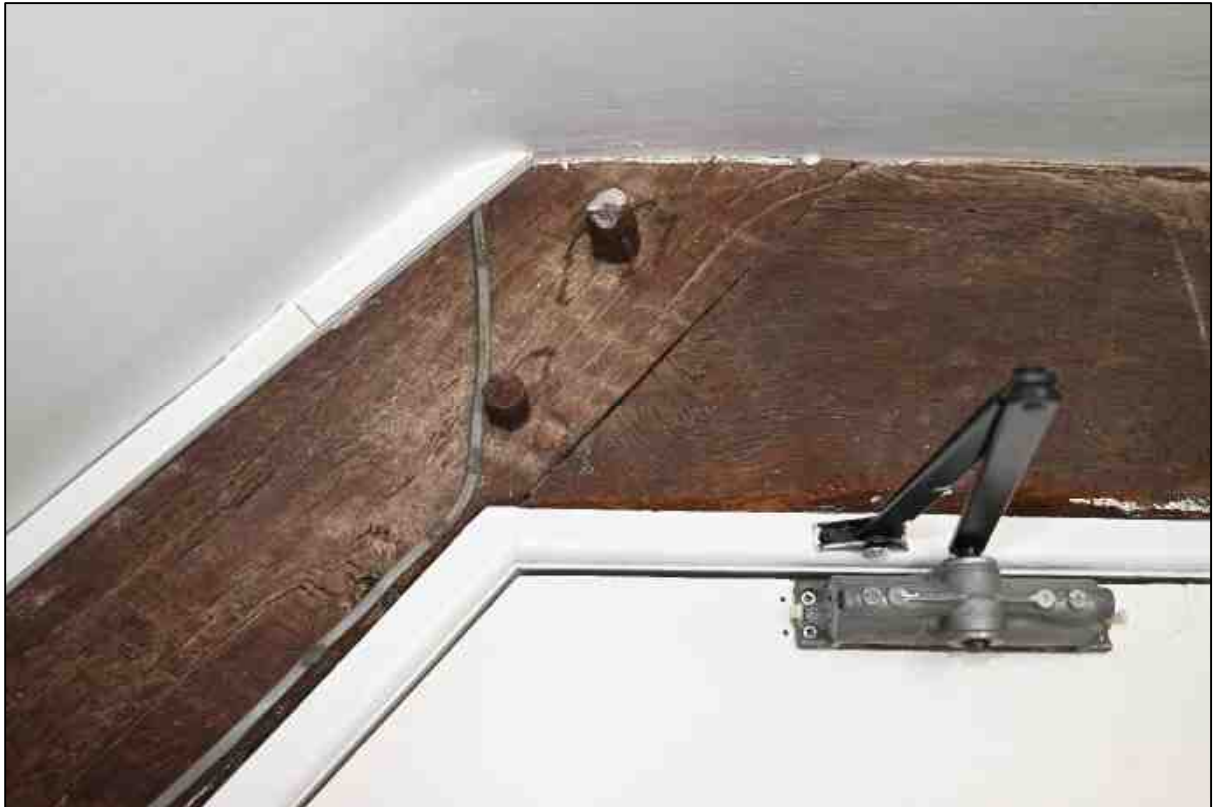
Plate 72: Detail of the joint between the collar and principal rafter of the truss in the northern room of the eastern range
