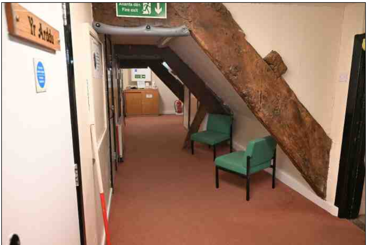
Plate 75: Trusses exposed in the corridor along the northern side of the central range
