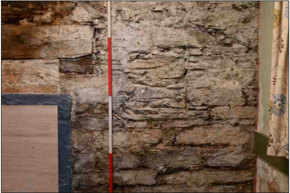
Plate 94: Blocked opening in the northern wall of the parlour
