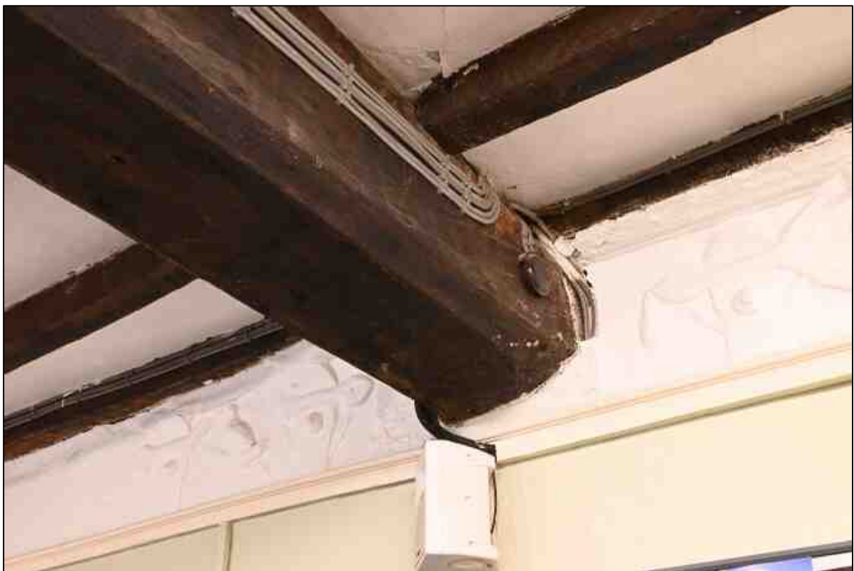
Plate 30: Chamfering and stop on the ceiling beam in the Parlour
