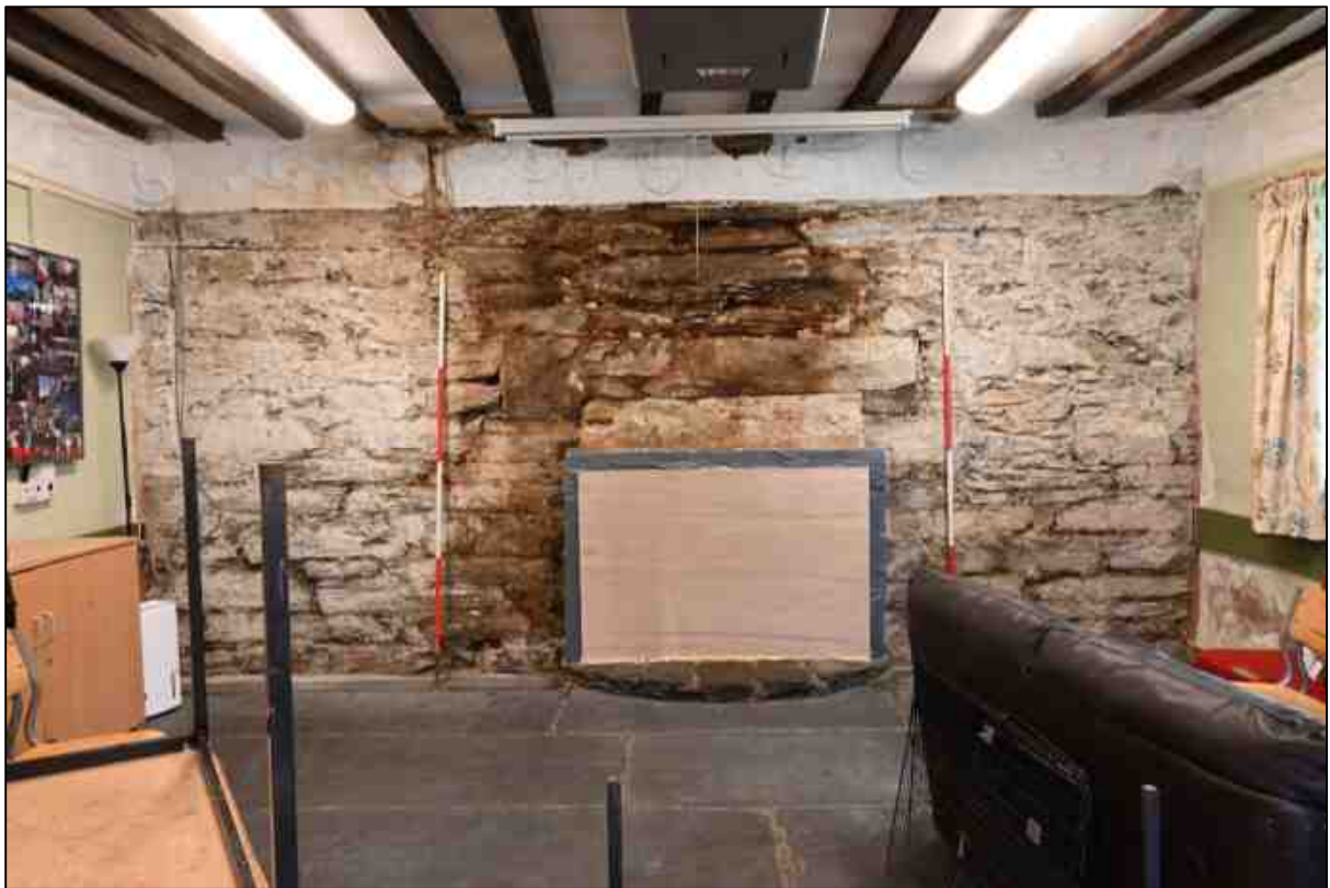
Plate 93: Parlour wall after the removal of the plasterboard sheets
