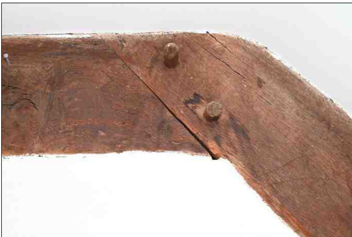
Plate 82: Detail of the joint between the collar and the principal rafter in the third bedroom on the second floor of the central range
