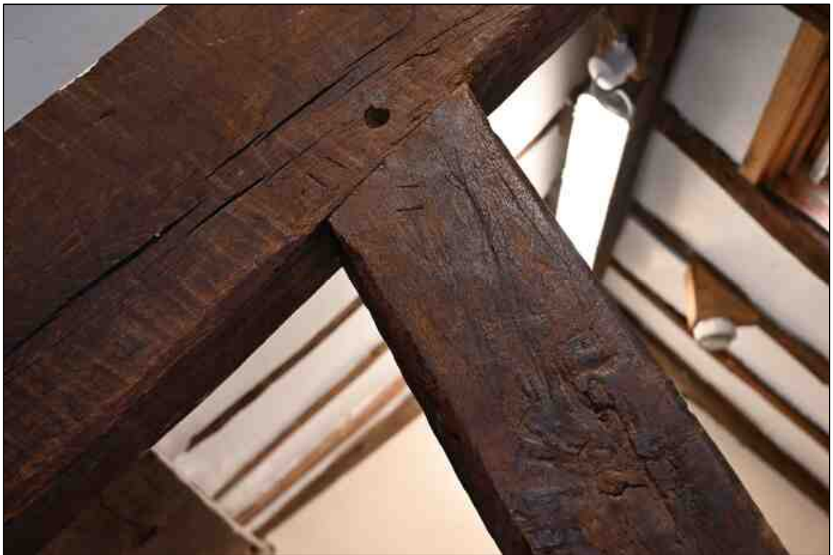
Plate 87: Carpenter's marks on the truss in the rear bedroom
