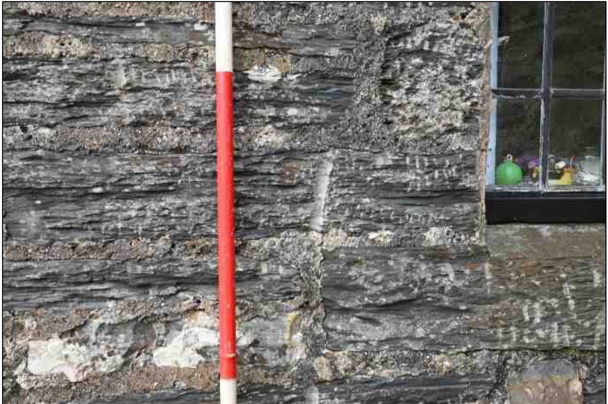
Plate 13: Drill casts on the eastern face of the western range
