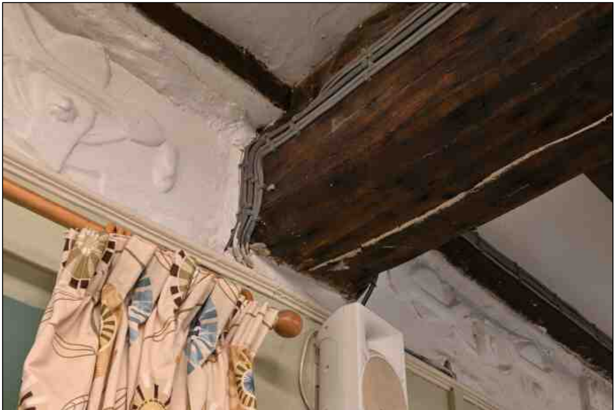
Plate 31: Chamfering and stop on the ceiling beam in the Parlour
