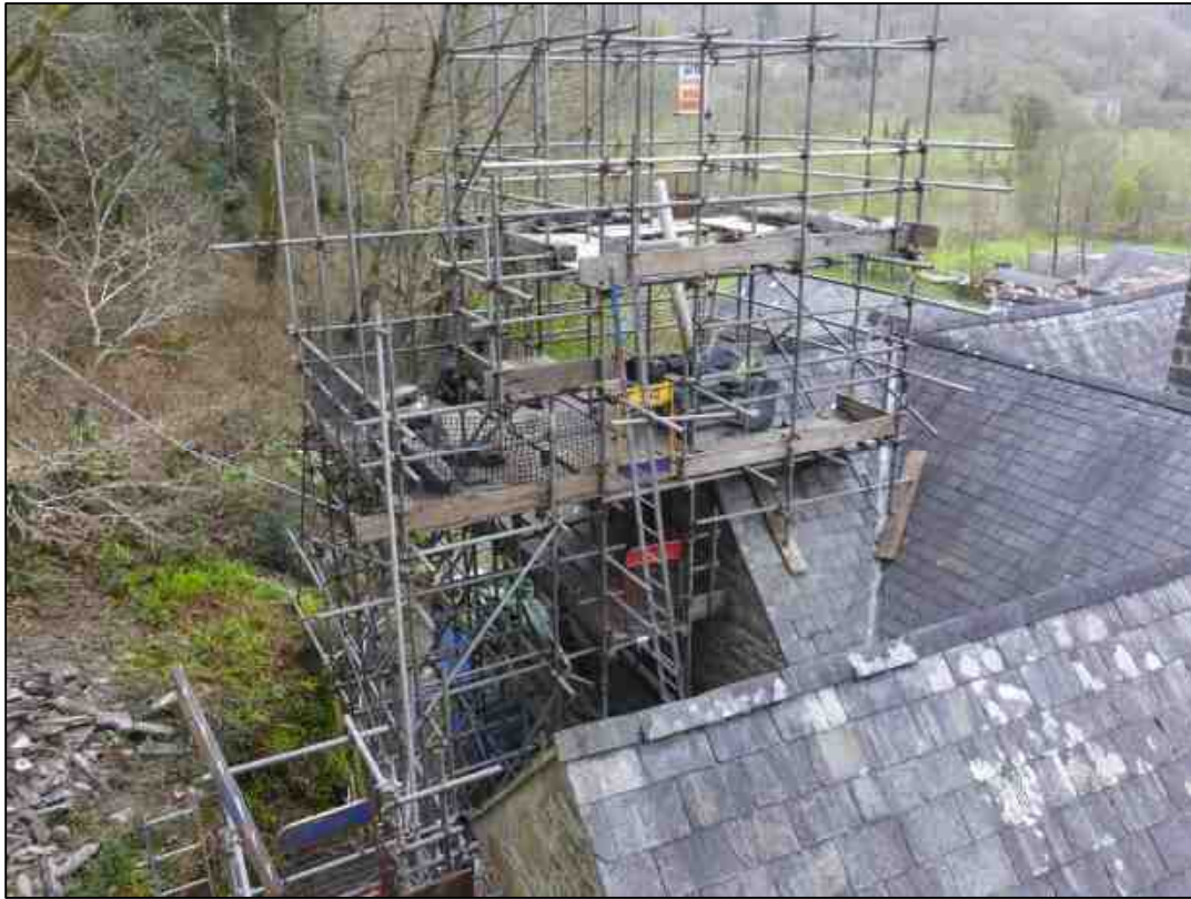
Plate 92: Chimney over the eastern range under demolition
