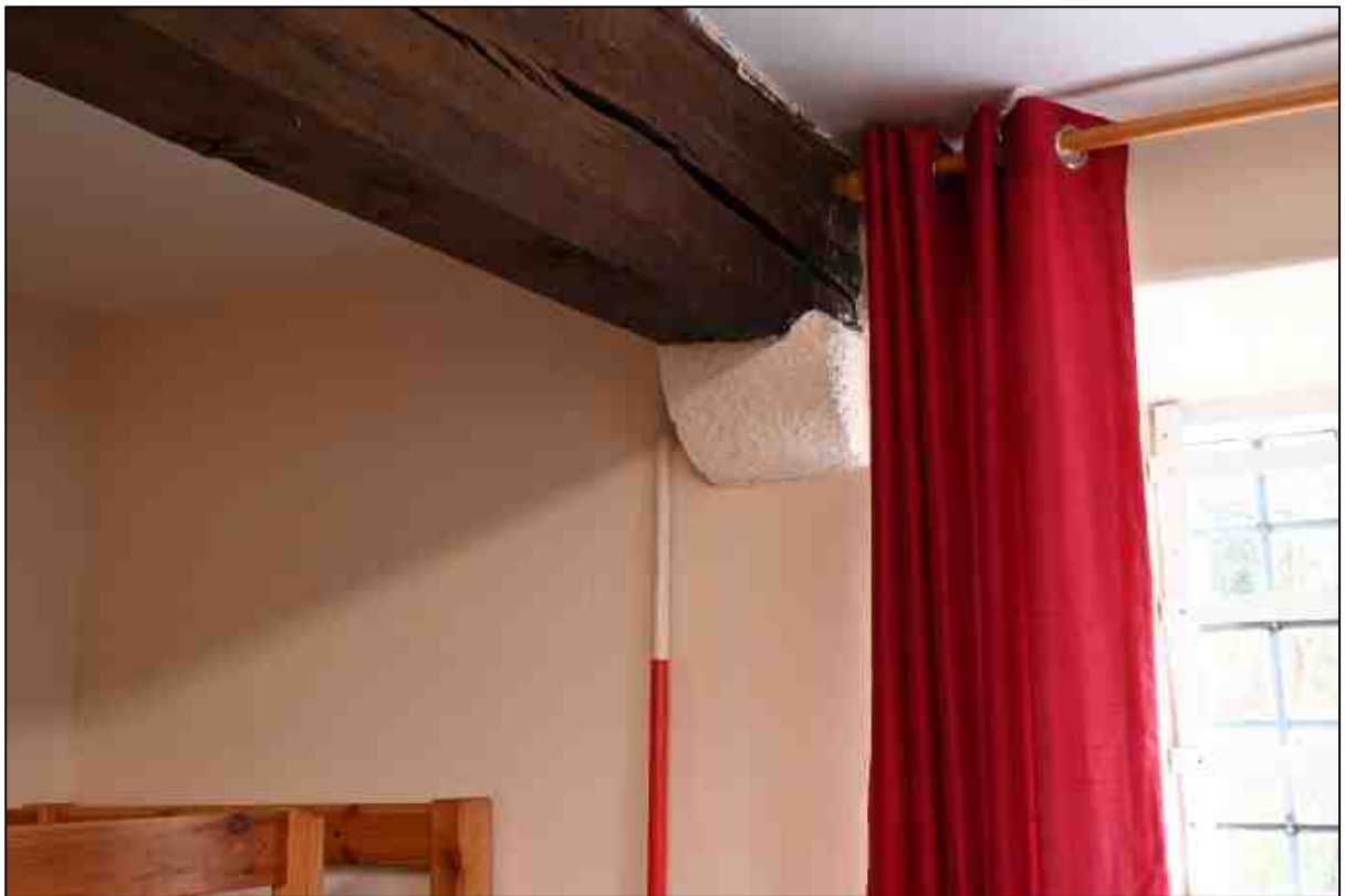
Plate 49: Corbel holding the main ceiling beams in the southern, first floor, bedroom of the eastern range
