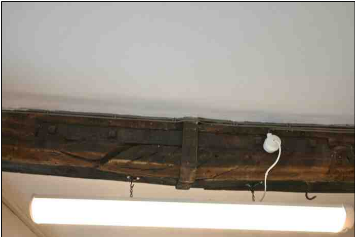
Plate 27: Repair to the ceiling beam in the Hall
