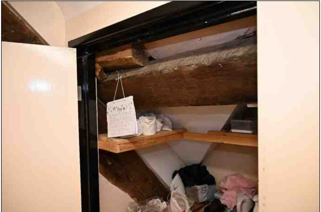
Plate 73: Purlin and principal rafter in the cleaning cupboard
