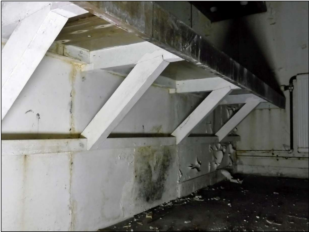
Plate 25: Supports for the bench of the vanity units
