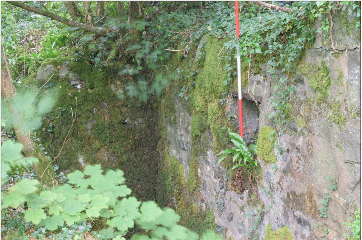
Plate 13: Hole for the wheel shaft in the wheel pit of the eastern "Pandy" Building
