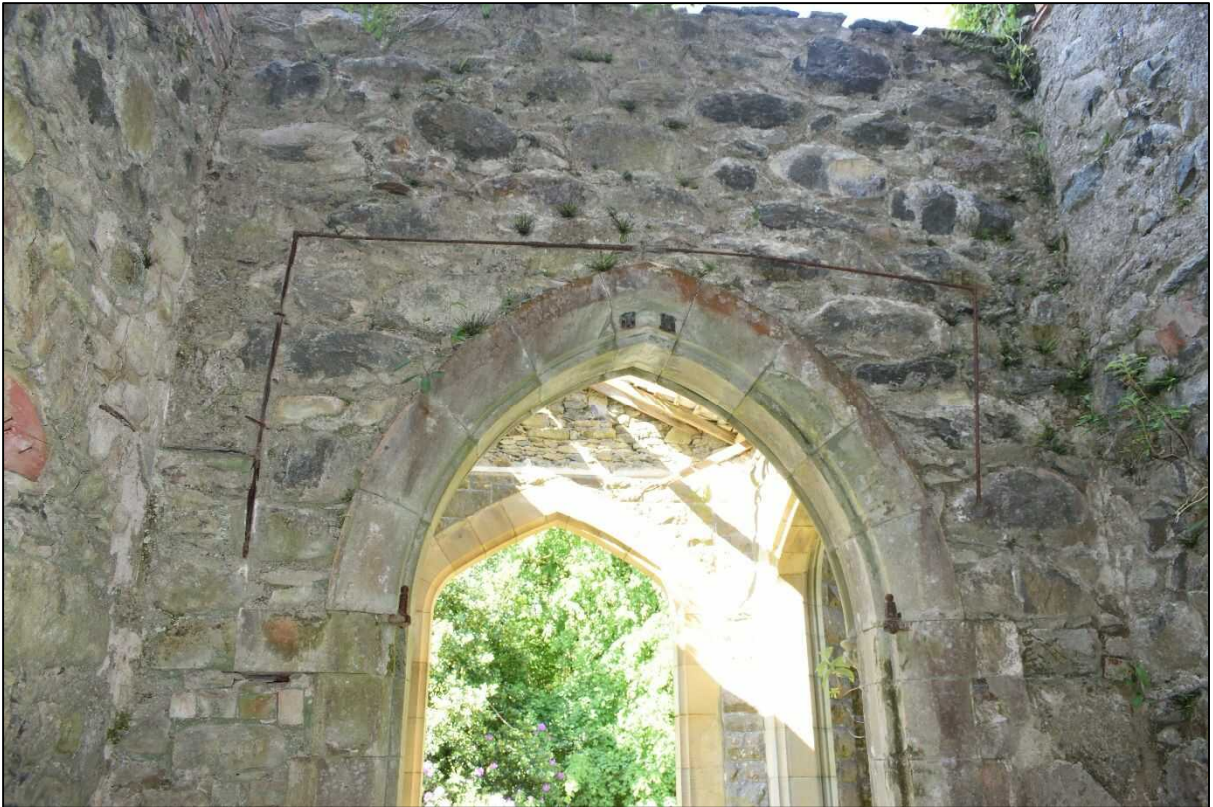
Plate 31: Remains of the bell pull system inside the main door
