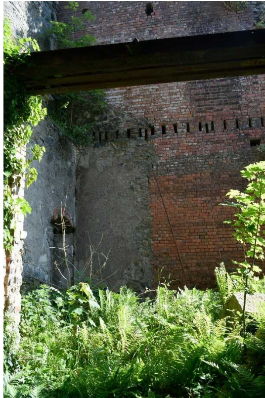
Plate 41: Relationship between a stone and brick wall towards the north eastern end of the main range
