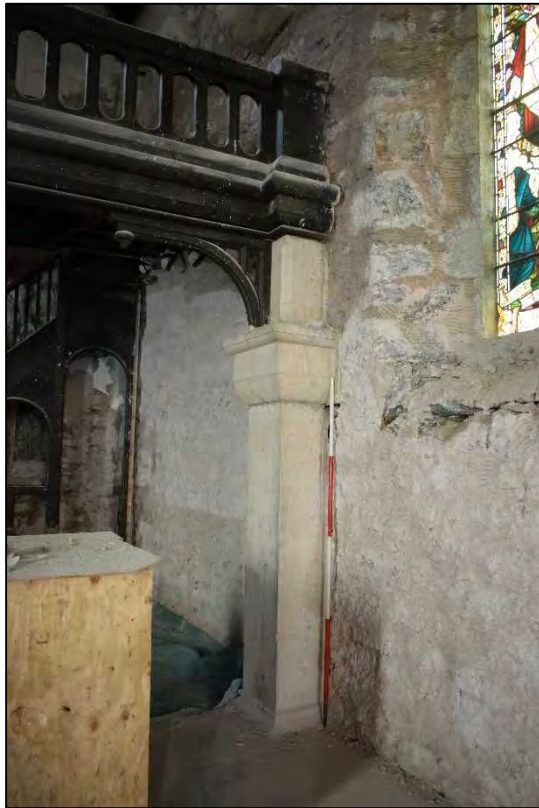
Plate 38: The northern pilaster supporting the gallery
