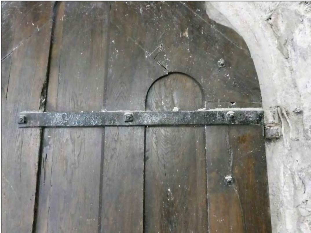
Plate 35: Detail of the inner hinge
