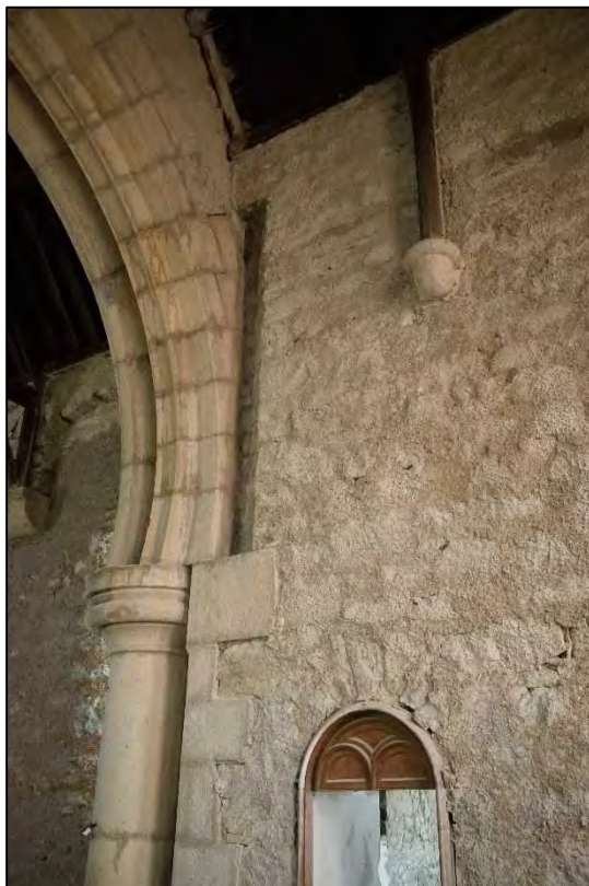
Plate 60: The relationship between the chancel arch and the chancel wall
