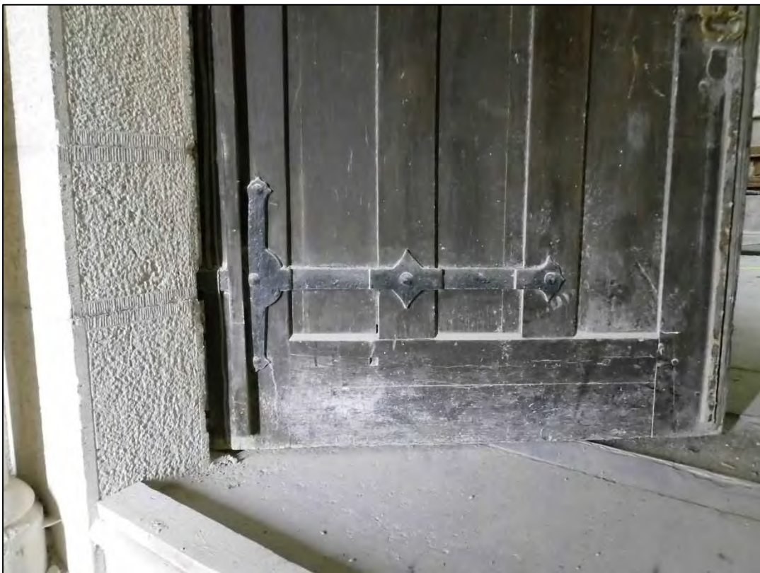
Plate 30: Detail of the outer mock hinge
