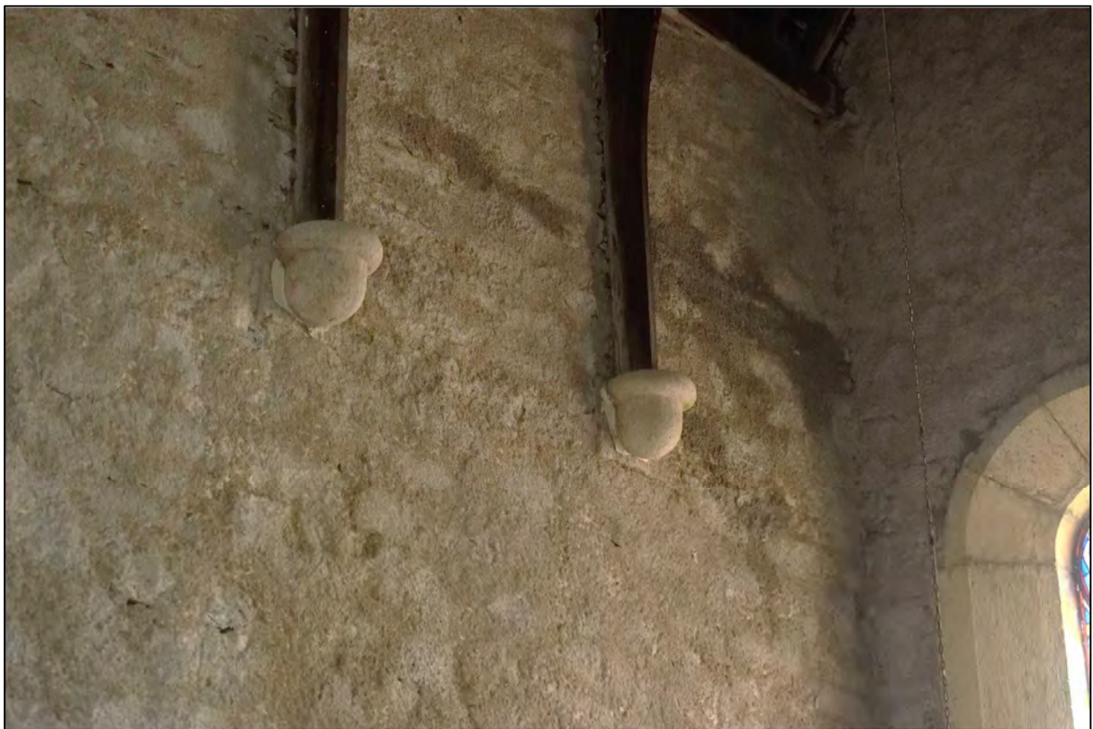
Plate 68: The corbels supporting the chancel roof
