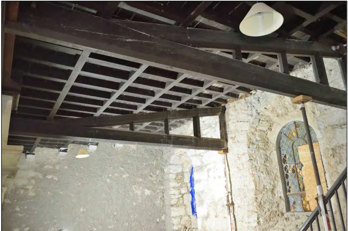
Plate 41: Brackets supporting the gallery
