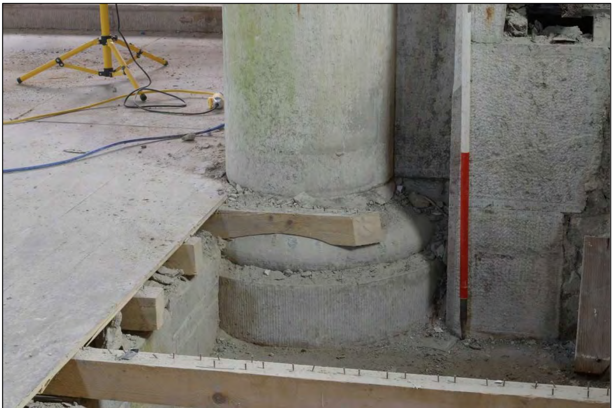
Plate 58: Base of the chancel arch hidden below the current floor
