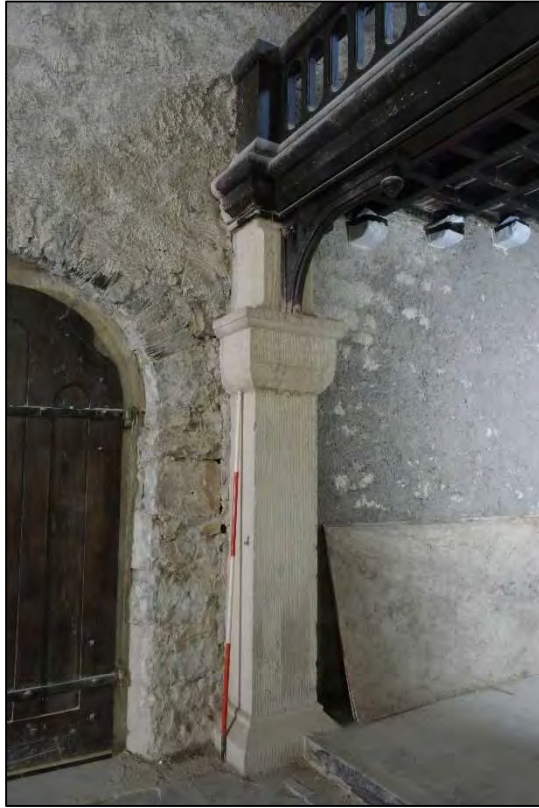
Plate 37: Southern pilaster supporting the gallery
