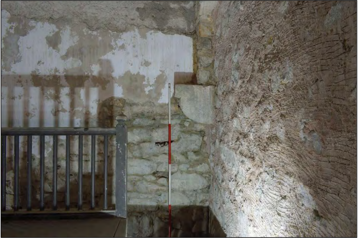
Plate 49: Corbel supporting the arcading on the north wall
