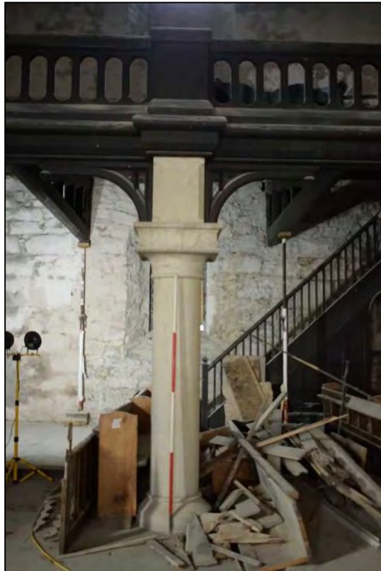
Plate 39: Central column supporting the gallery
