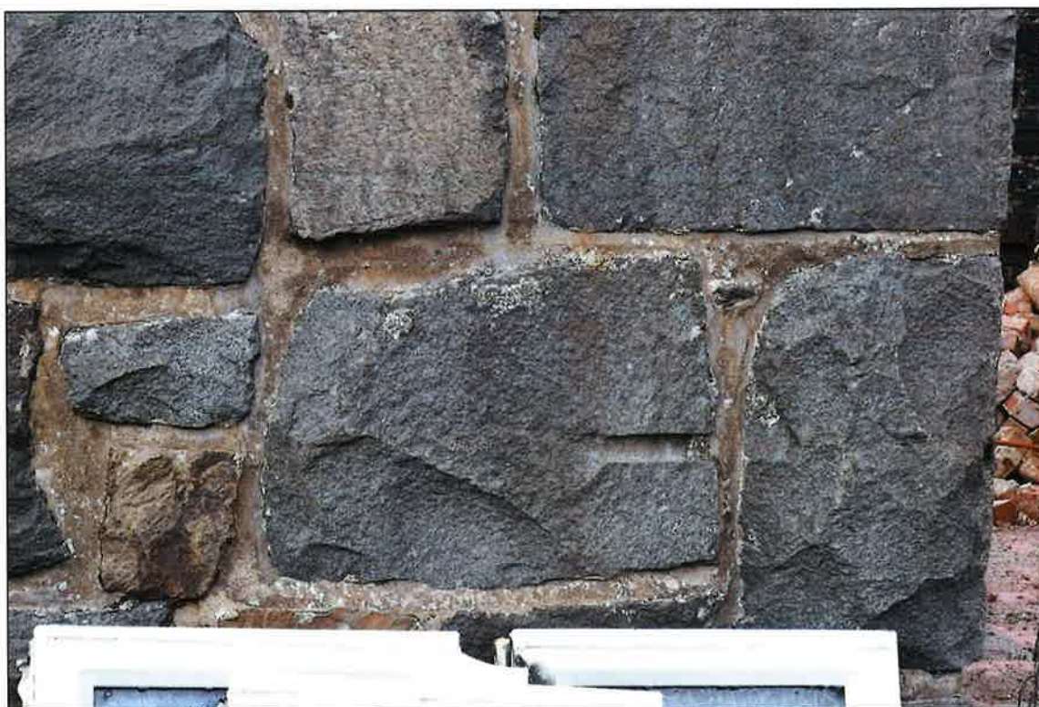
Plate 14: Remains of a drill hole in one of the blocks of the southern elevation of Range 5.
