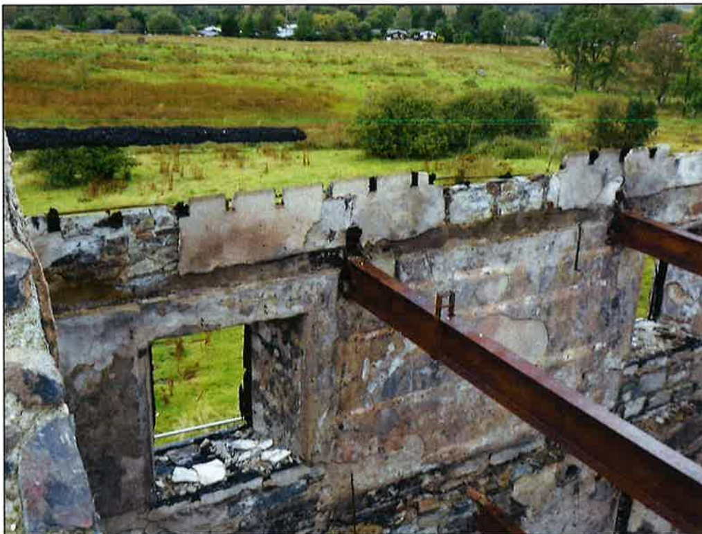
Plate 46: Upper joists within Range 1, showing the position of the trusses.
