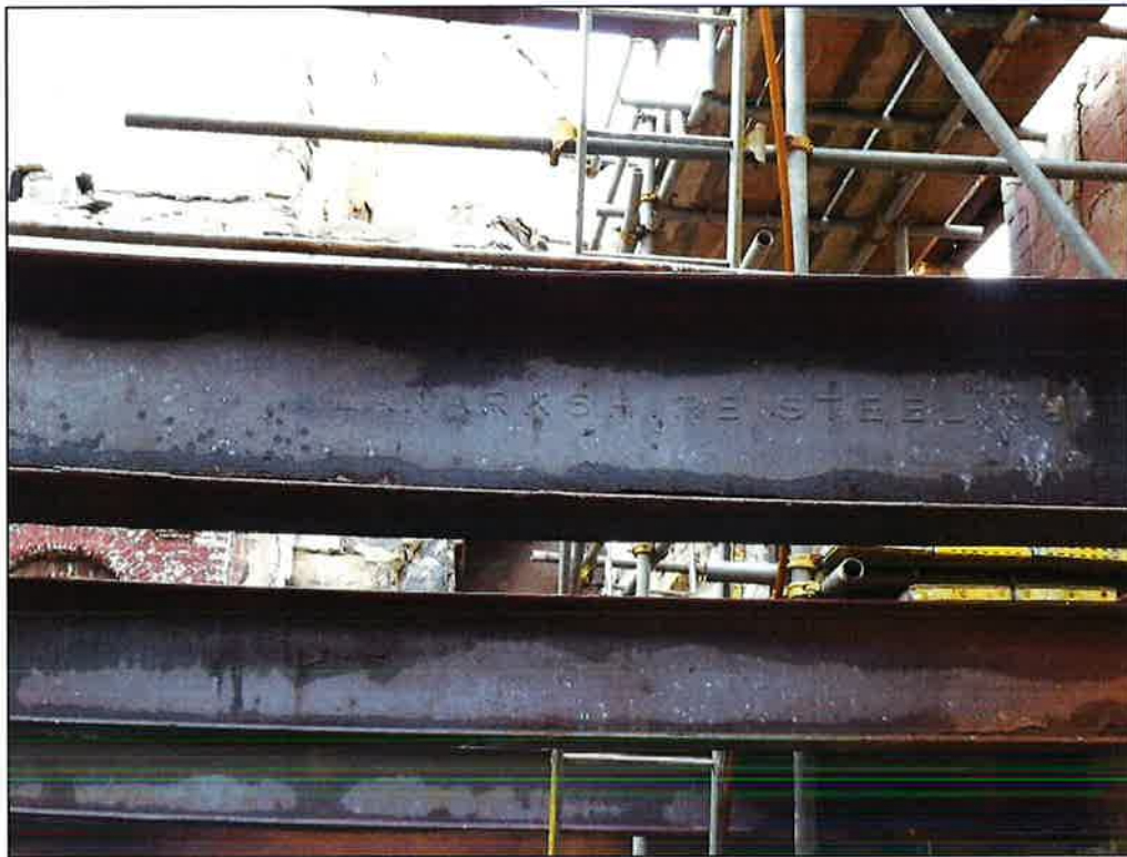
Plate 45: Rolled steel joist in Range 1
