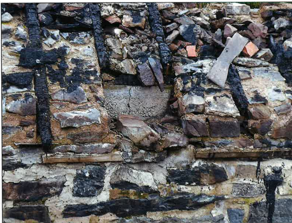
Plate 26: Concrete beam on top of the southern wall of Range 3
