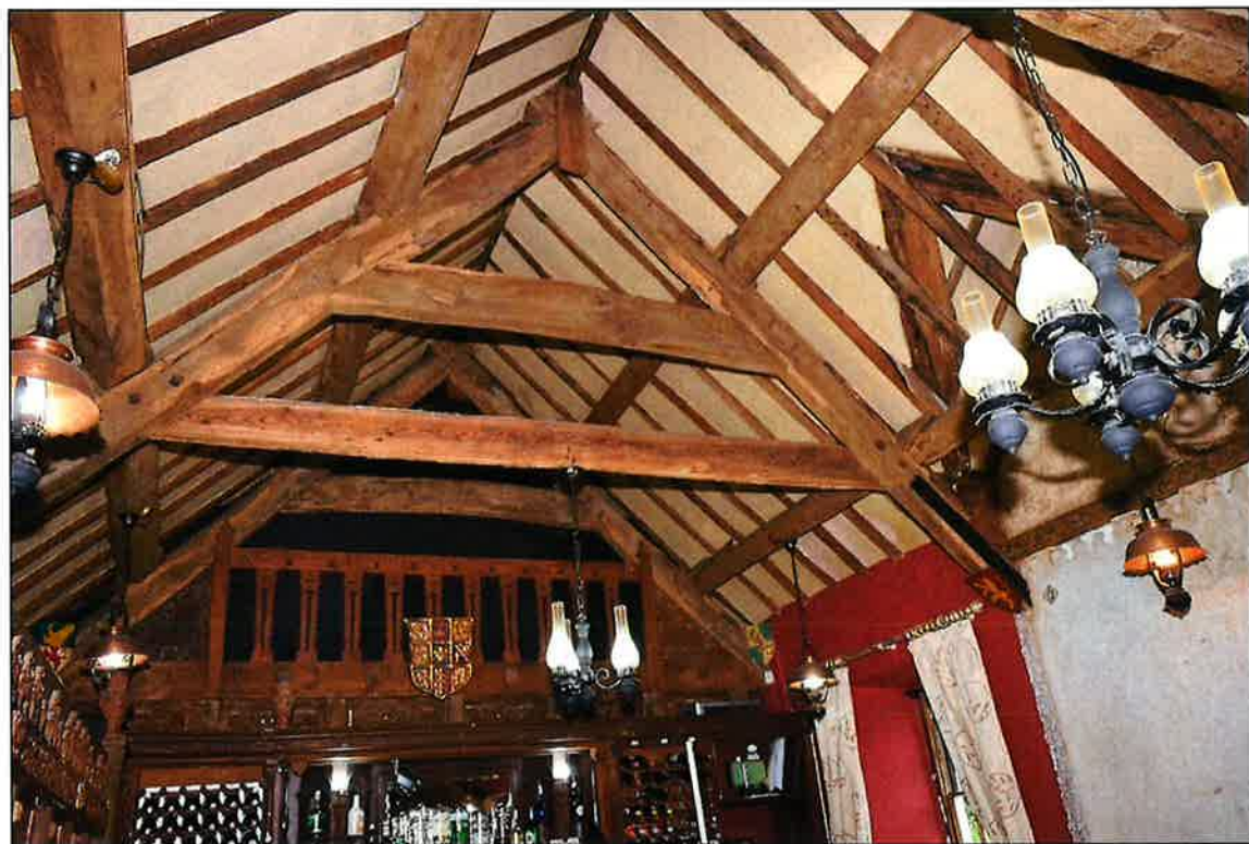
Plate 38: Truss 3, looking west
