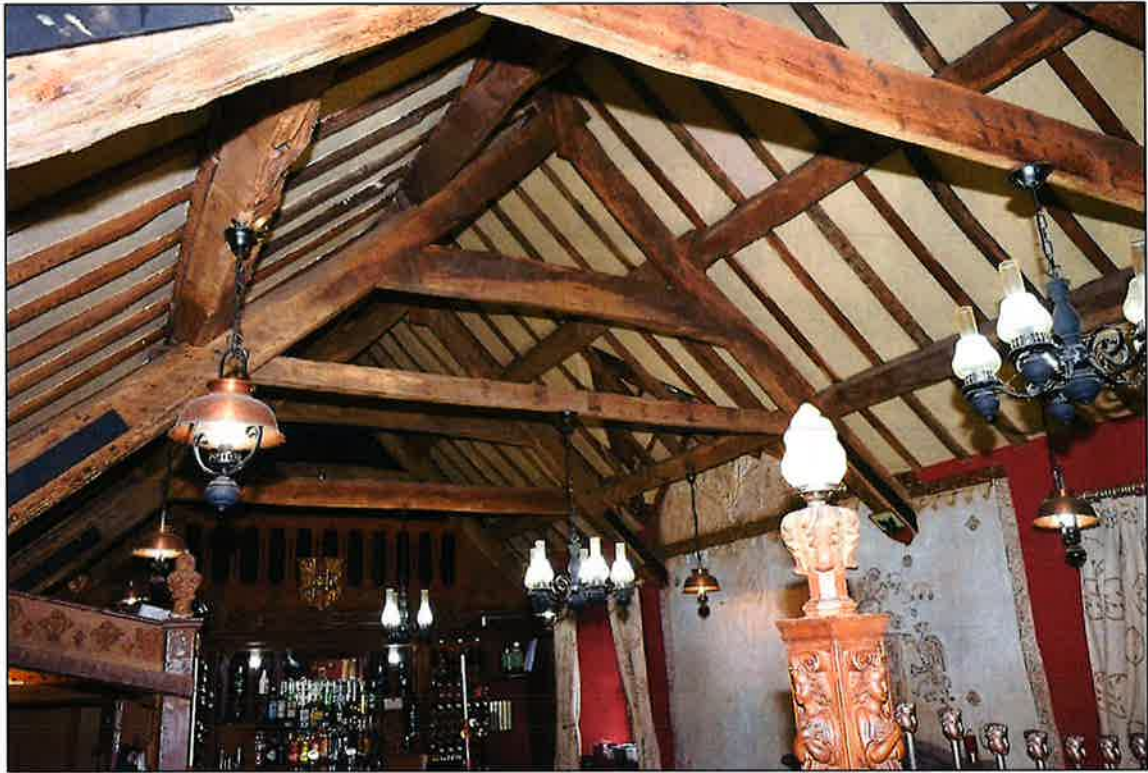
Plate 37: Truss 2, looking west
