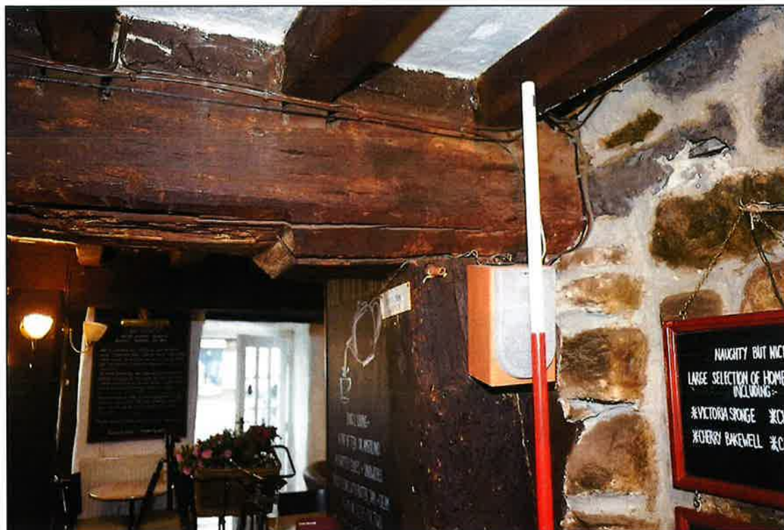
Plate 22: Chamfer on one of the ceiling beams
