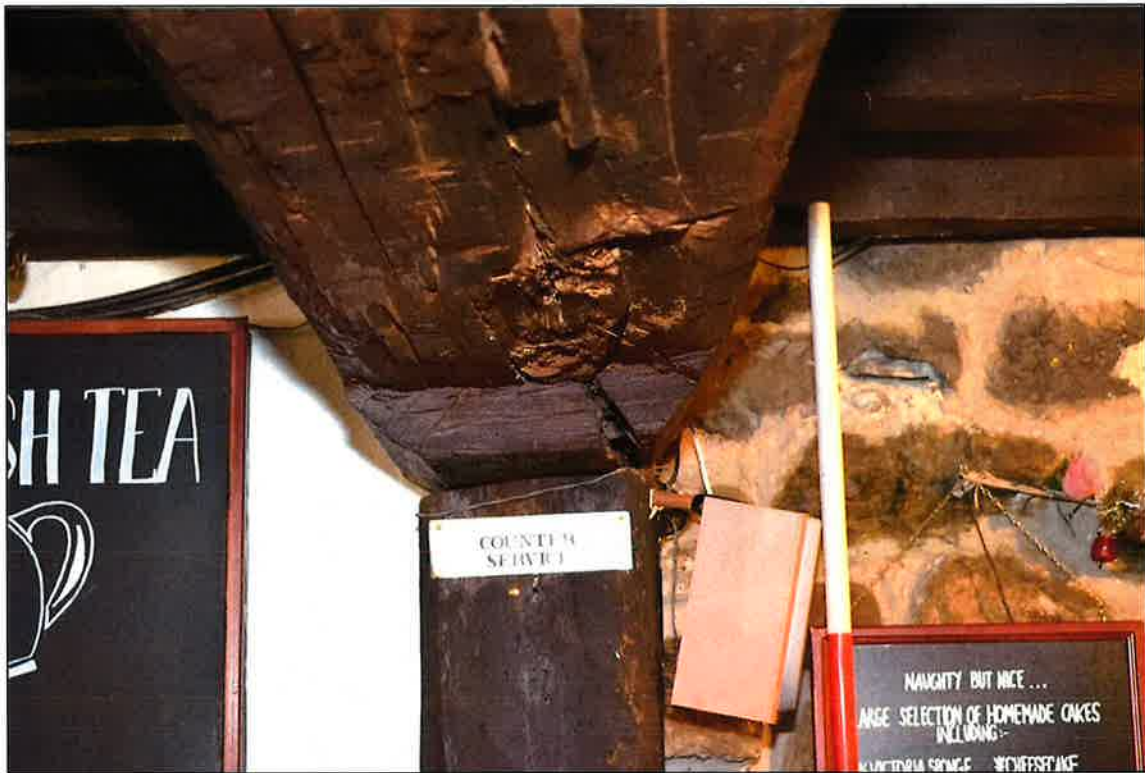
Plate 21: Underside of one of the ceiling beams in the tearoom, showing the thinning
