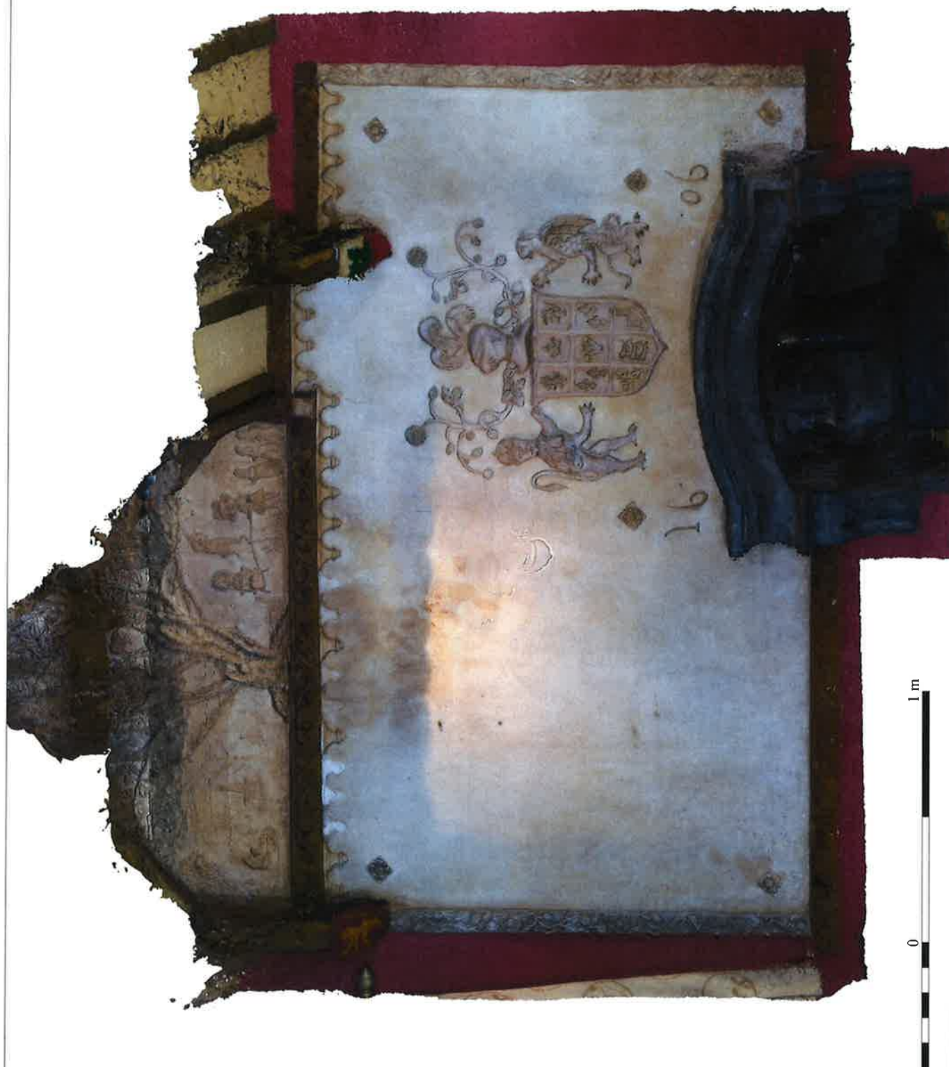
Figure 20: Photogrammetric Image of the Plasterwork Scale 1:20
