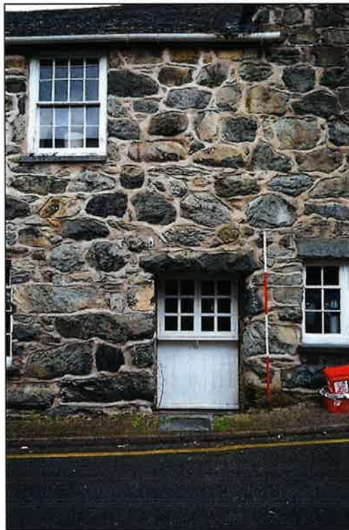
Plate 17: Partially blocked doorway and window above
