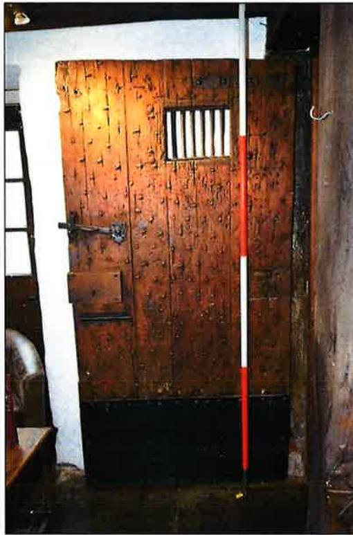
Plate 29: Door at the base of the staircase
