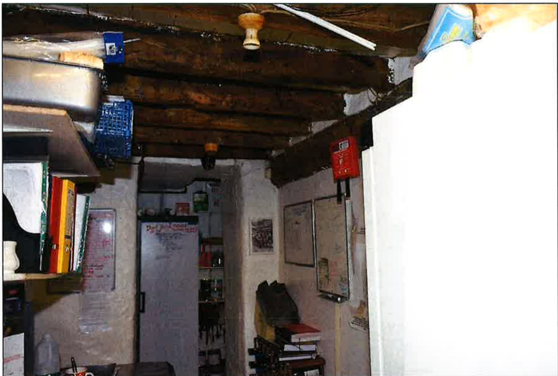
Plate 30: Passageway, looking south
