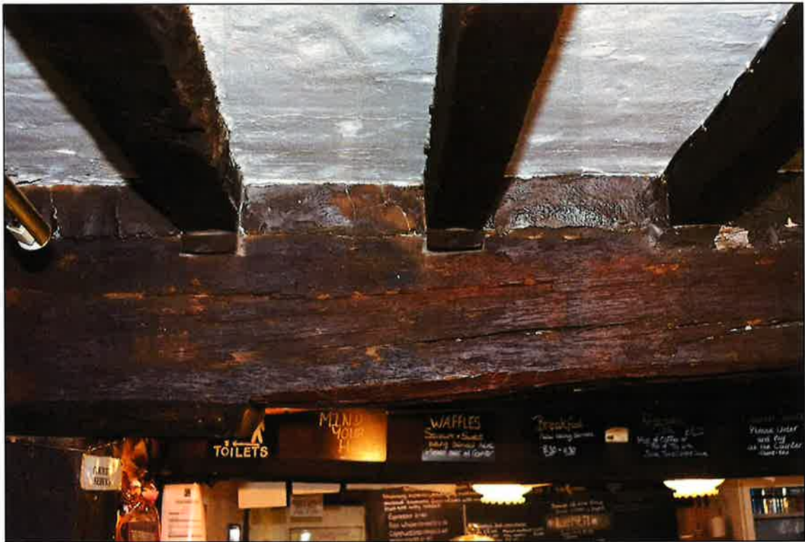
Plate 25: Cogged joists
