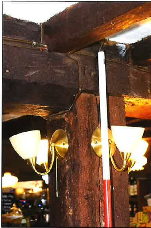
Plate 23: Chamfer on one of the ceiling beams
