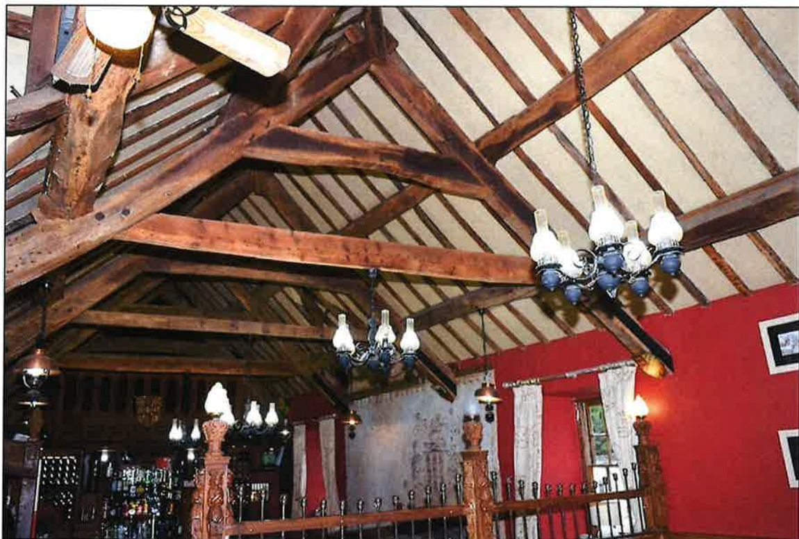
Plate 36: Truss 1, looking west
