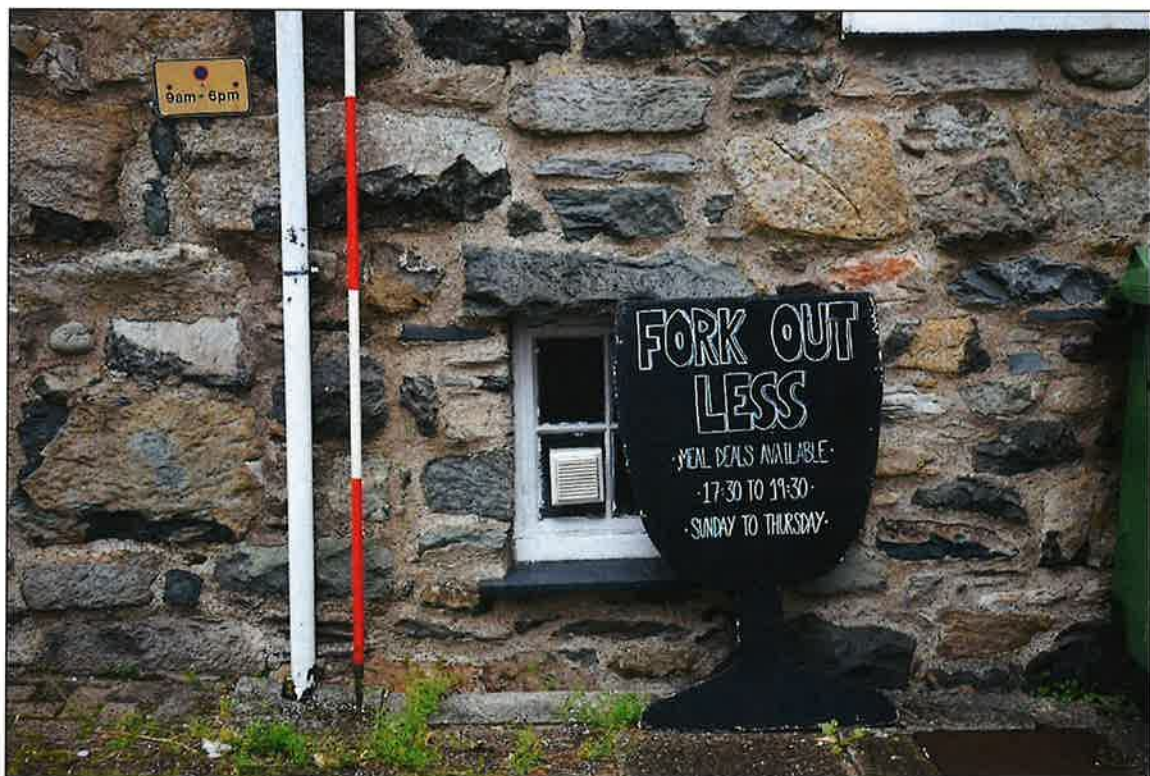
Plate 8: Ground floor window in the southern elevation
