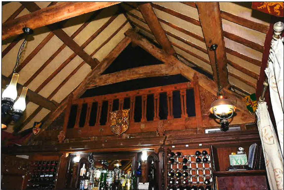
Plate 39: Truss 4, looking south west
