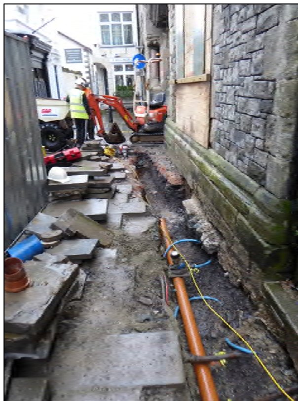
Plate 5: The new sewer trench during construction
