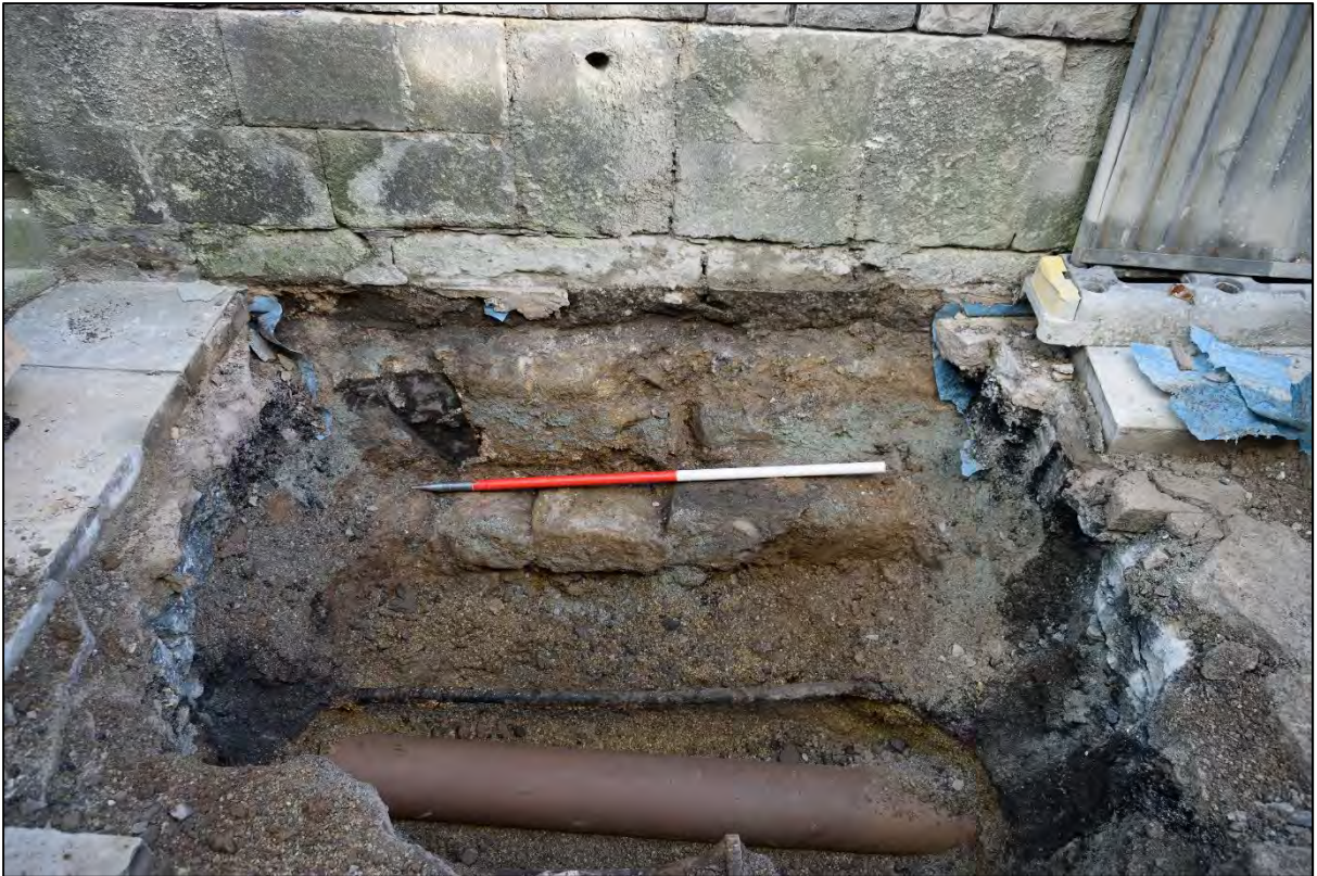
Plate 6: Footing of 3 Hole in the Wall Street in new sewer trench
