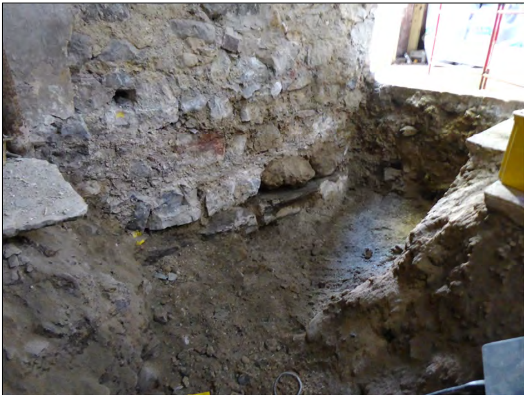
Plate 2: Footings of western wall of 3 Hole in the Wall Street
