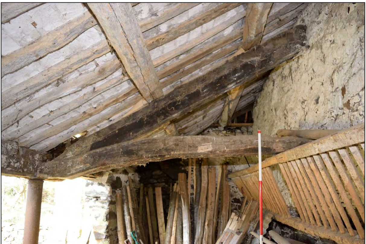
Plate 8: Truss in the byre, looking north
