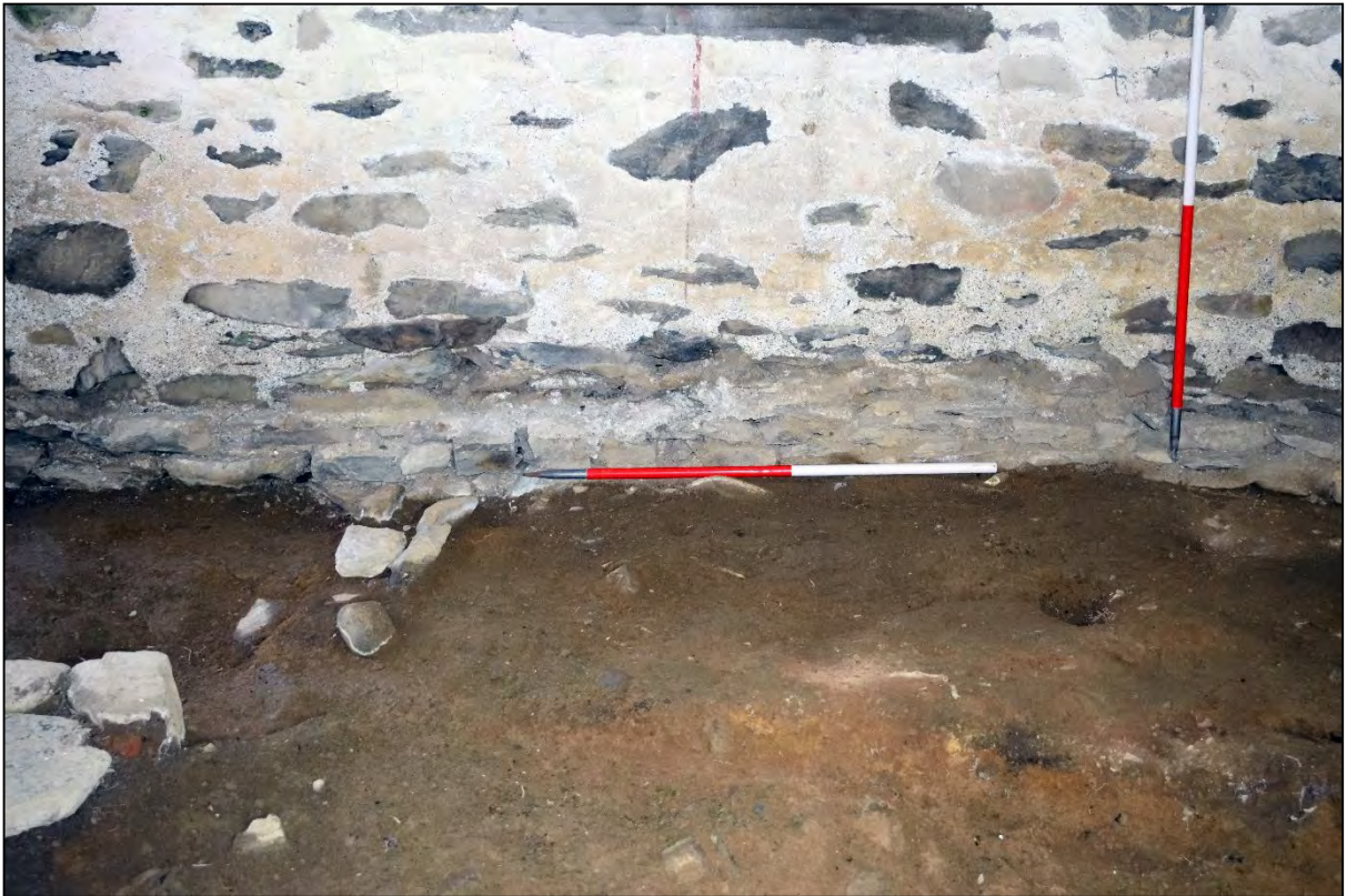
Plate 30: Drain, Context 10 and footings of the western gable wall
