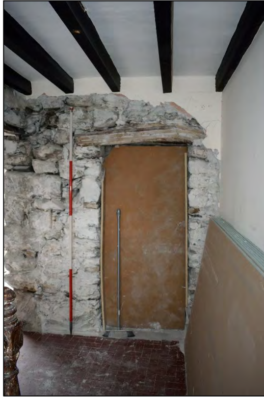
Plate 7: Blocked doorway in the rear elevation (internal)
