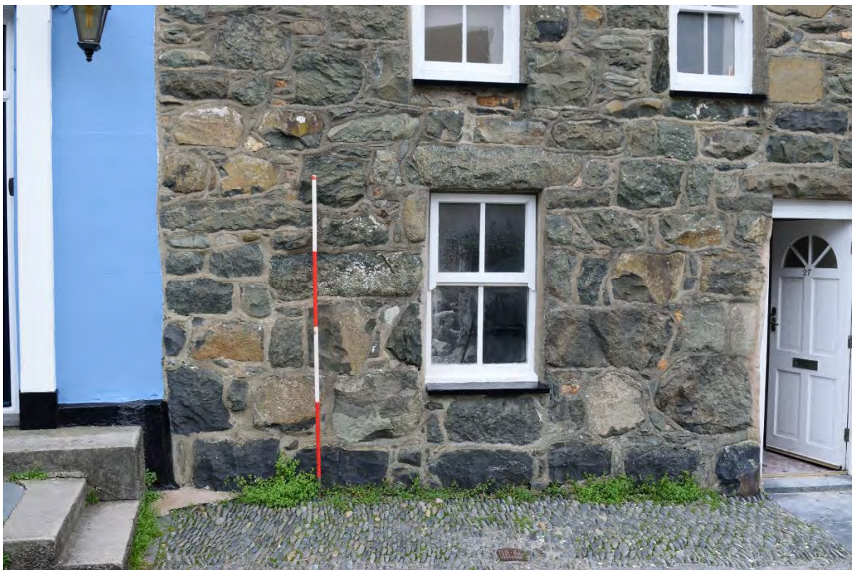
Plate 6: Partly blocked doorway and blocked widow in the front elevation
