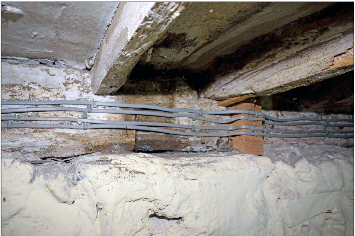
Plate 26: Joint on the western side of the beam in the cellars
