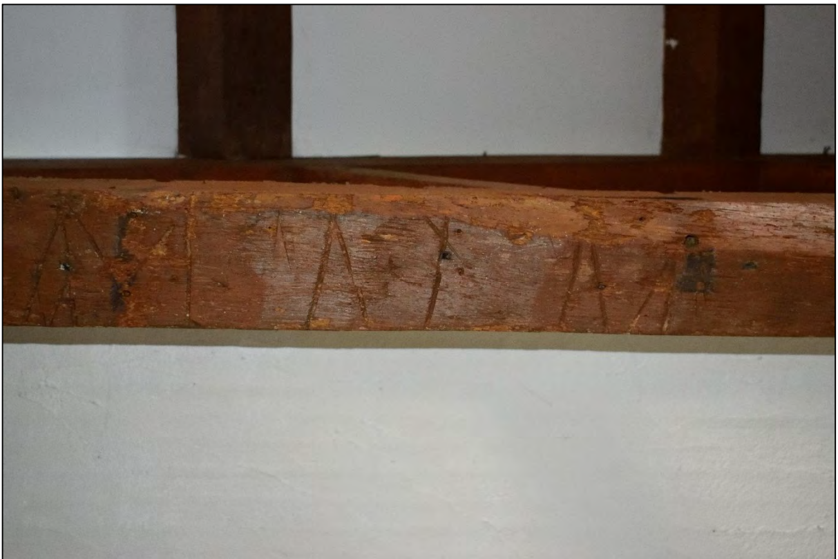
Plate 50: Marks in the underside of the half truss collar in Room 7
