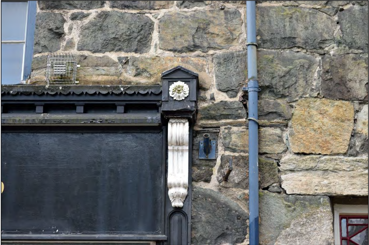
Plate 3: Detail of the console and pedimented cap.
