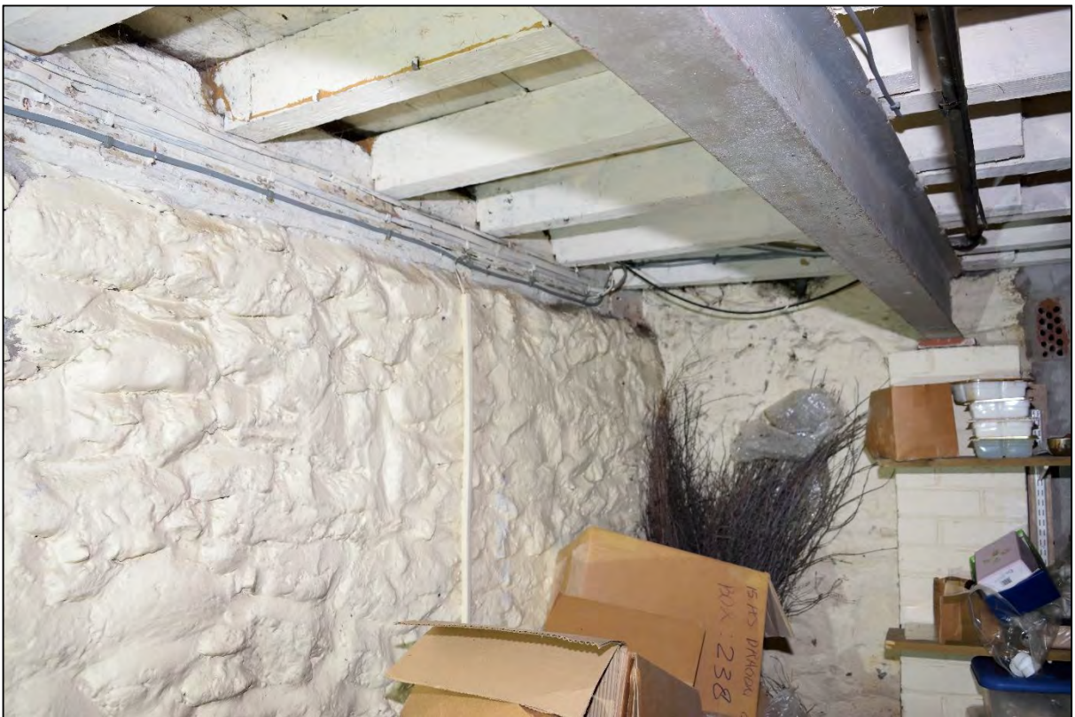
Plate 24: Wooden beam capping the wall between Cellar 4 and Cellars 2 and 3
