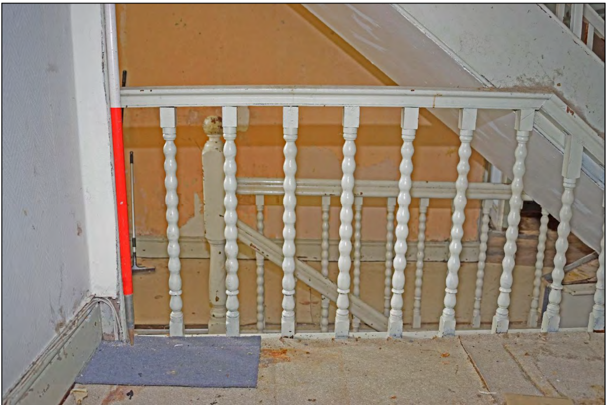
Plate 36: Turned balusters between the ground and first floor
