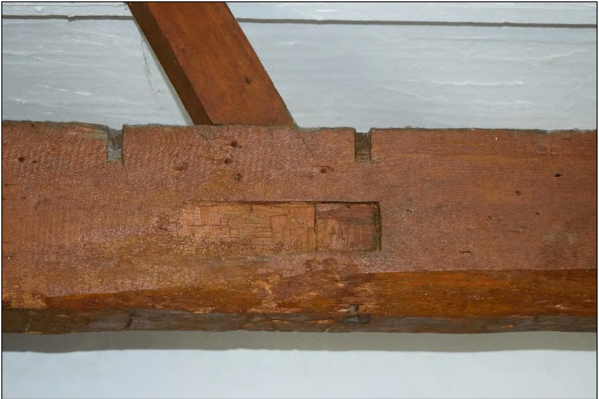
Plate 47: Socket for a partition on the truss in Room 7
