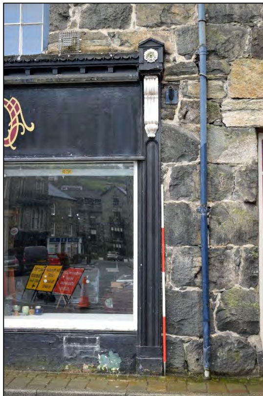
Plate 2: Detail of pilaster defining the shop window
