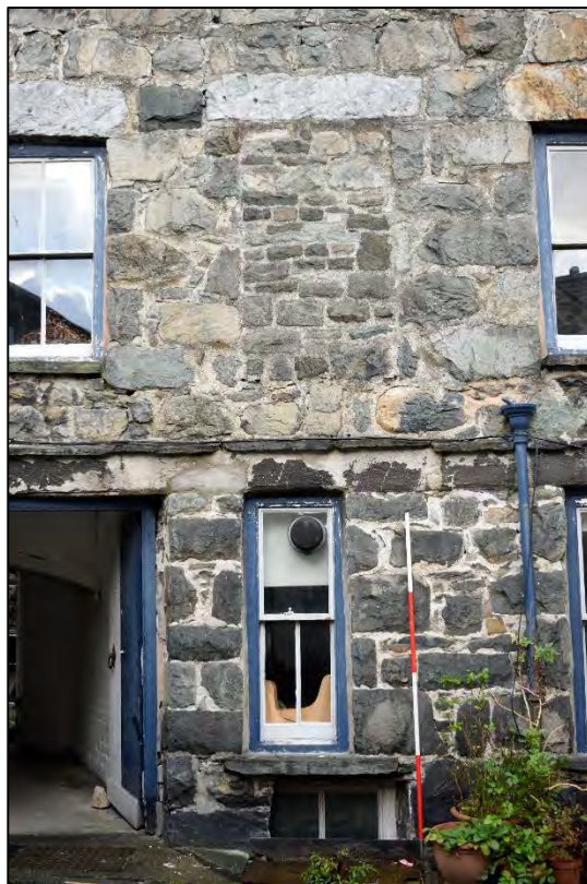
Plate 10: Blocked window in the rear range
