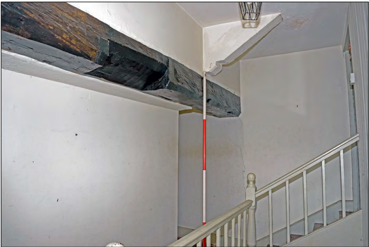
Plate 52: Foot of truss resting on main beam over the stairwell.
