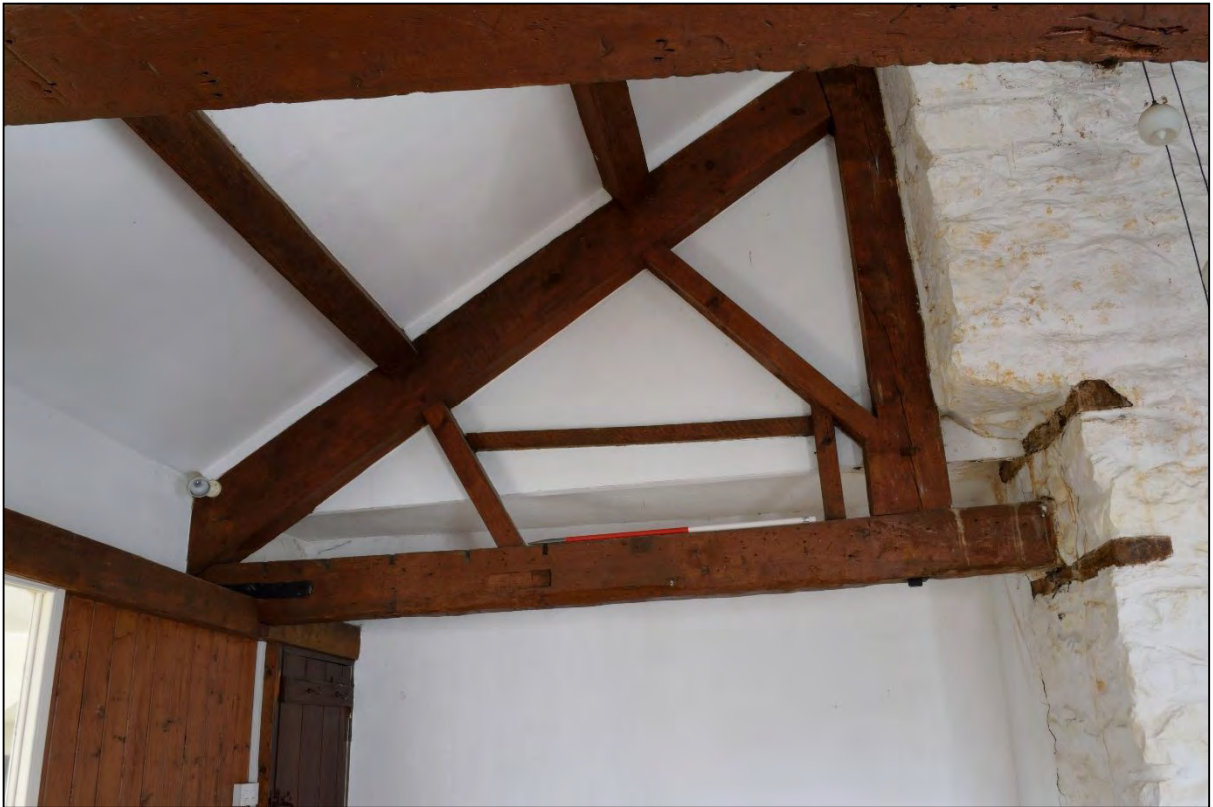
Plate 49: Half truss in Room 7
