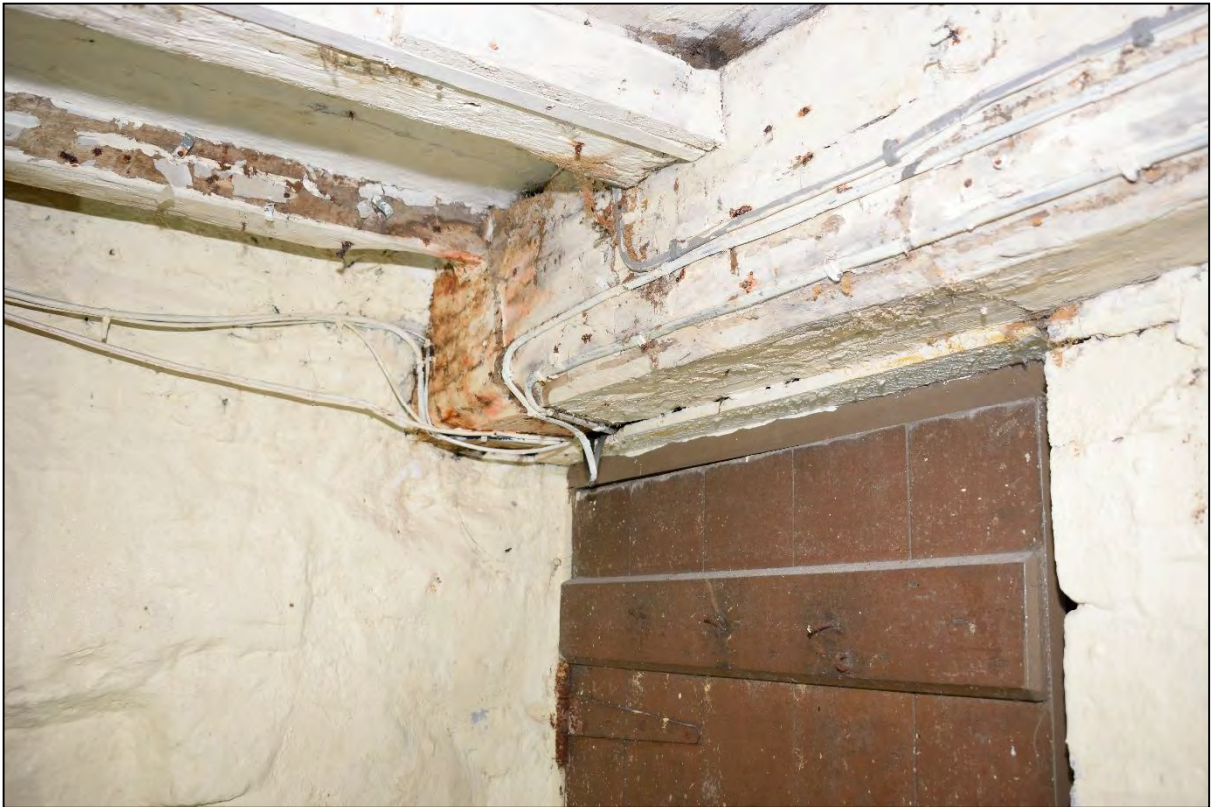
Plate 25: Detail of chamfer and stop
