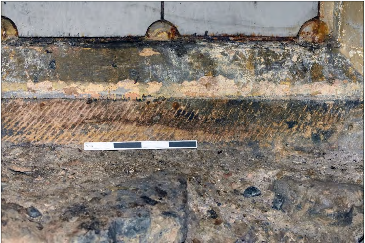
Plate 59: Circular saw marks on the lintel of the double window in the north gatehouse
