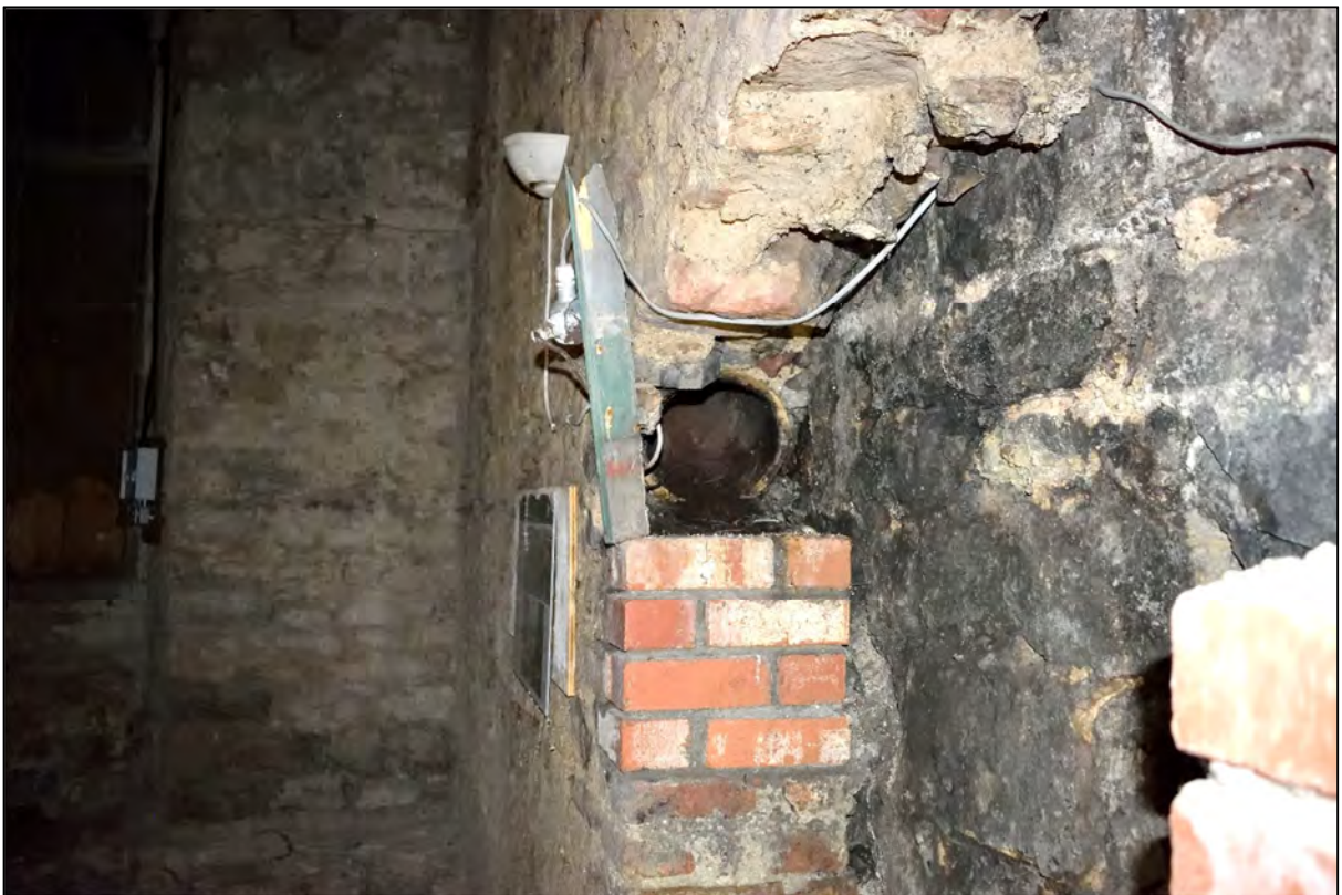
Plate 66: Flue in the side of the fireplace
