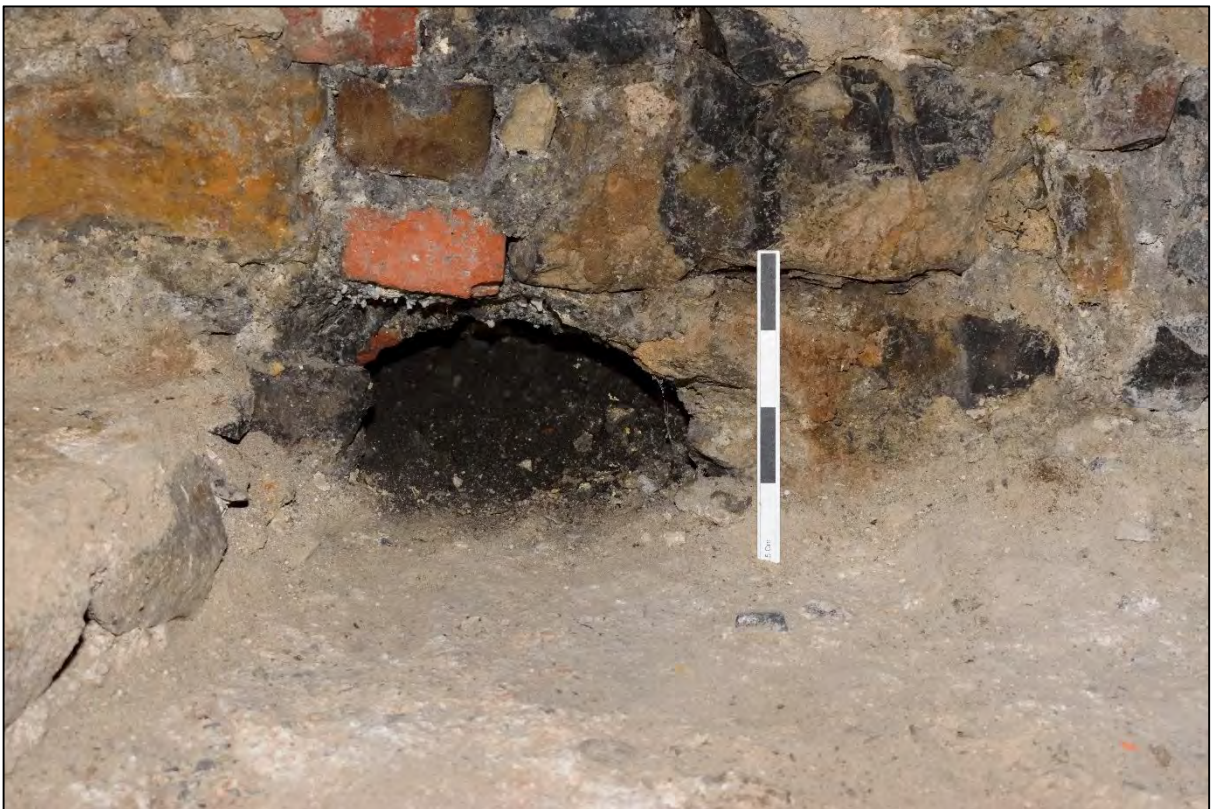
Plate 82: Hole for a service pipe below the western wall
