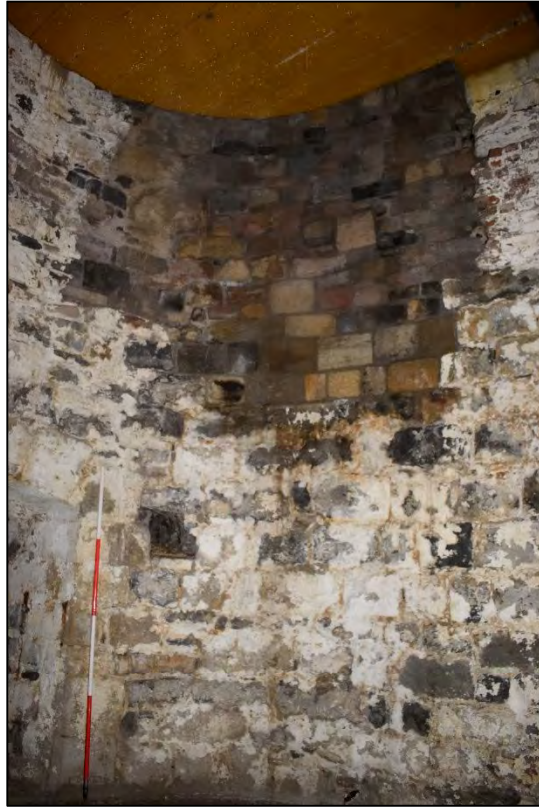
Plate 39: Repair to the southern gatehouse
