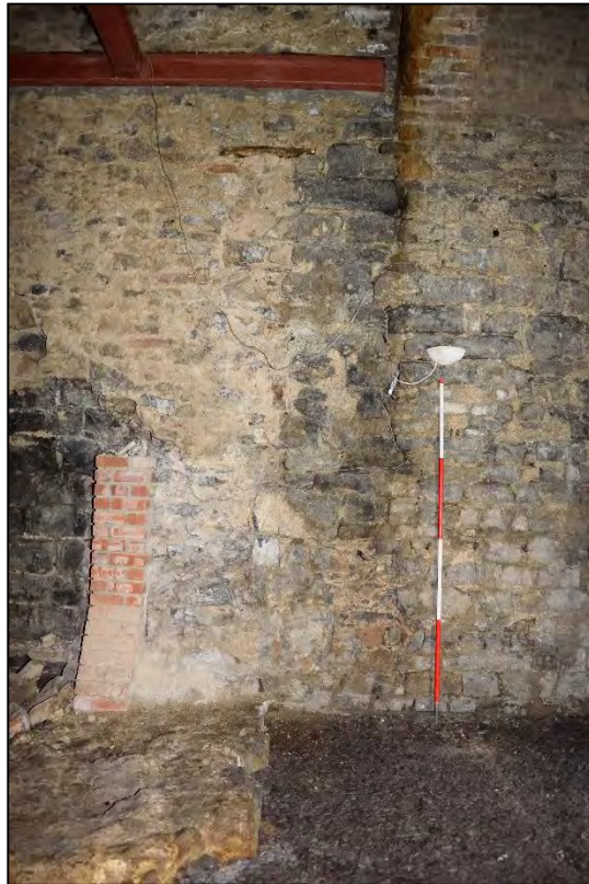
Plate 63: Change in building materials in the northern wall of the northern gatehouse
