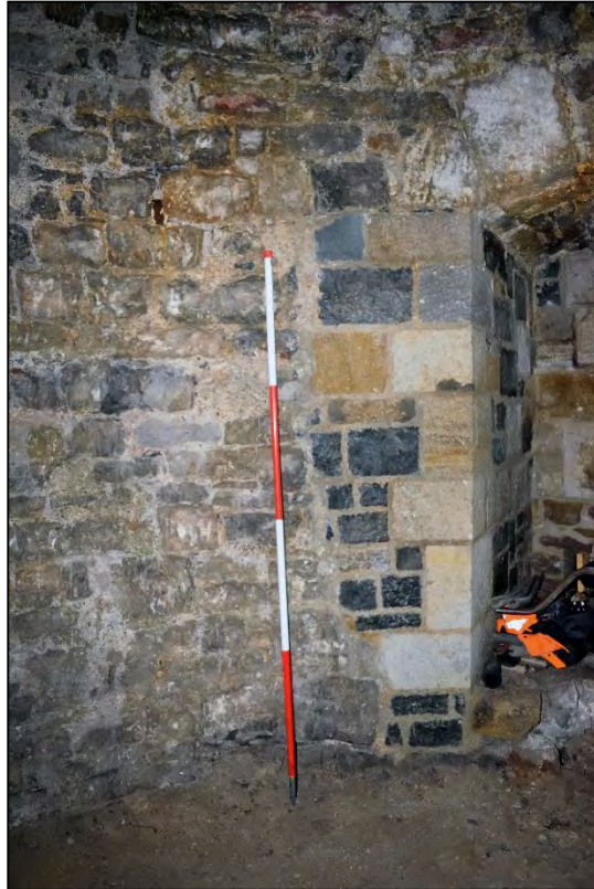
Plate 57: Modern repairs to the embrasure
