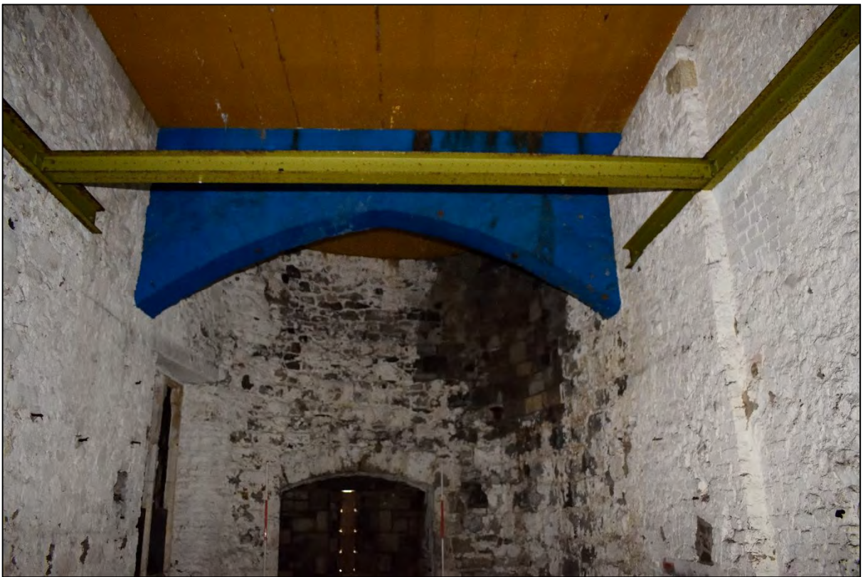
Plate 44: Arch over the southern gatehouse and modern metal supports
