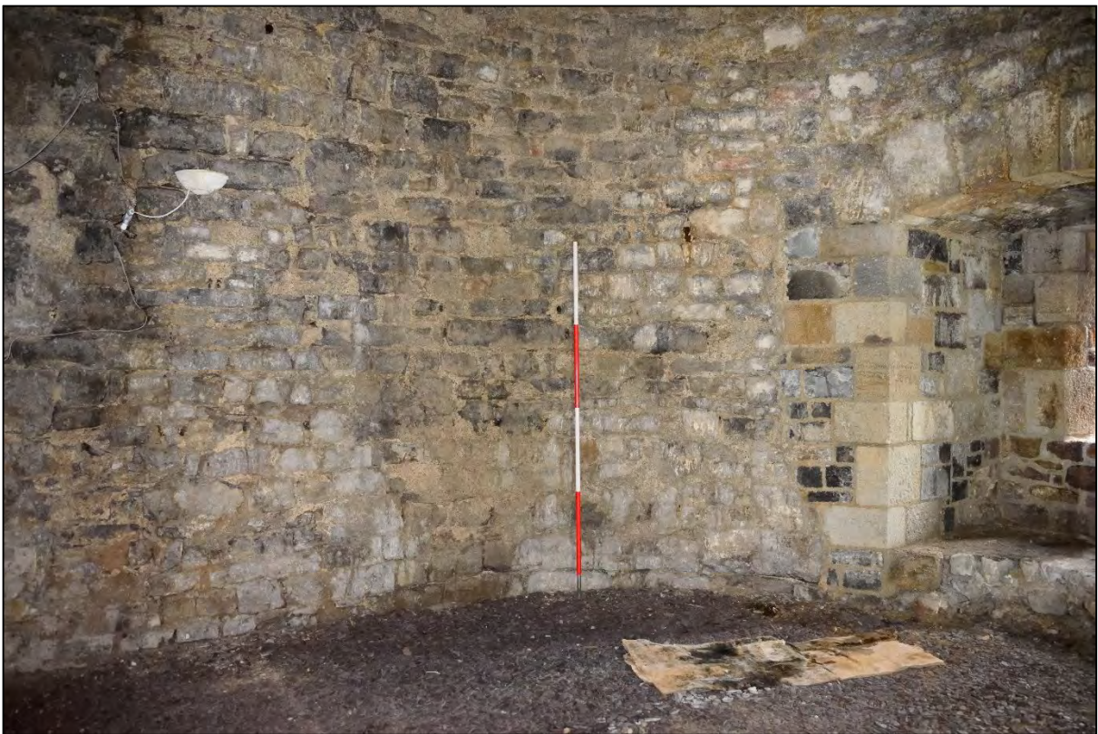
Plate 62: Course, moderate sized block at the east end of the north wall
