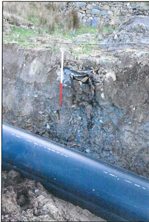
Plate 45: Slate lined drain PRN 61714
