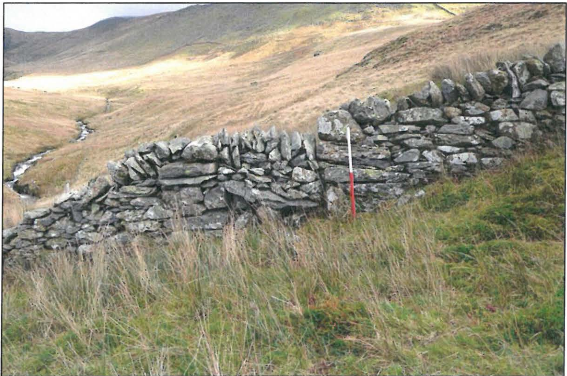
Plate 10: Blocked opening in Wall PRN 61694
