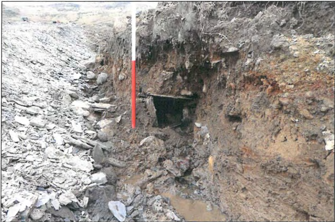
Plate 53: Slate lined drain PRN 61709
