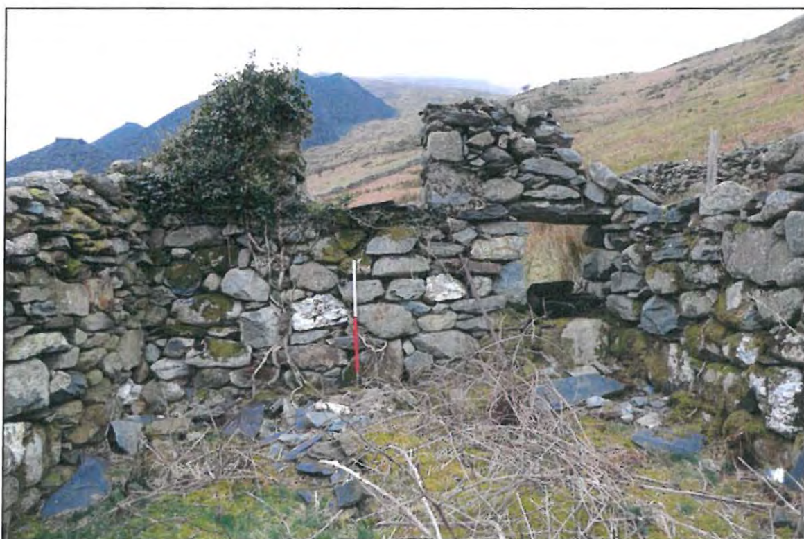
Plate 42: Inside northern gable of PRN 61705 showing both the door and pitching hole
