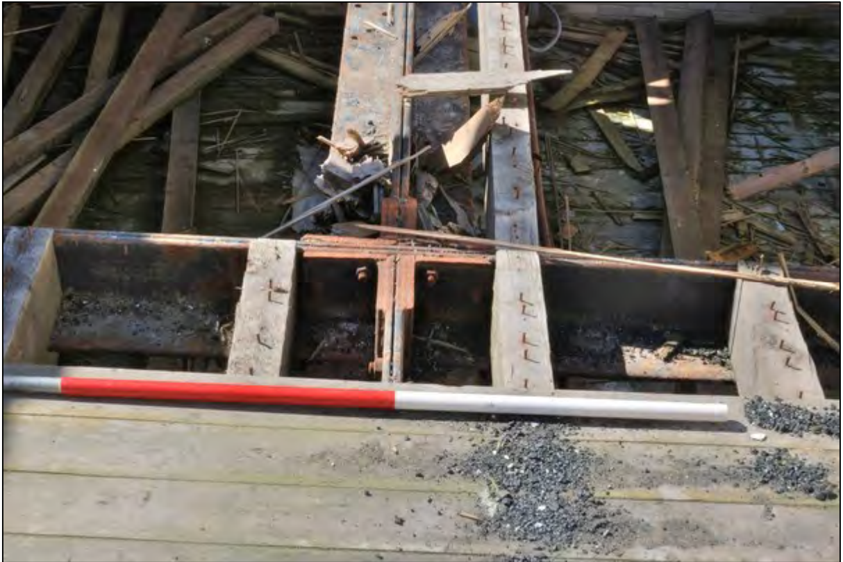
Plate 23: The upper side of the floor supports
