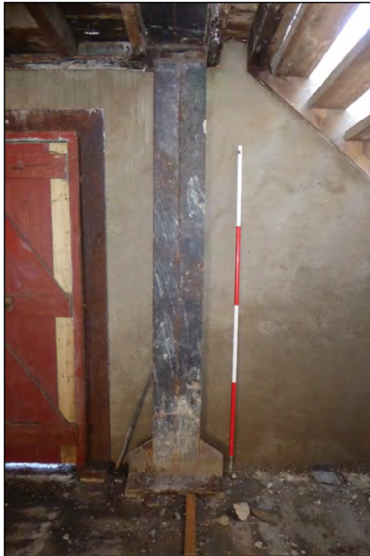
Plate 15: Steel post in the northern gable wall
