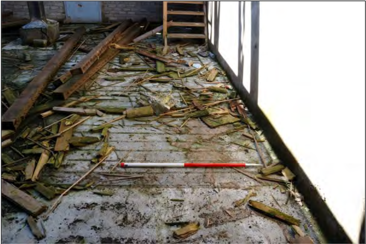
Plate 19: Differential floor finish between the two ends of the main ground floor room
