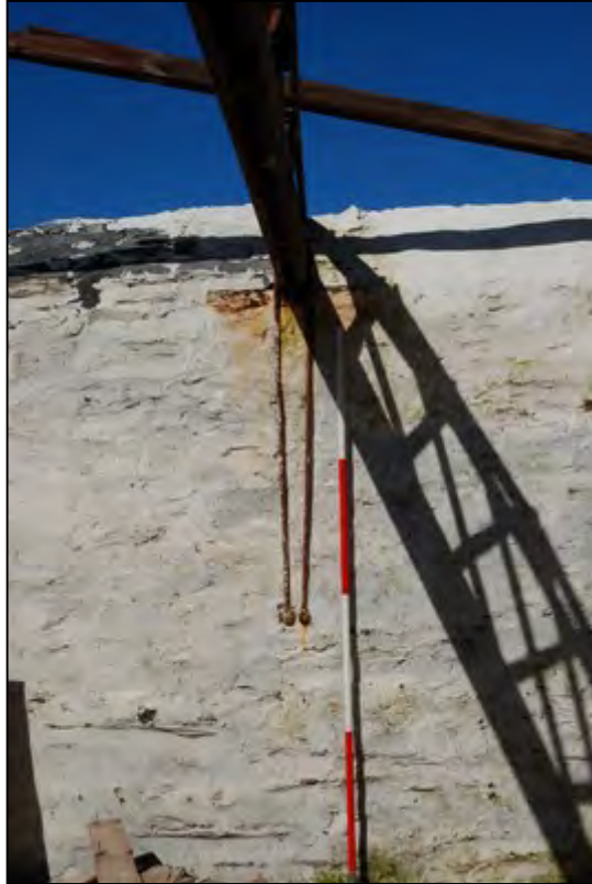
Plate 31: Iron straps holding the roof structure
