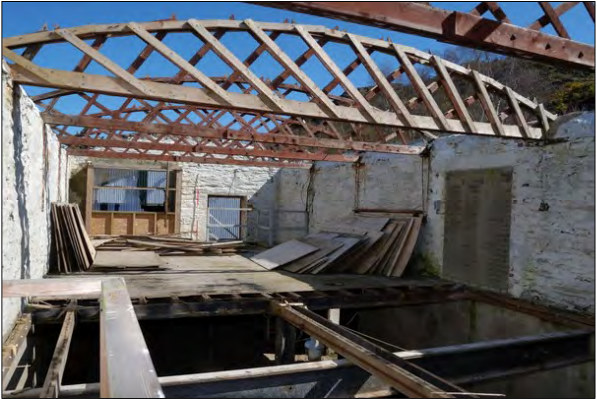
Plate 27: The “Belfast Trusses”
