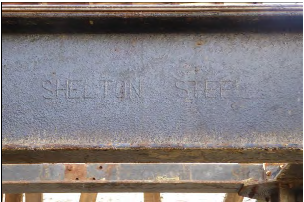
Plate 16: Manufacturer's stamp on one of the rolled steel beams.
