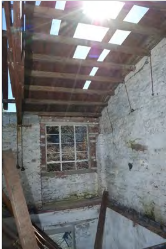
Plate 29: The surviving portion of the roof structure
