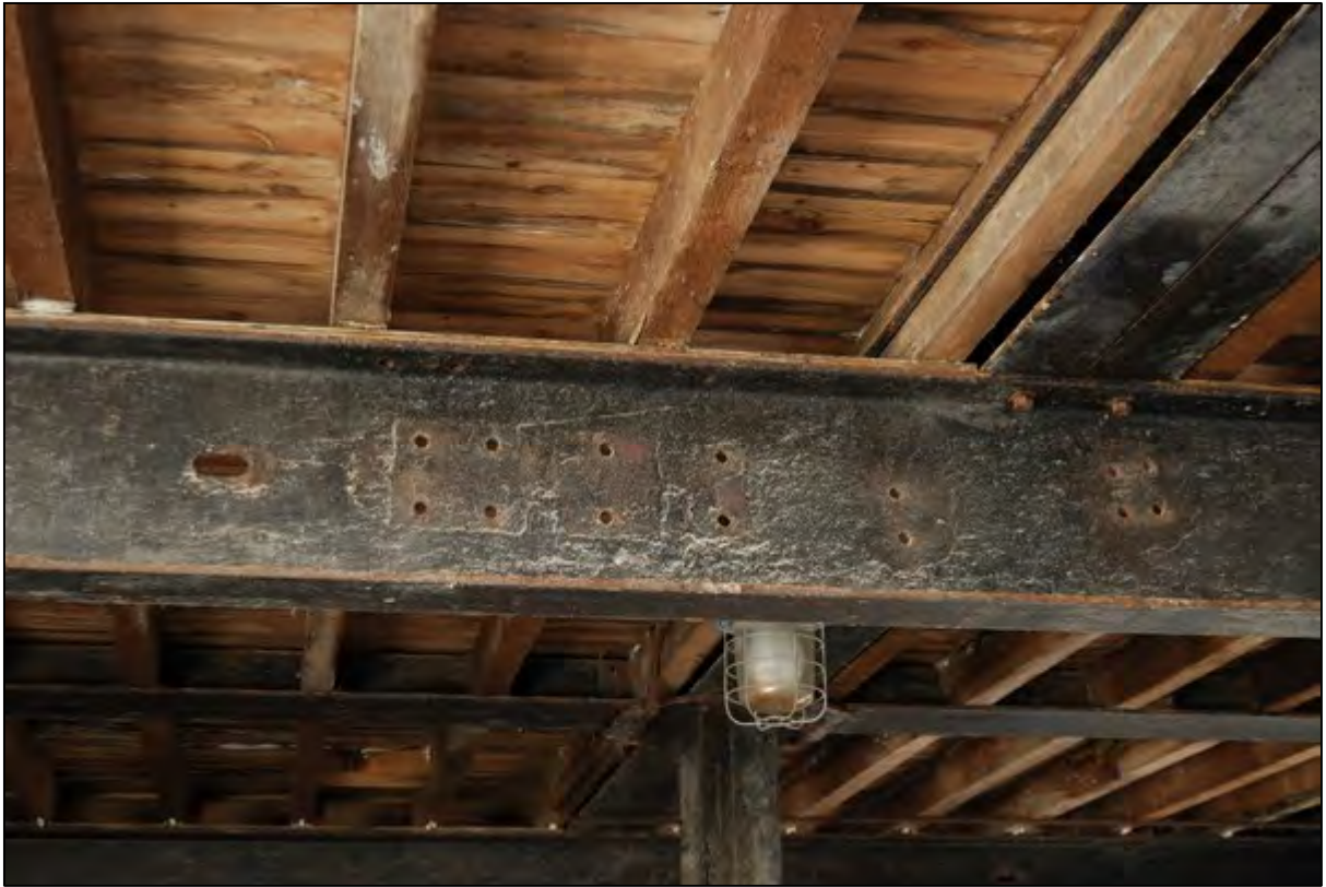
Plate 17: Evidence for possible previous use of the rolled steel beams
