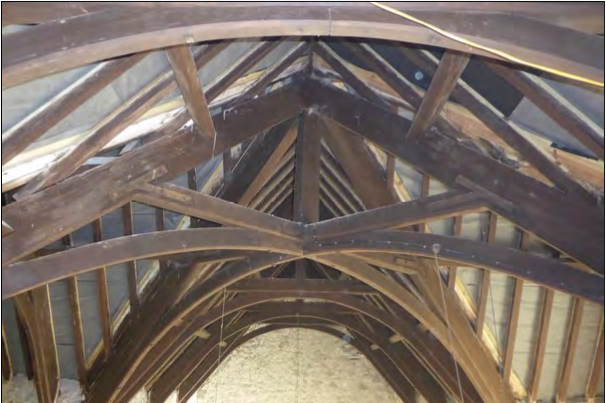
Plate 26: The roof structure over the crossing
