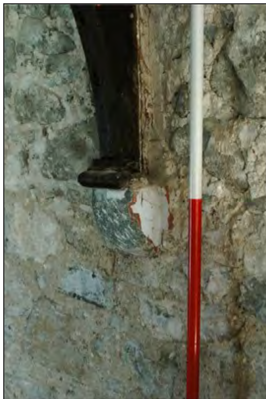
Plate 27: Corbel and base of Truss 7
