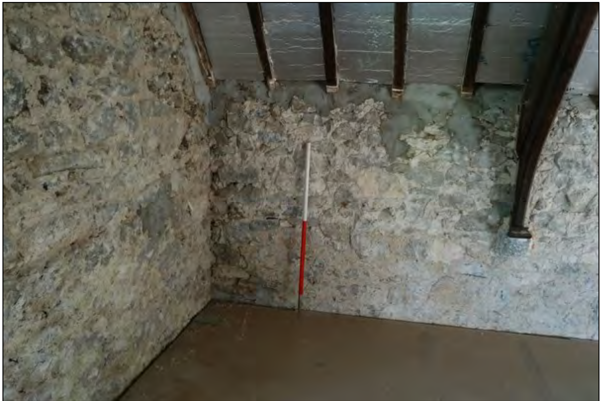
Plate 28: Break in the stonework at the level of the corbels
